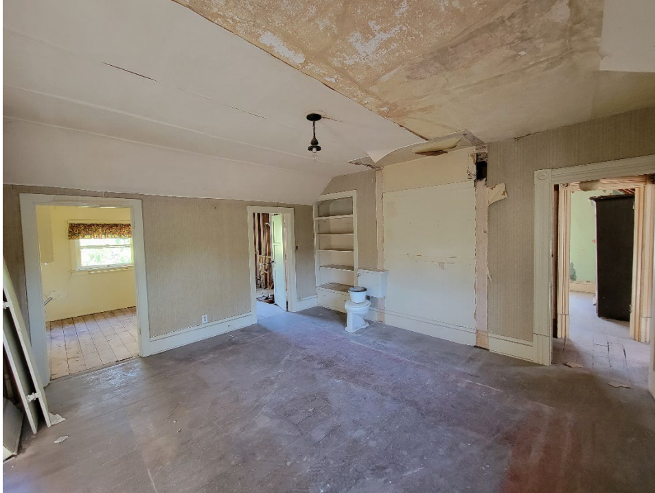
Photo 11 Second floor bedroom north side, view to southeast
