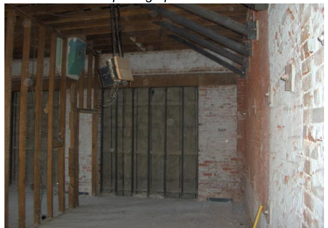
Figure 2: Unfinished second floor interior.
