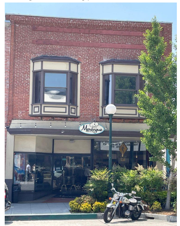
Figure 4: Current building, post-2008 remodel.
