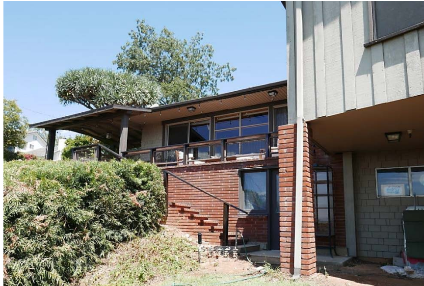
Figure 4. Tertiary (Southern) Façade, 126 Sky Way SOURCE: Sapphos Environmental, Inc., 2017
