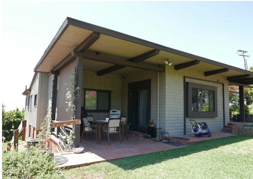
Figure 2. Primary (Northern) Façade Porch, 126 Sky Way SOURCE: Sapphos Environmental, Inc., 2017
