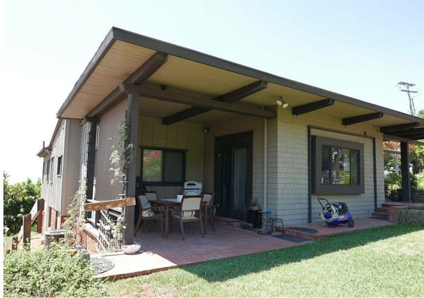
Figure 7. Primary (Northern) Façade Porch, 126 Sky Way SOURCE: Sapphos Environmental, Inc., 2017
