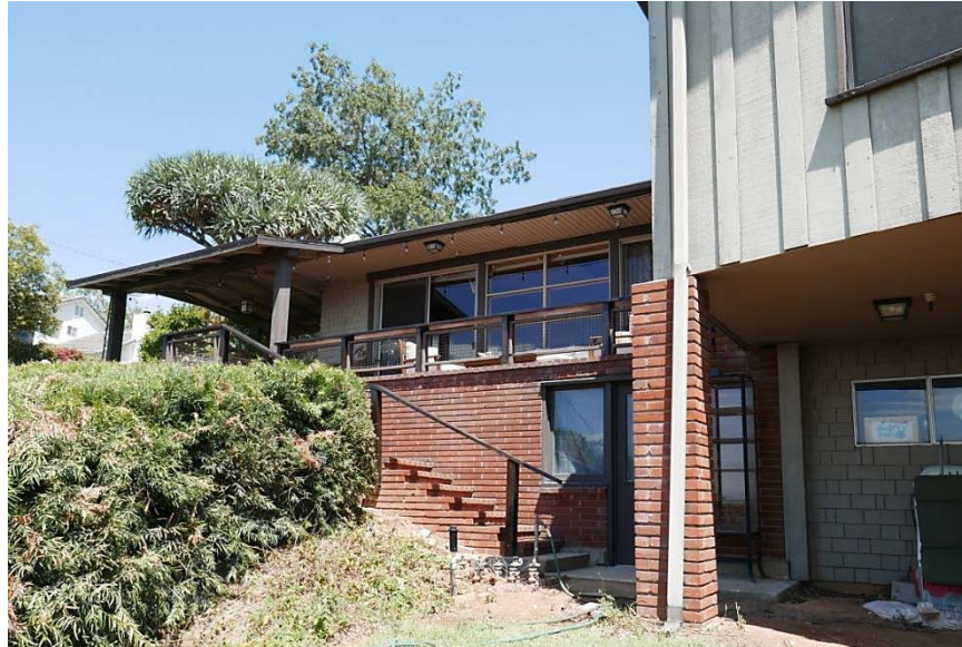
Figure 9. Tertiary (Southern) Façade, 126 Sky Way SOURCE: Sapphos Environmental, Inc., 2017
