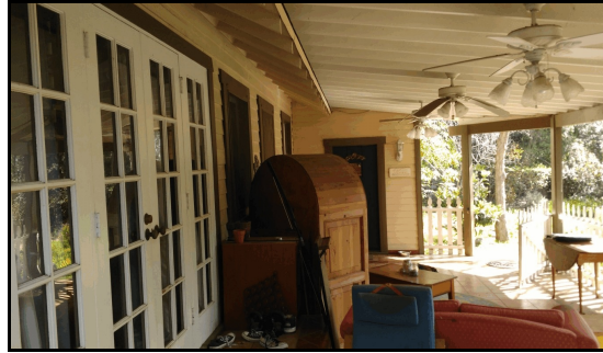
French Doors Installed - 1980
