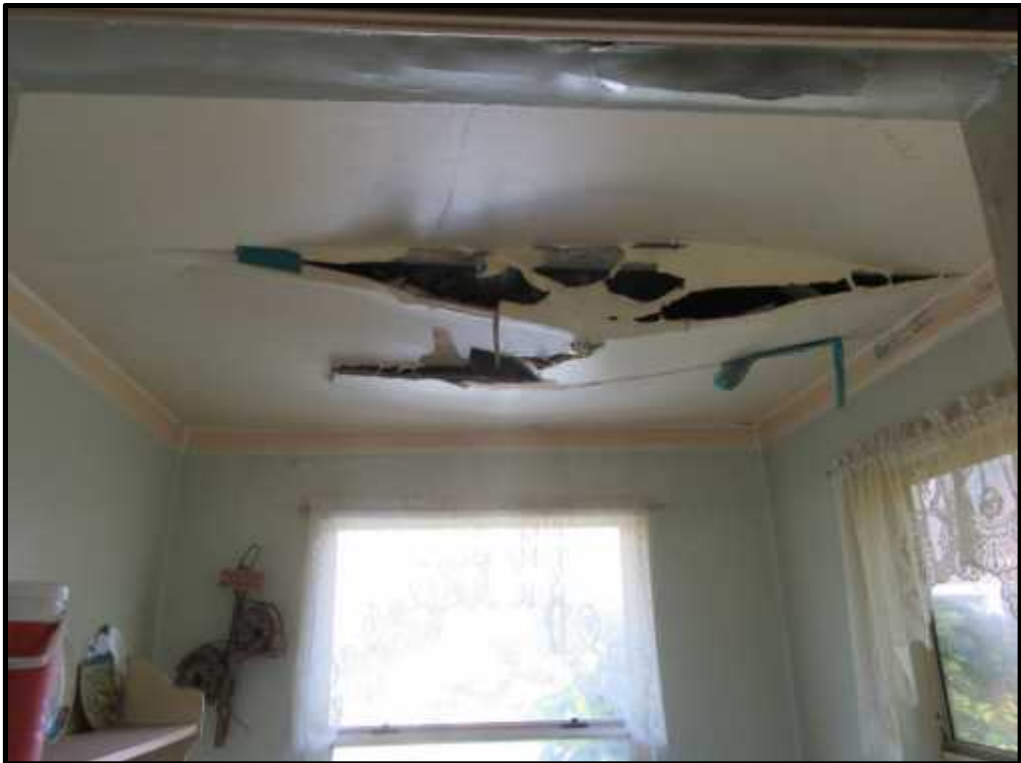
PHOTO OF INTERIOR
