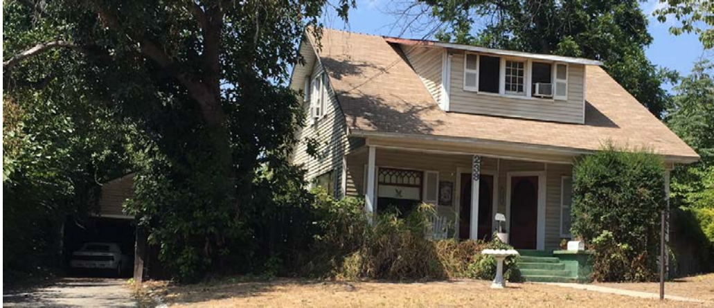
Garage and residence southern elevation, view to the northwest (8/23/17).
