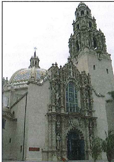
The 1915 Panama-California Exposition buildings in Balboa Park became San Diego's first designated historic site and district. (Photo courtesy City of San Diego)
