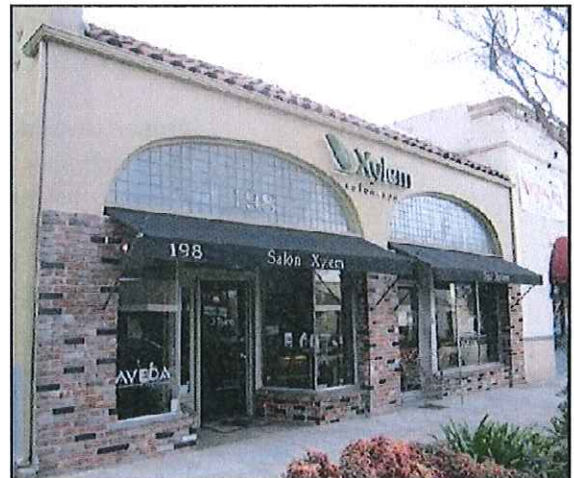
The owners of this commercial property restored the building's original transoms and later removed the non-contributing brick façade, thanks in part to supportive ordinances and other incentives of Monrovia's preservation program.
