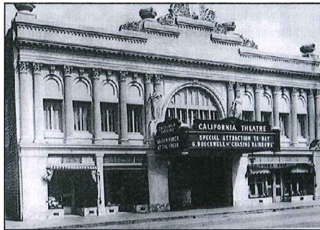
California Theatre, ca 1920s. (All photos courtesy City of Pittsburg)
