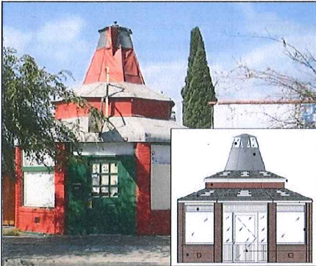
The Koffee Pot rehabilitation project is one example of the city's collaboration with property owners to preserve Long Beach's historic resources and ensure the sustainability of local businesses. (Photo courtesy City of Long Beach)
