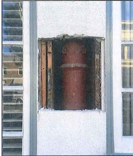
Ainsworth Block, one of the oldest buildings in Orange, is being restored by its present-day owner, with careful attention to historic accuracy. The building's original cast iron columns will be incorporated into the restored
