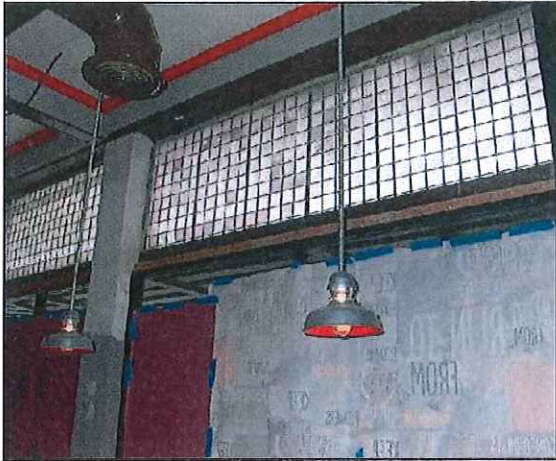
Original leaded-glass transoms were rediscovered and preserved during the Blaze Pizza rehabilitation project.
