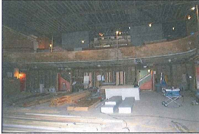
Main auditorium during restoration. Among the challenges was removing a destructive colony of bats.
