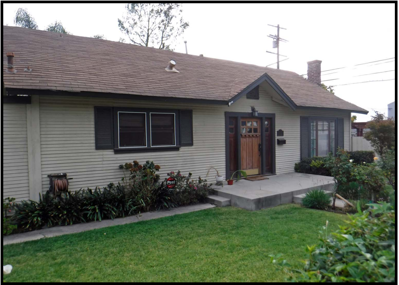
Overview of North Elevation, 448 Linwood Avenue, Monrovia (SE)
