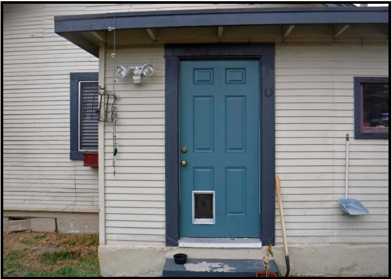
Replaced Rear Door, East Elevation, 448 Linwood Avenue, Monrovia (W)
