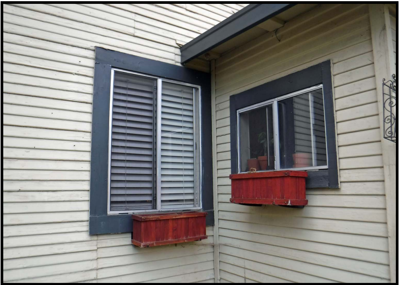
Replaced Windows on East Elevation, 448 Linwood Avenue, Monrovia (NW)
