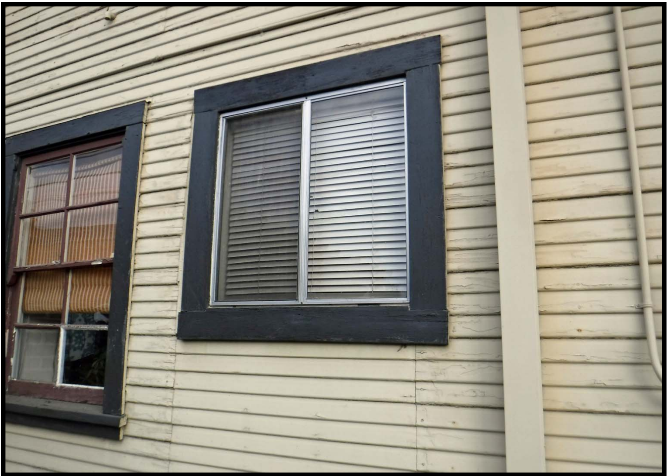
Window Detail, West Elevation, 448 Linwood Avenue, Monrovia (NE)
