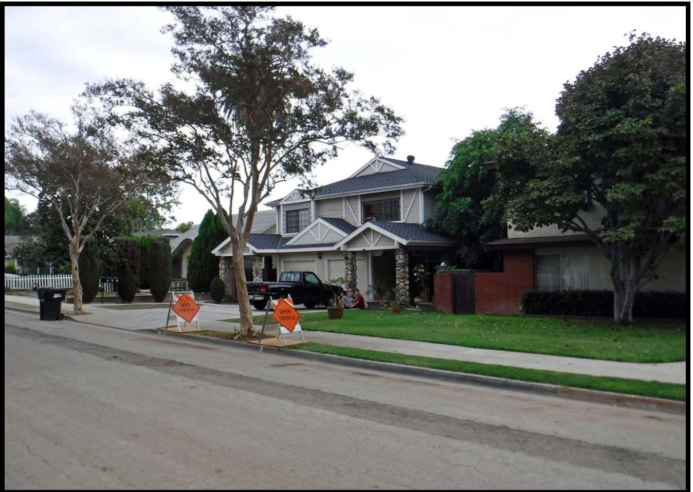
MRF Complex at 430 Linwood Avenue, Monrovia (recently replacing at 1924 residence; SE)
