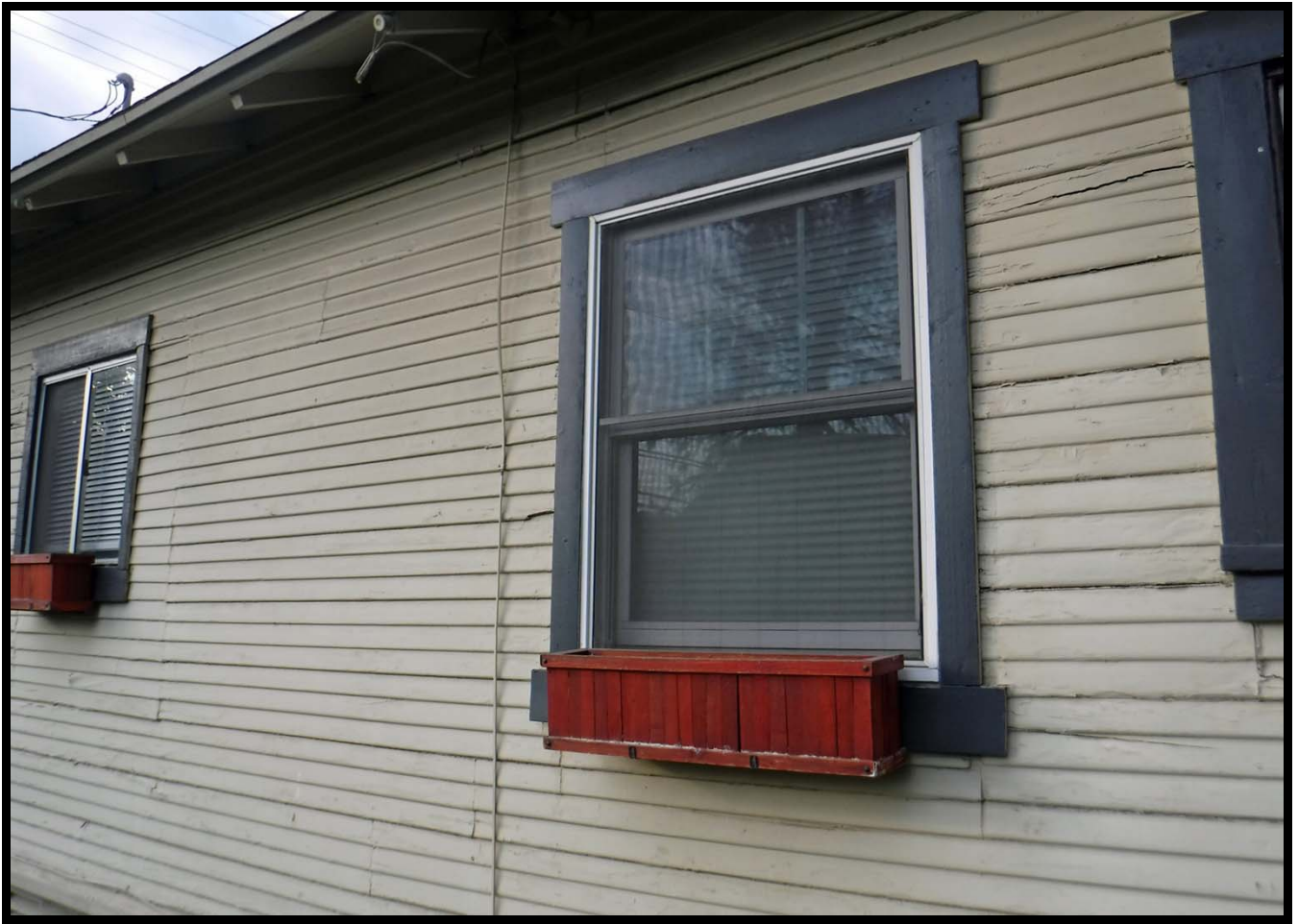
Replaced Window on South Elevation, 448 Linwood Avenue, Monrovia (NW)
