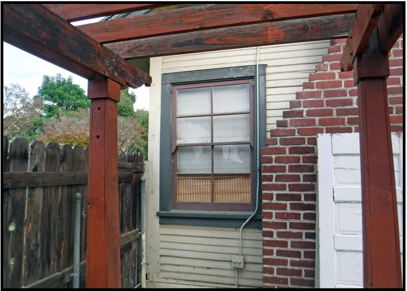
Original Window on West Elevation, 448 Linwood Avenue, Monrovia (ENE)
