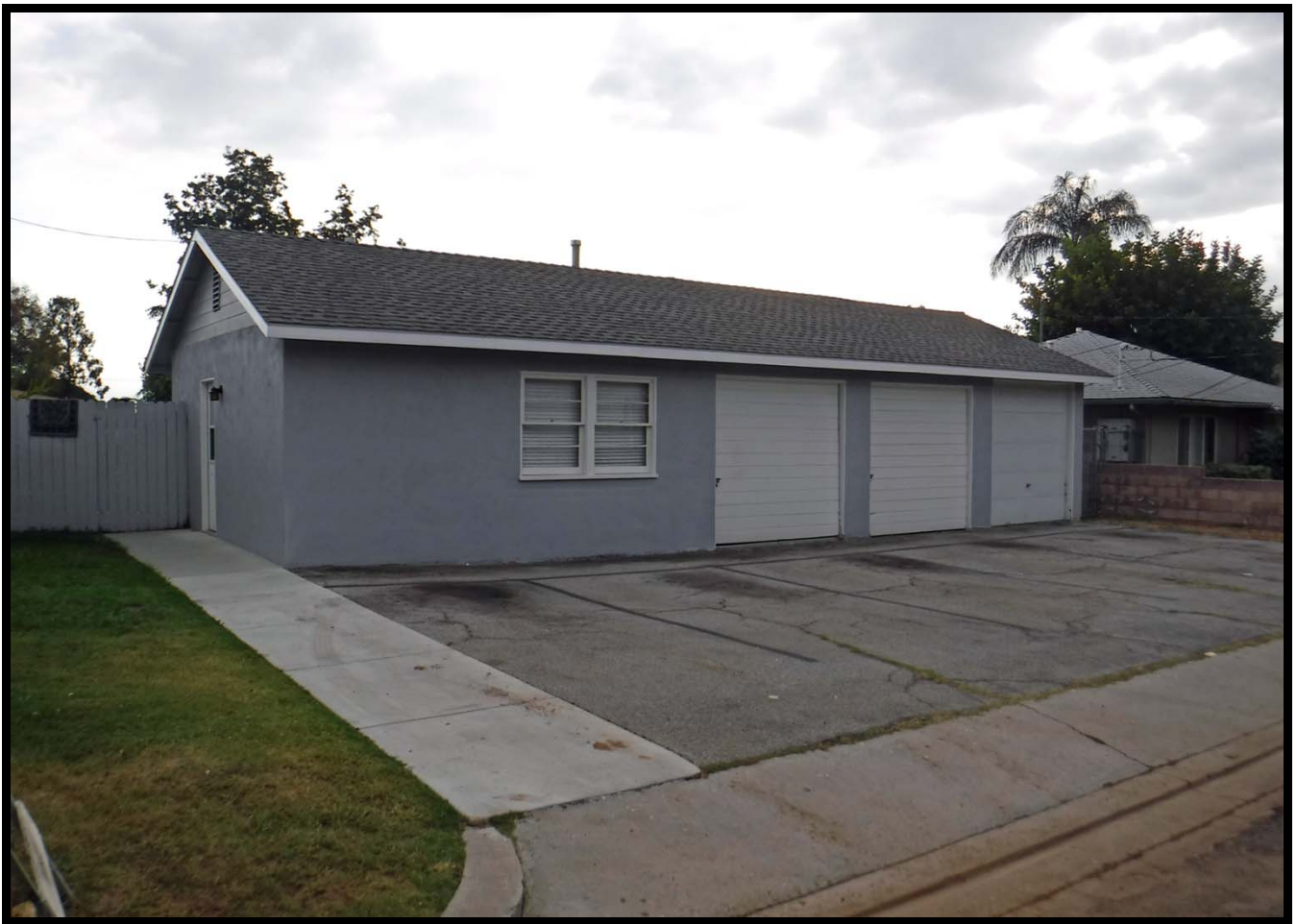
Garage Complex at 502 Linwood Avenue, Monrovia (1952; W)
