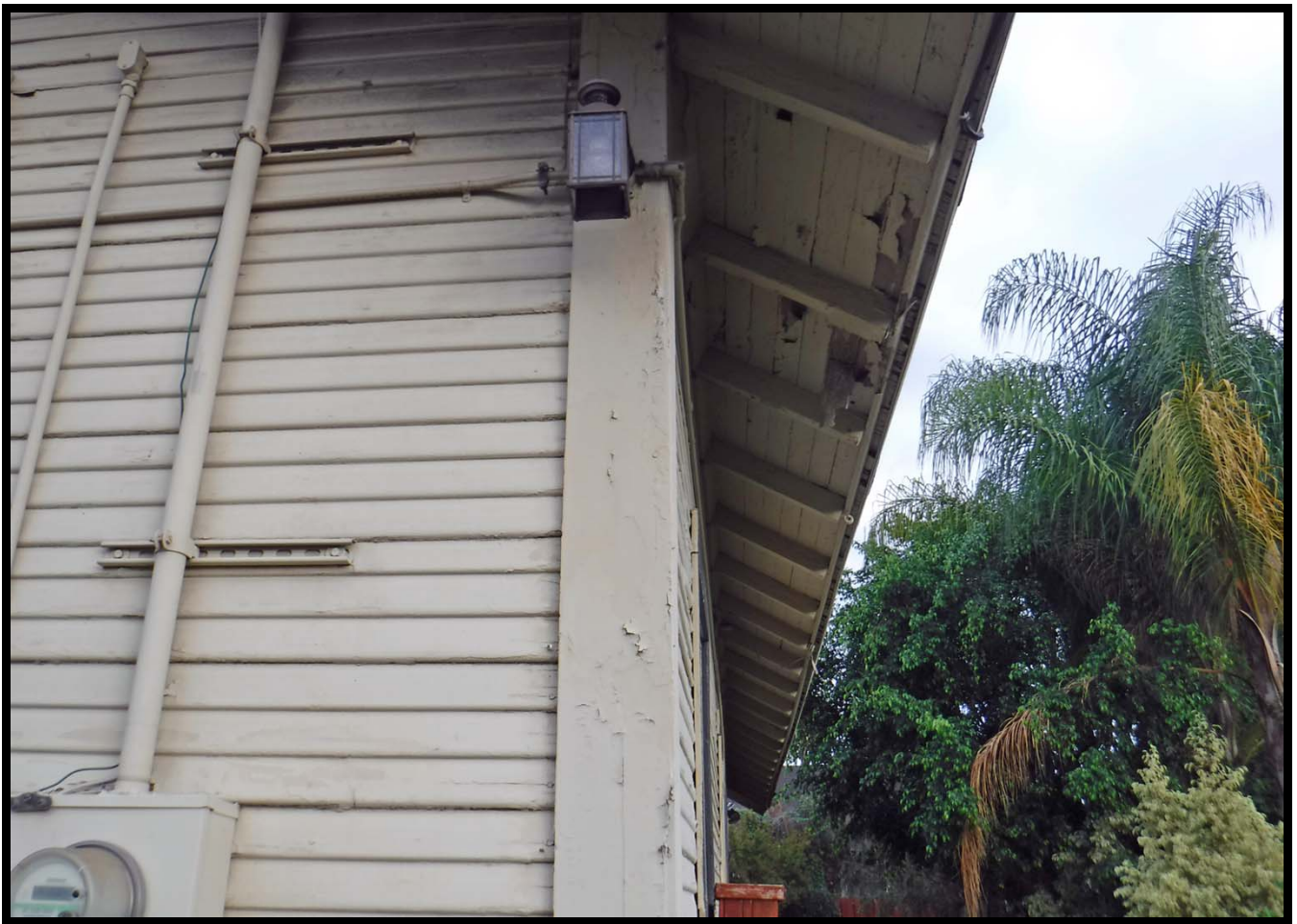
Eave on South Elevation 448 Linwood Avenue, Monrovia (E)
