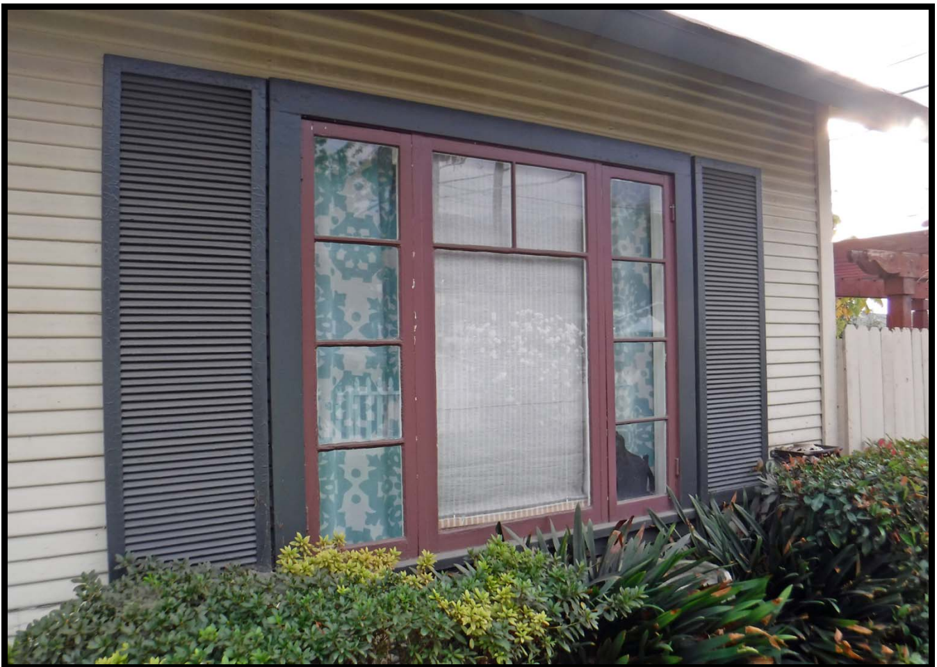
Window Detail on North Elevation of 448 Linwood Avenue, Monrovia (SE)
