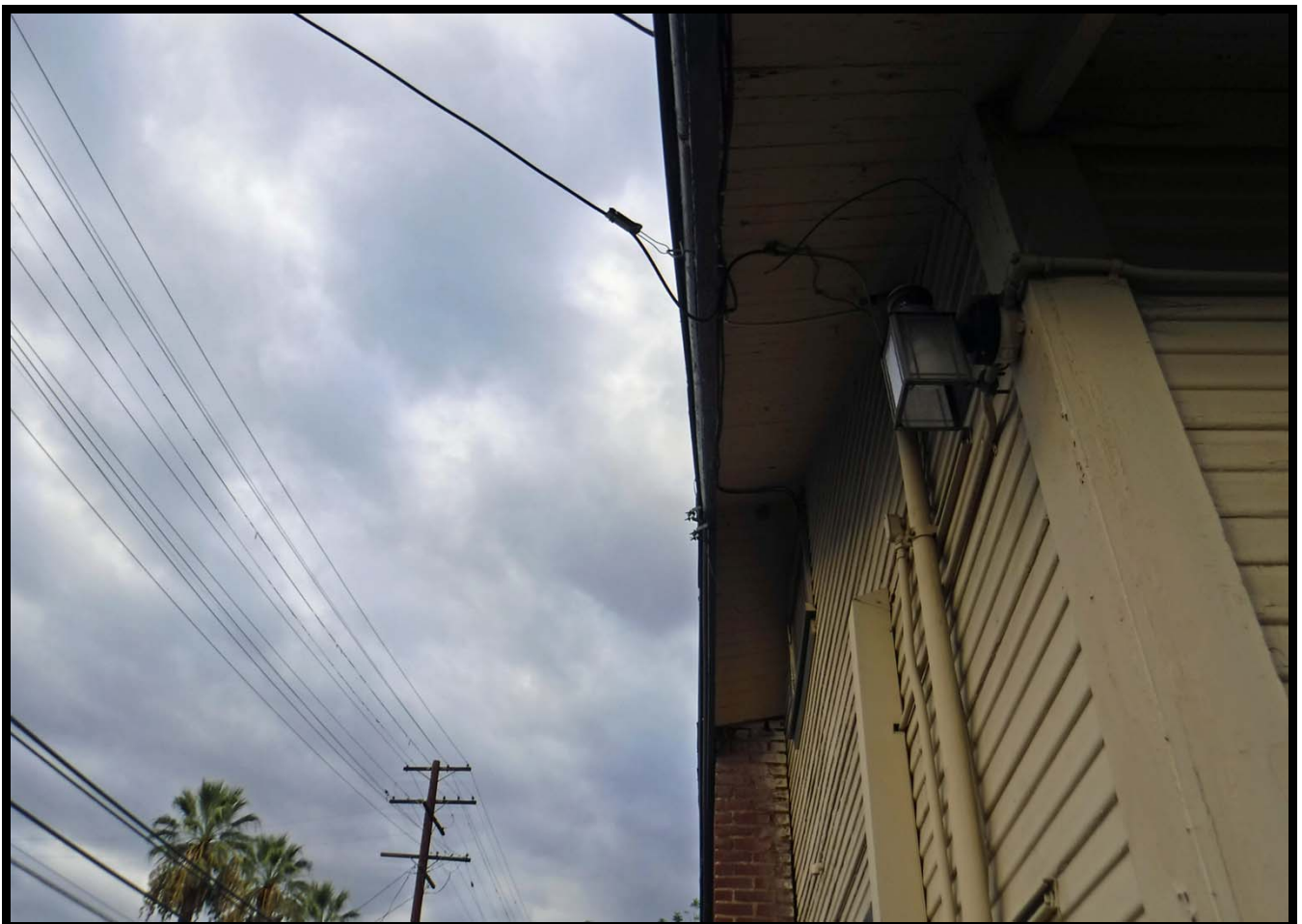
Eave on West Elevation, 448 Linwood Avenue, Monrovia (N)
