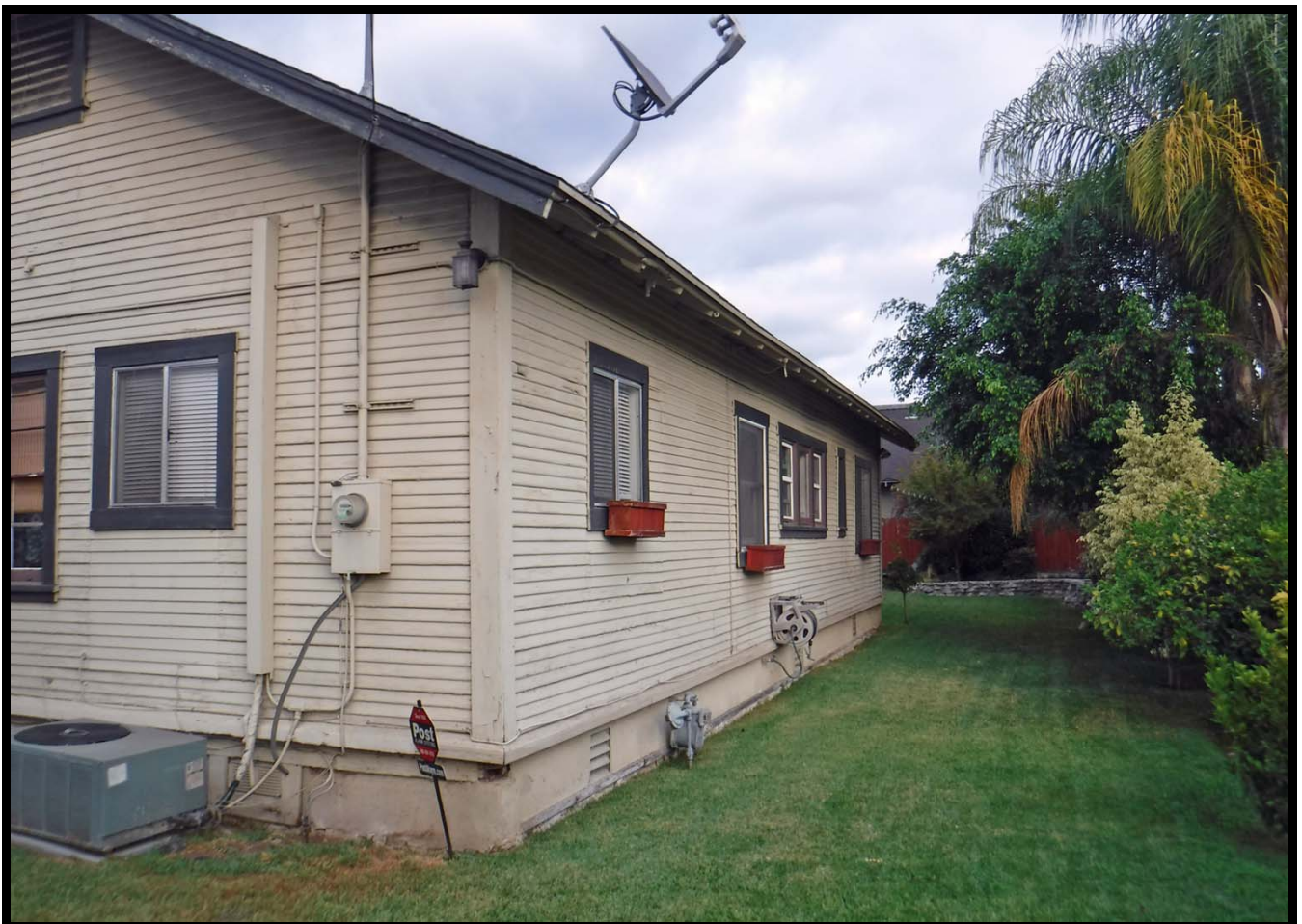
Overview of South Elevation, 448 Linwood Avenue, Monrovia (ENE)
