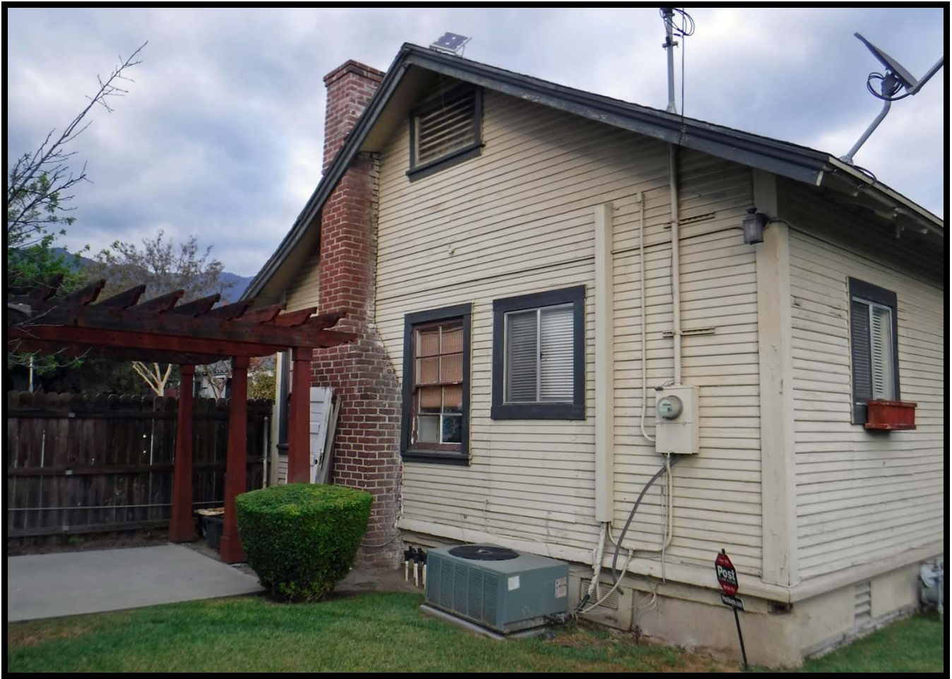
Overview of West Elevation, 448 Linwood Avenue, Monrovia (NE)
