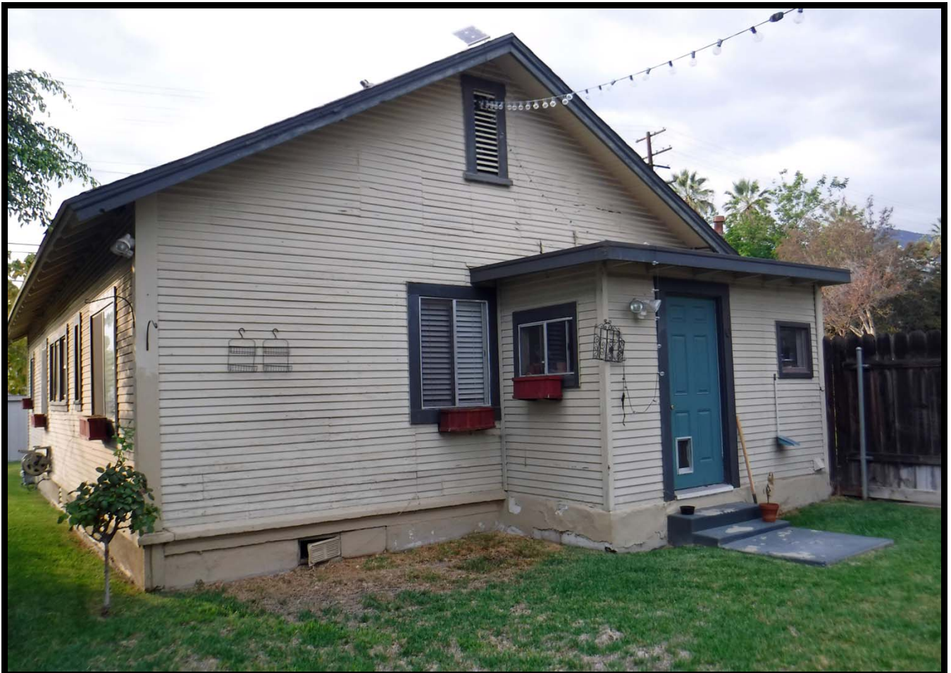
Overview of East Elevation, 448 Linwood Avenue, Monrovia (NW)
