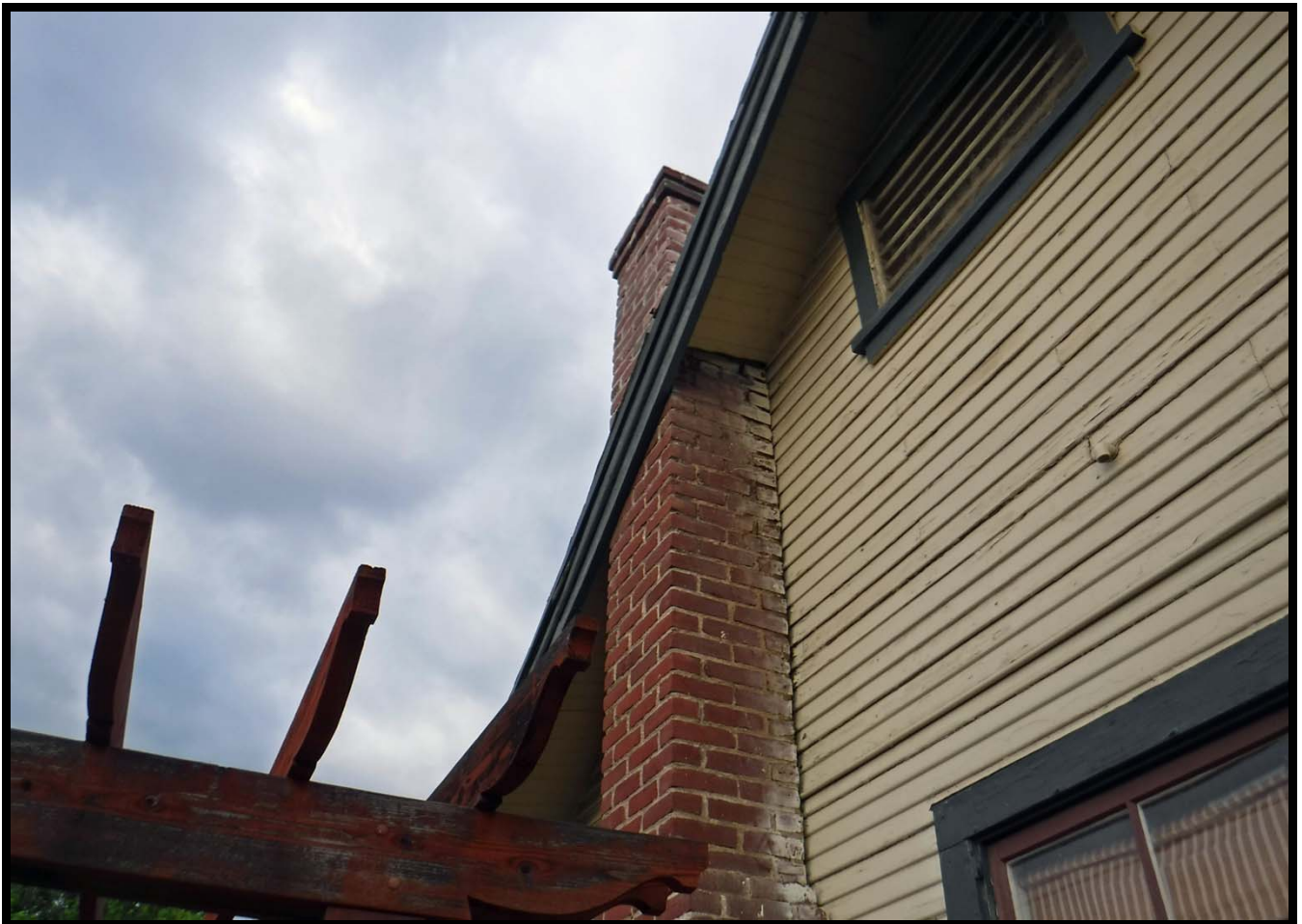
Red Brick Chimney on West Elevation, 448 Linwood Avenue, Monrovia (NE)
