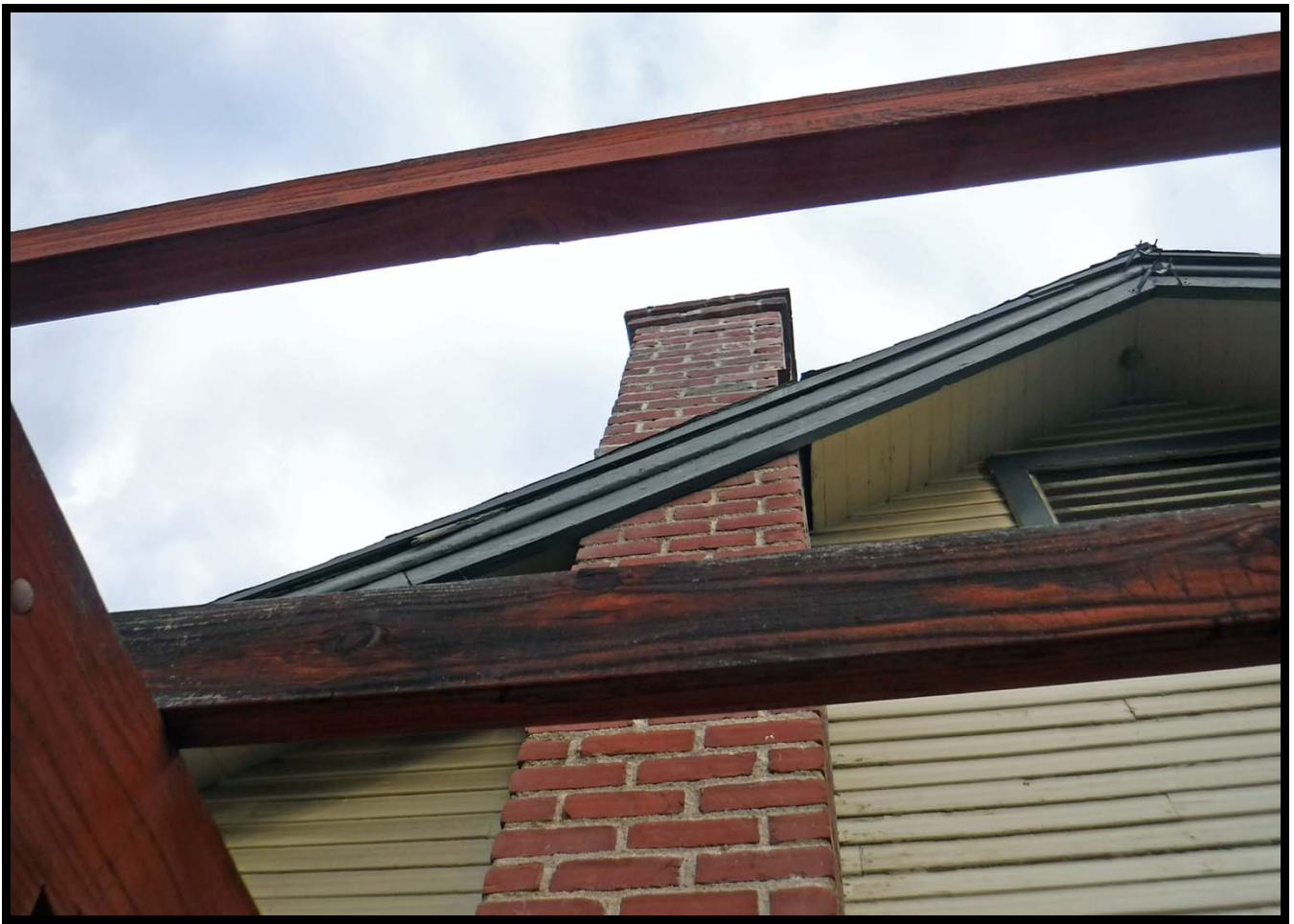
Chimney on West Elevation, 448 Linwood Avenue, Monrovia (E)
