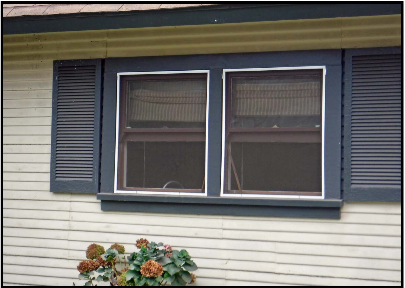
North Elevation and Original Windows, 448 Linwood Avenue, Monrovia (SSE)
