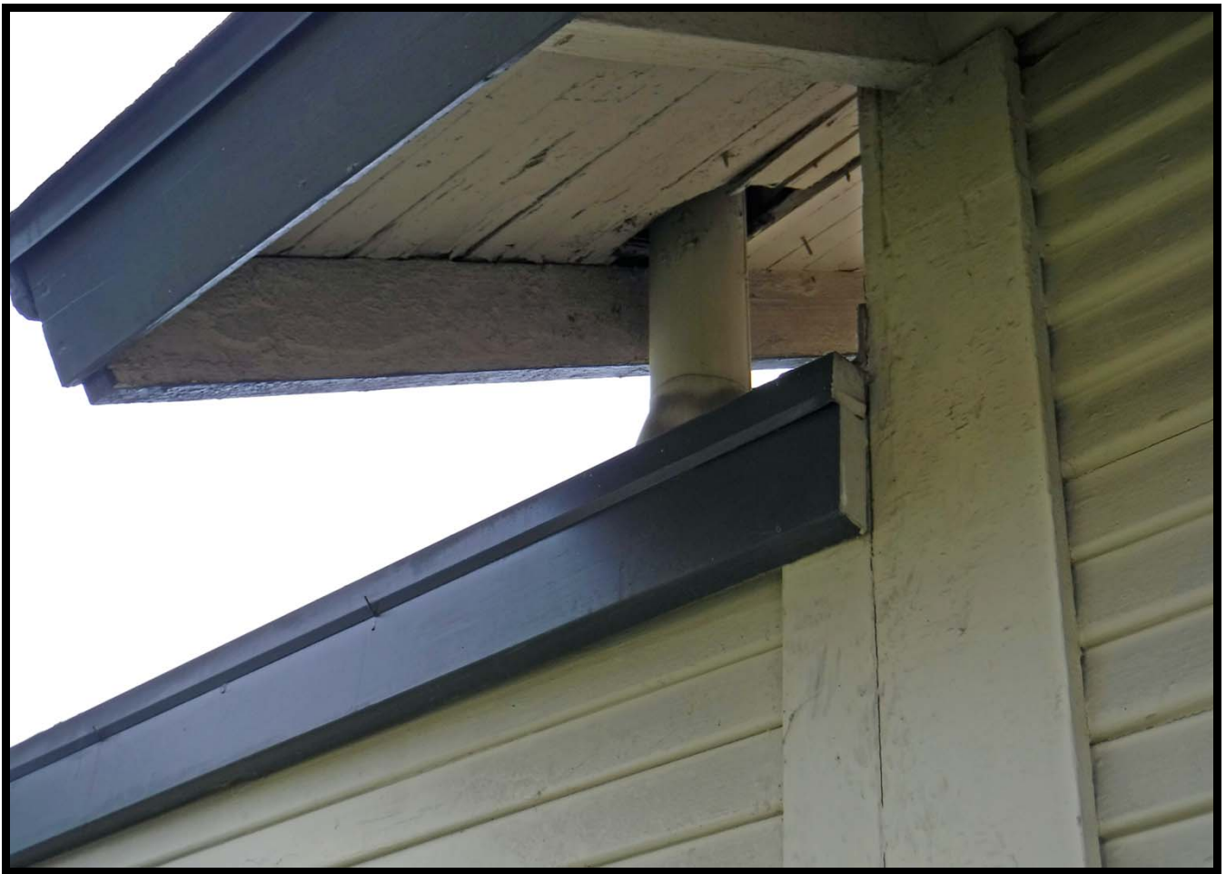
Roof Lines on North Elevation, 448 Linwood Avenue, Monrovia (SSE)
