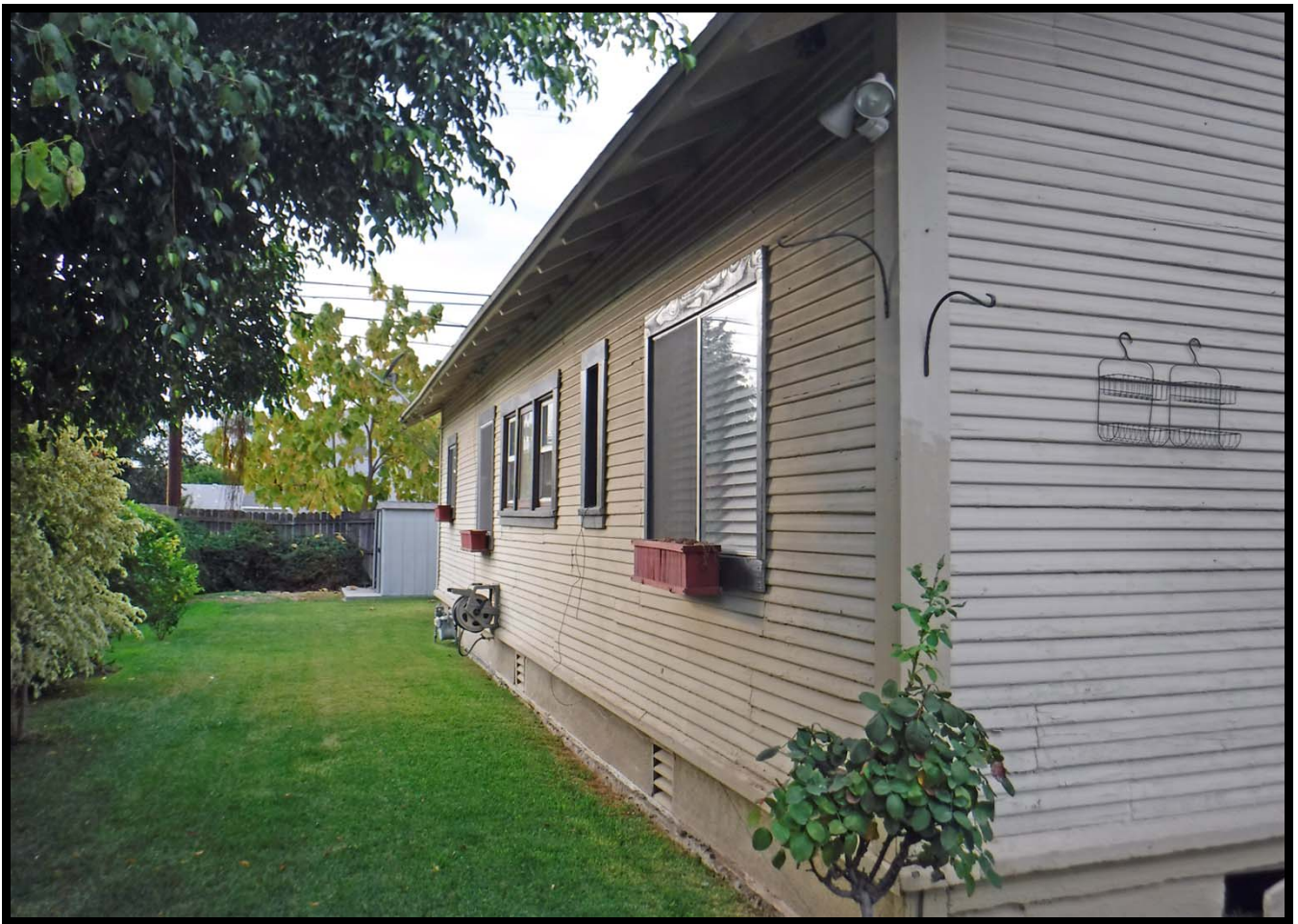
Overview of South Elevation, 448 Linwood Avenue, Monrovia (WNW)
