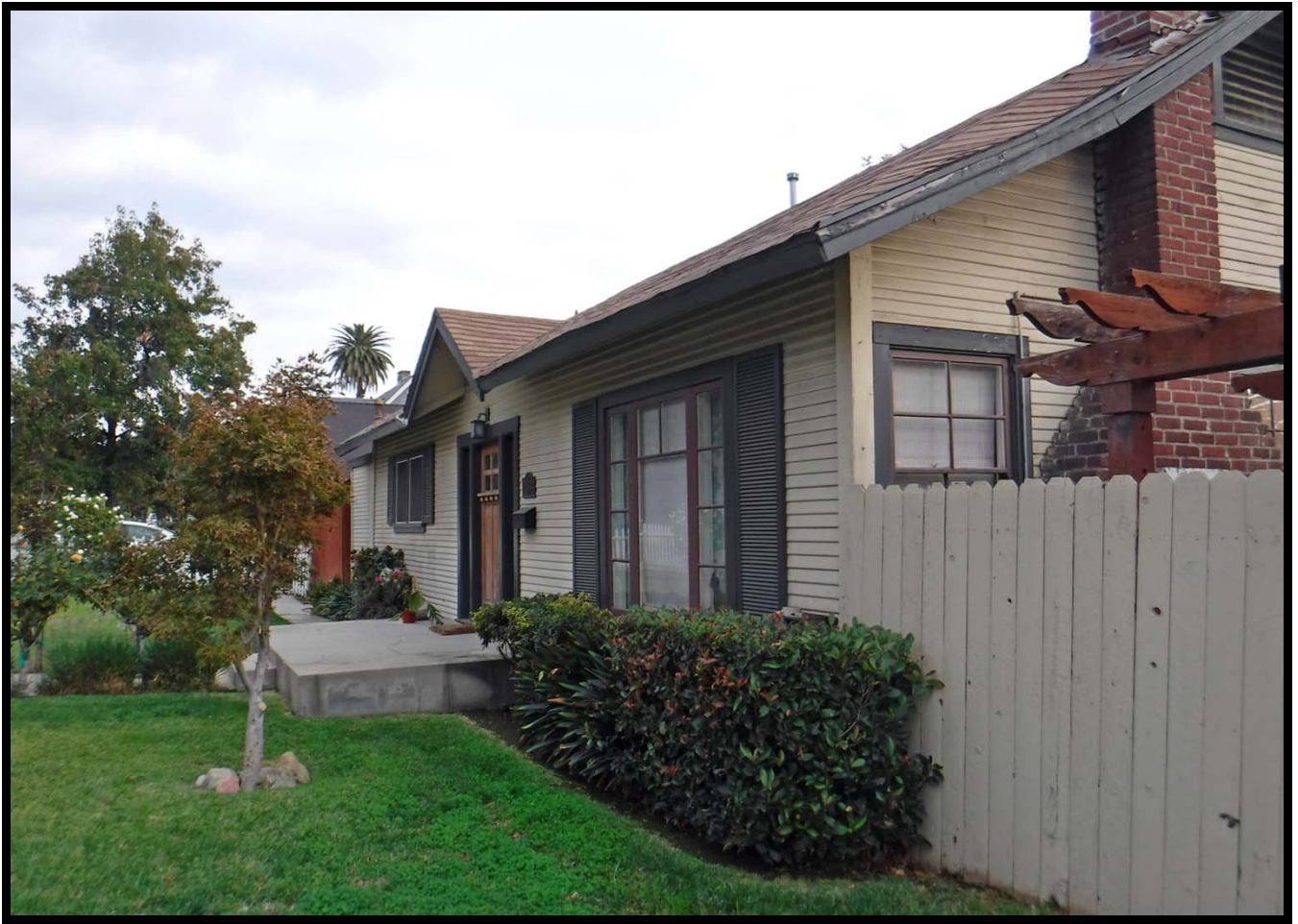
North Elevation of 448 Linwood Avenue, Monrovia (ESE)
