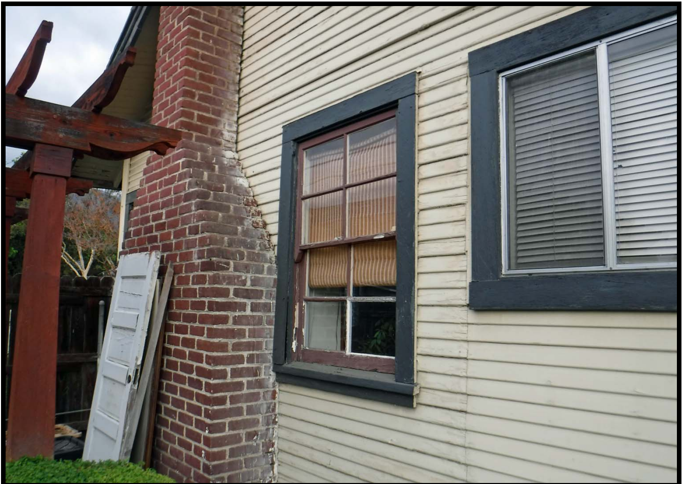
Original and Replaced Window on West Elevation, 448 Linwood Avenue, Monrovia (NE)
