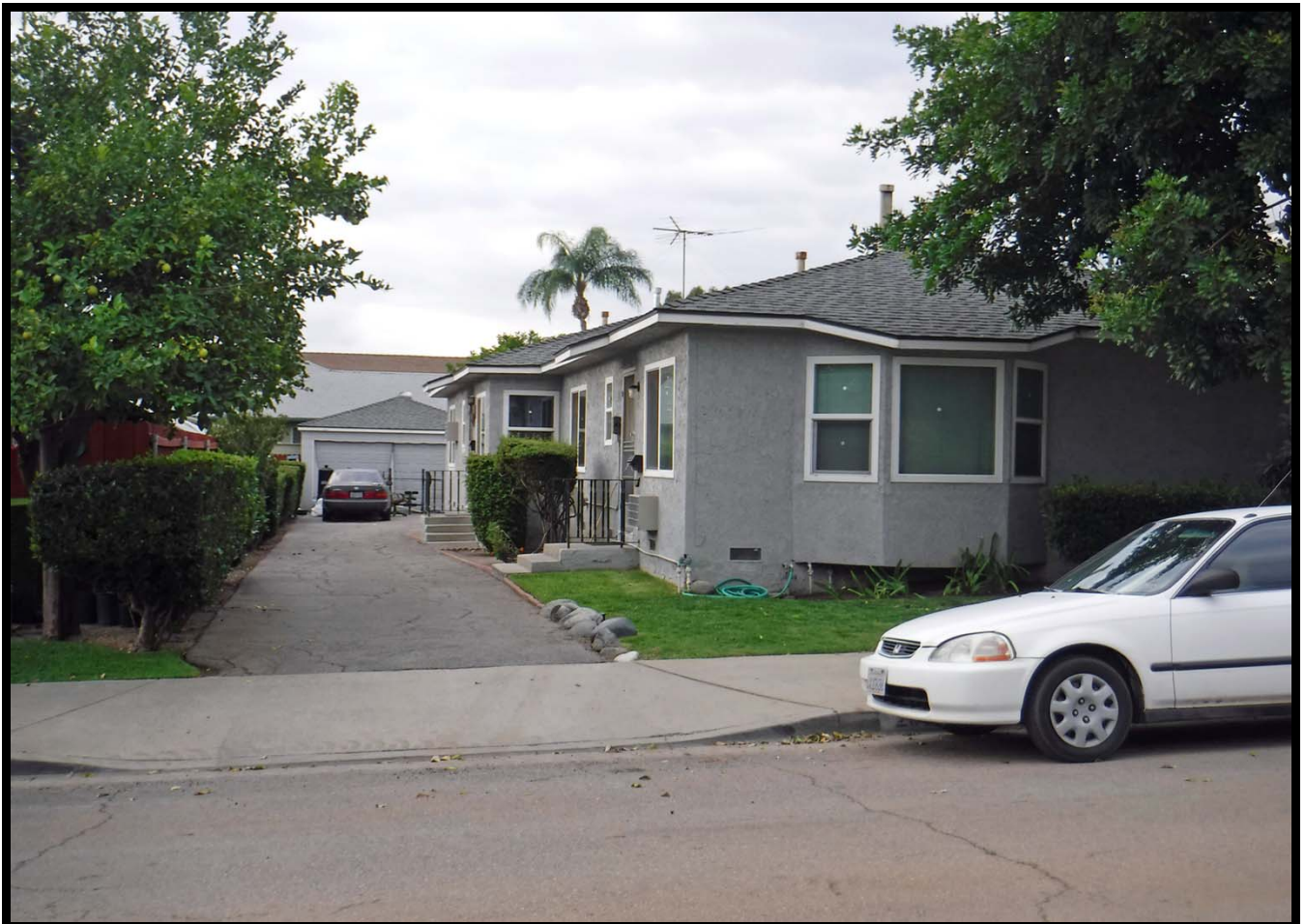
MFR Complex at 205 Mayflkower Avenue, Monrovia (1952; W)
