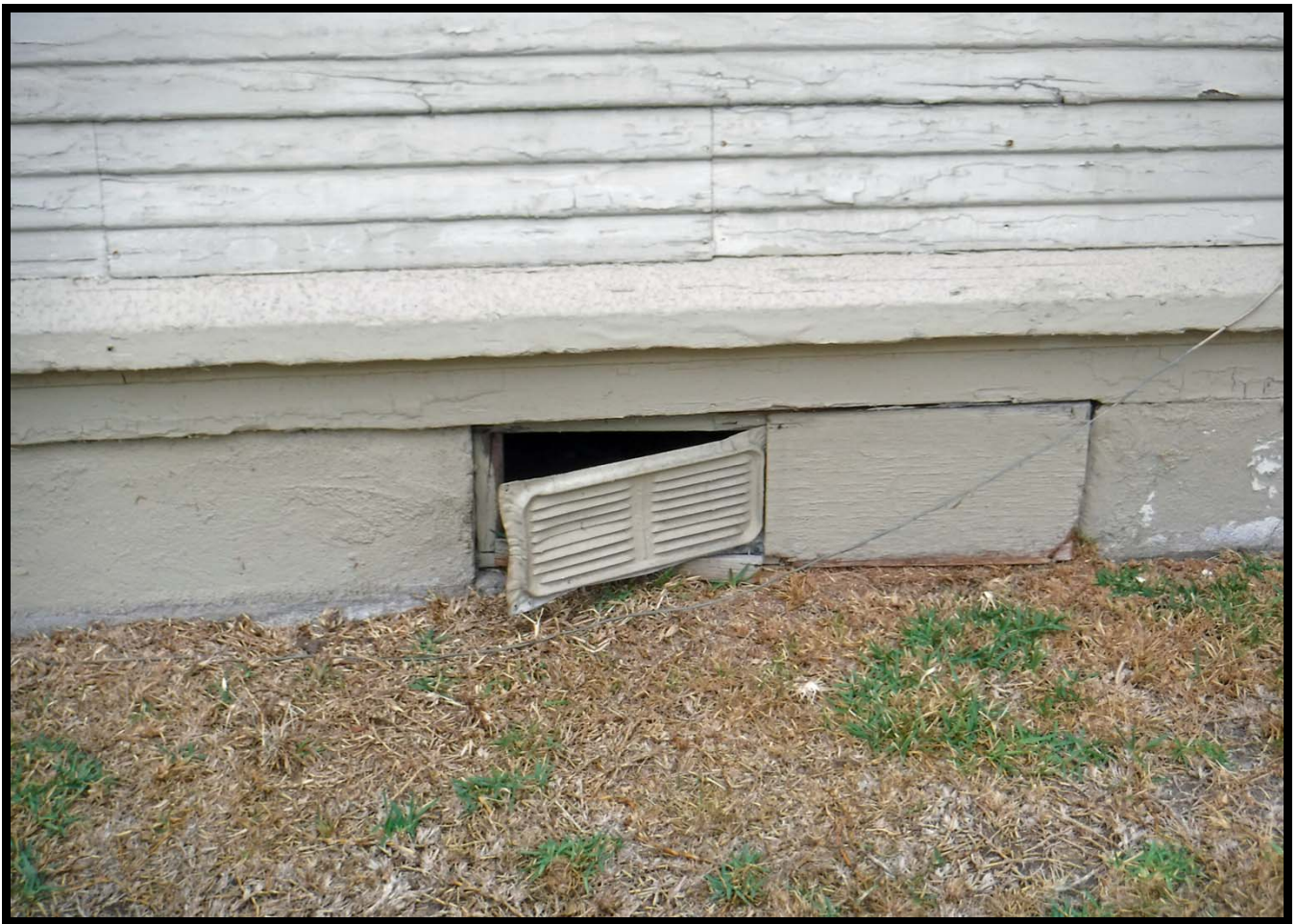
Floor Vent on East Elevation, 448 Linwood Avenue, Monrovia (W)
