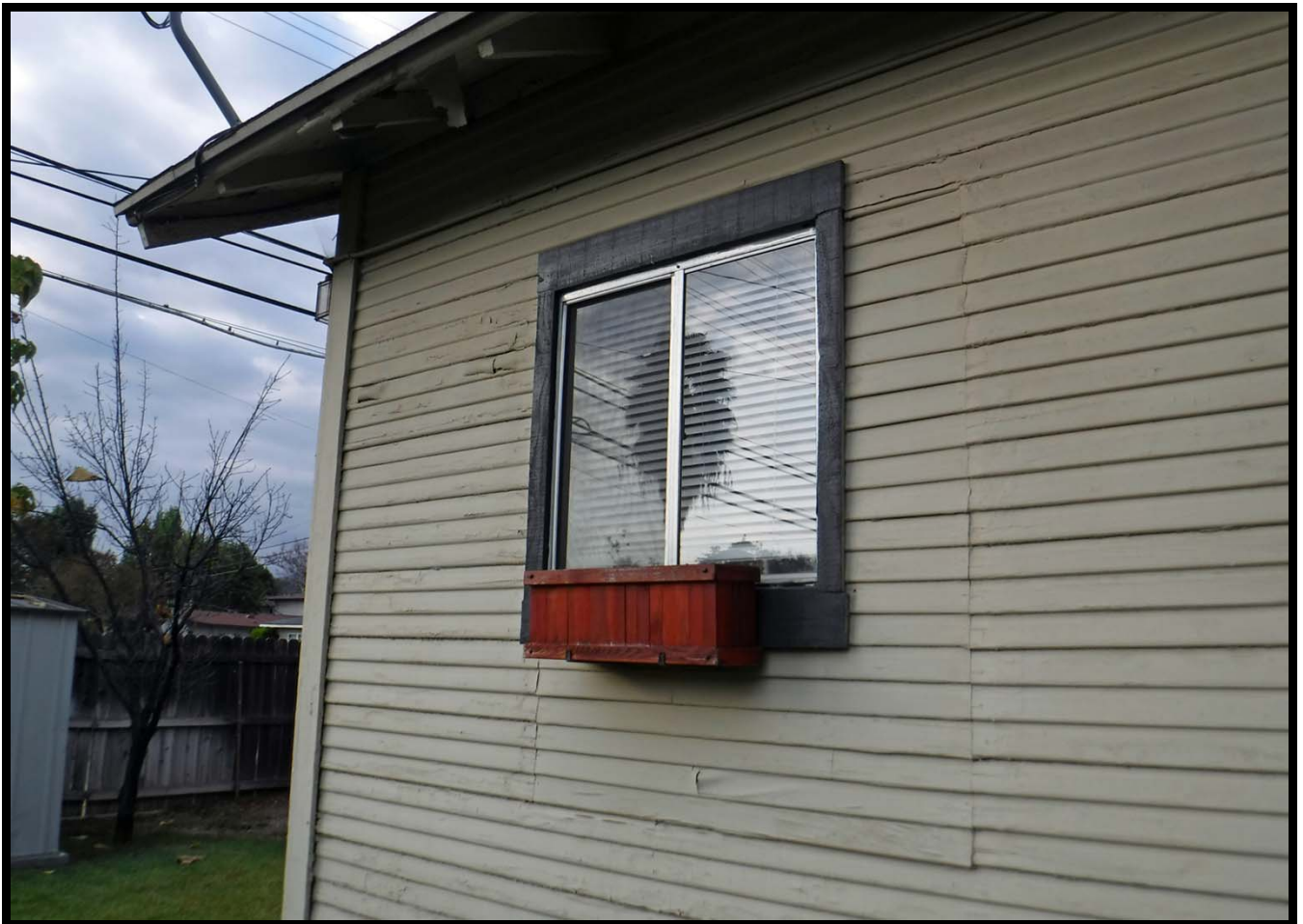
Replaced Window on South Elevation, 448 Linwood Avenue, Monrovia (SW)
