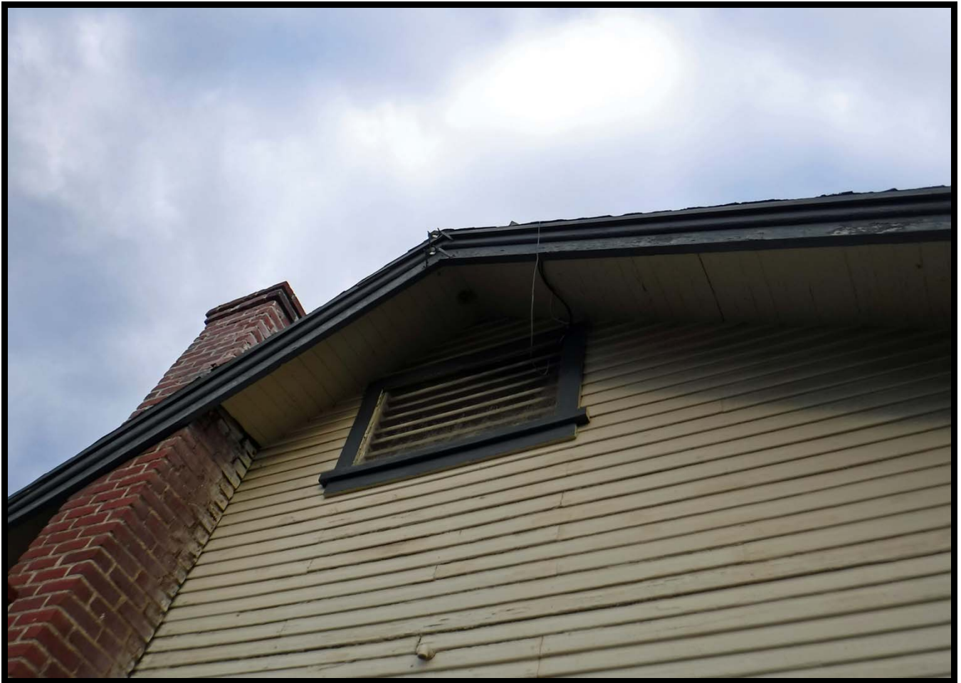
Attic Vent on West Elevation, 448 Linwood Avenue, Monrovia (ENE)
