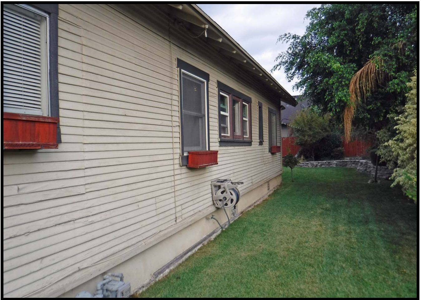
South Elevation of Residence at 448 Linwood Avenue, Monrovia (ENE)
