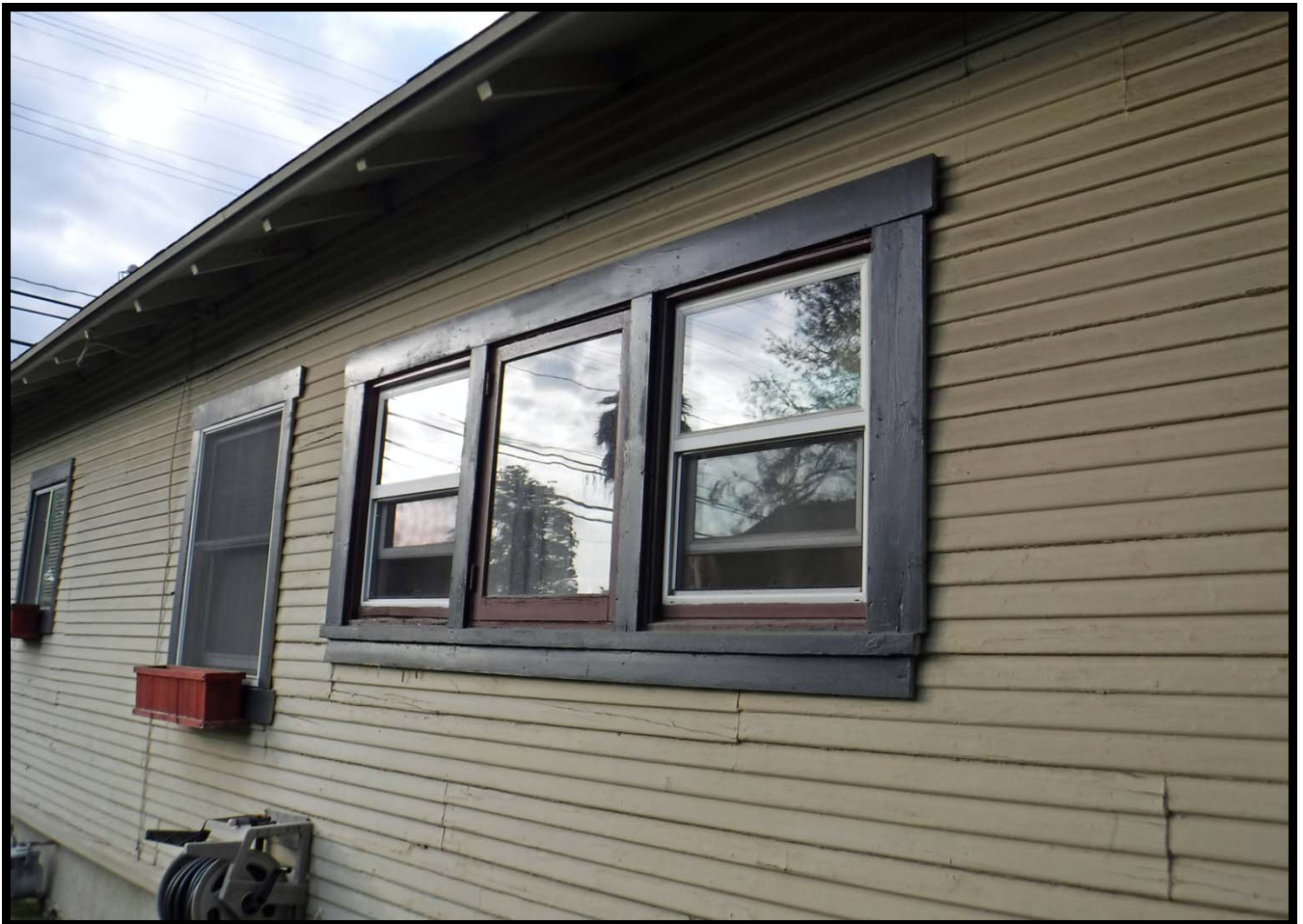
Replaced Windows on South Elevation, 448 Linwood Avenue, Monrovia (NW)
