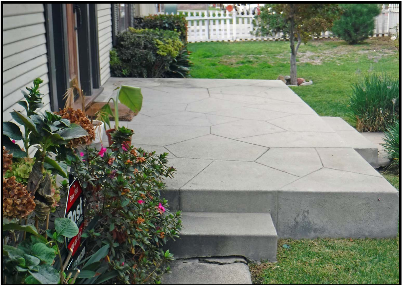
Modern Concrete Stoop on North Elevation, 448 Linwood Avenue, Monrovia (W)
