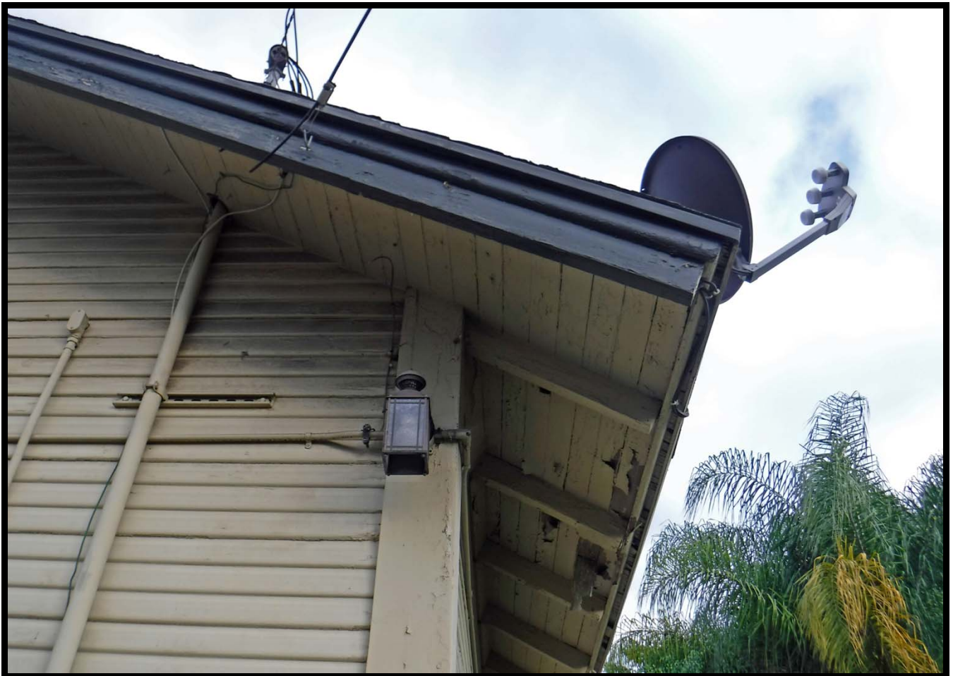
Detail on Southwestern Corner of Residence, 448 Linwood Avenue, Monrovia (W)
