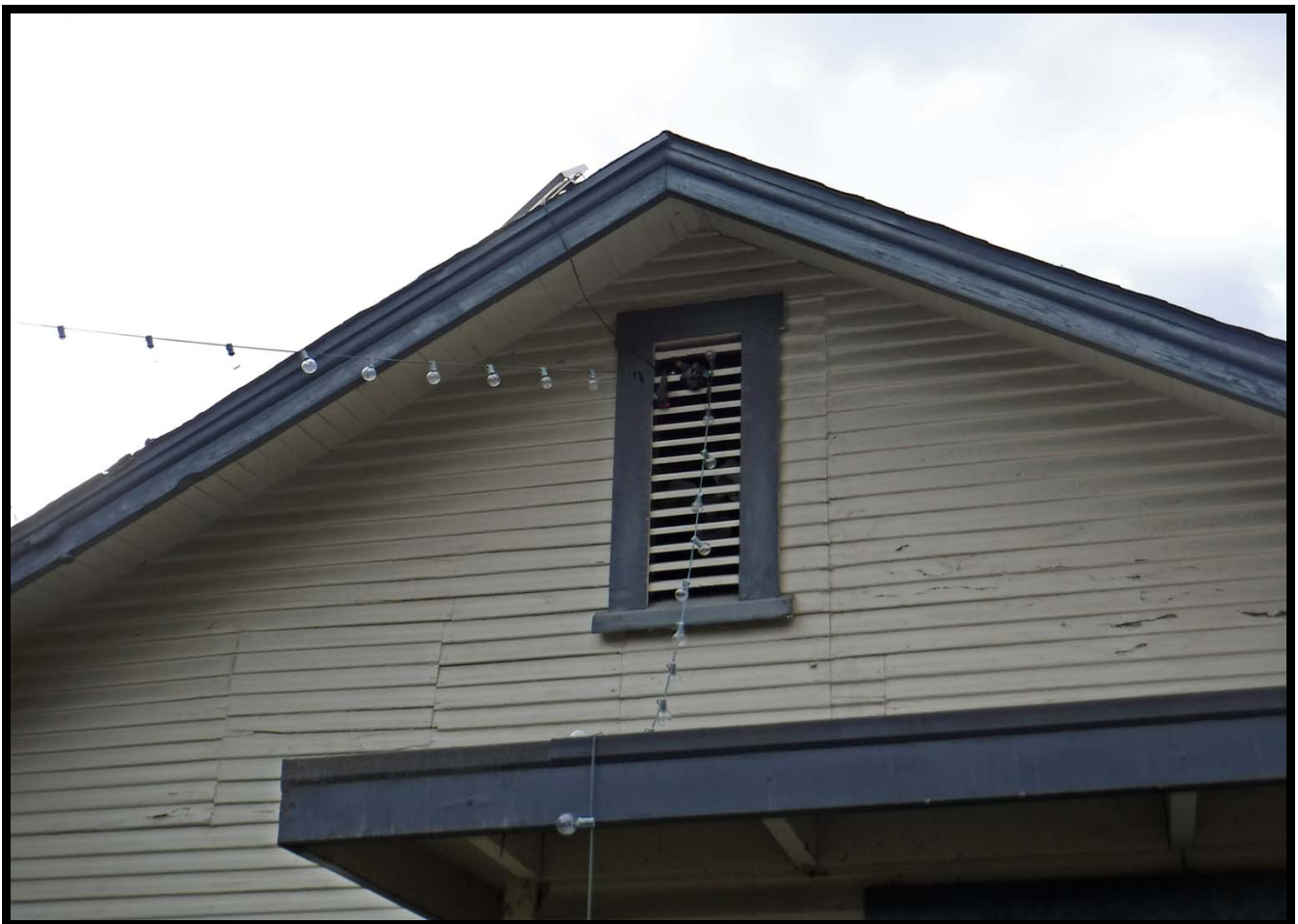
Attic Vent on East Elevation, 448 Linwood Avenue, Monrovia (W)
