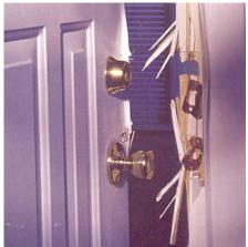
Doors – Solid core wood doors with frames that cannot be spread apart with a pry bar are recommended.
