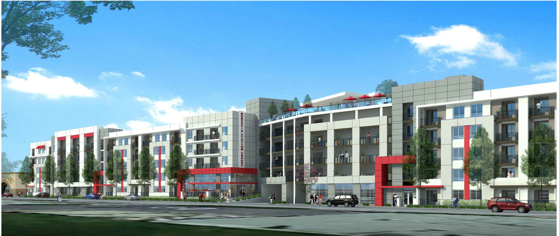
FROM POMONA LOOKING SOUTHEAST
