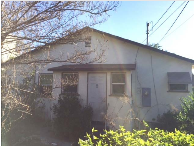
Rear (west) elevation, view to the east (2/4/18)
