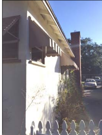
South elevation, taken from the rear of the house, view to the east (2/4/18)
