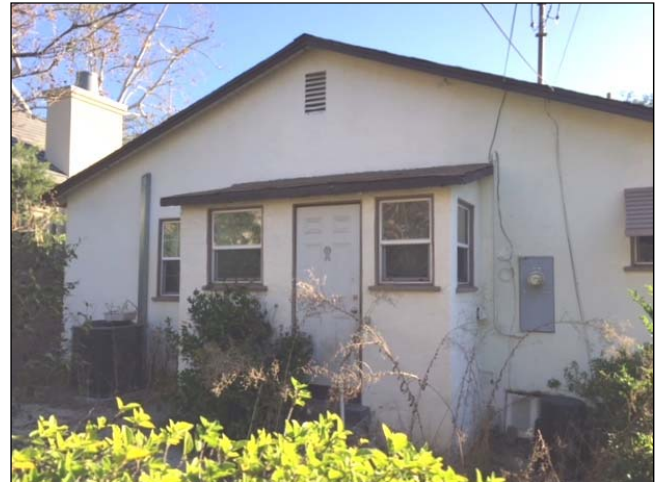
Rear (west) elevation, view to the northeast (2/4/18)
