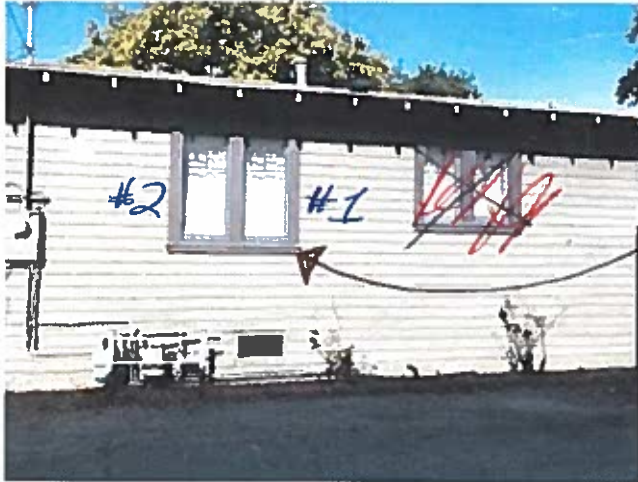
Window Facing South
