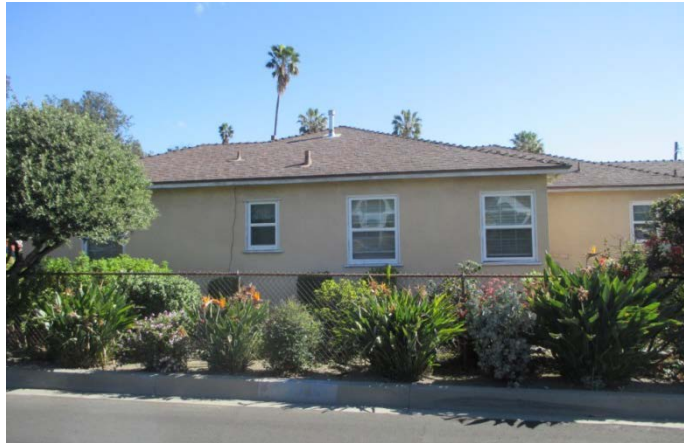
Western Façade, North End, 518 East Olive Avenue
