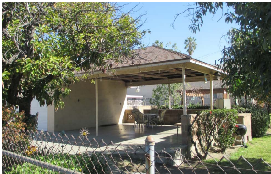
Figure 9. Rear of Property, 518 East Olive Avenue SOURCE: Sapphos Environmental, Inc., 2018
