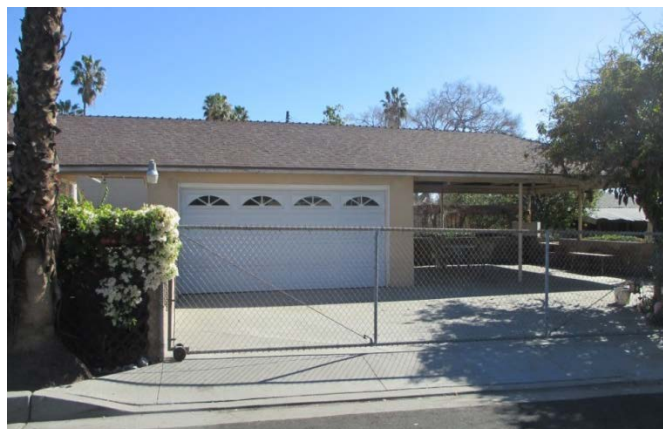
Garage and Carport, South Wing, 518 East Olive Avenue
