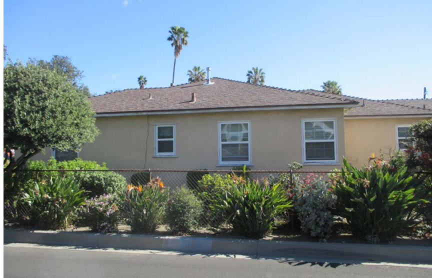
Figure 6. Western Façade, North End, 518 East Olive Avenue SOURCE: Sapphos Environmental, Inc., 2018
