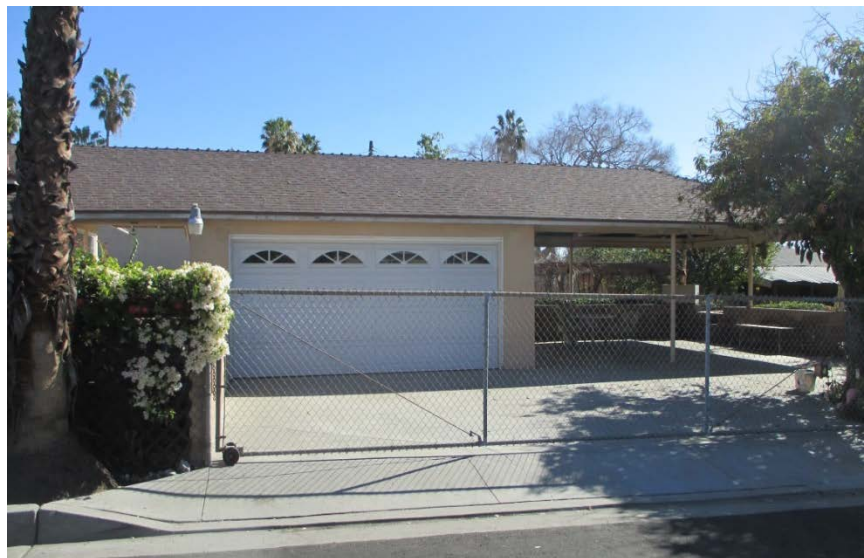
Figure 7. Western Façade, South End, 518 East Olive Avenue SOURCE: Sapphos Environmental, Inc., 2018
