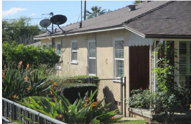
Eastern Façade, 518 East Olive Avenue
