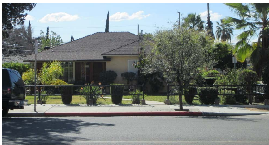
Figure 4. General Street View, House at 518 East Olive Avenue SOURCE: Sapphos Environmental, Inc., 2018
