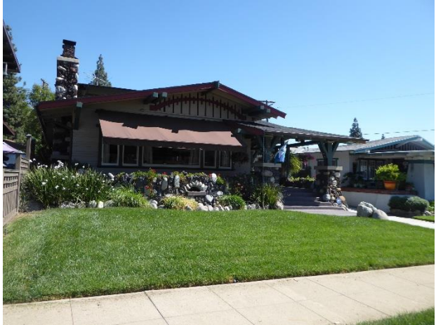
Figure 6.50 West façade of Swiss Chalet-influenced Craftsman at 120 North May Avenue.
