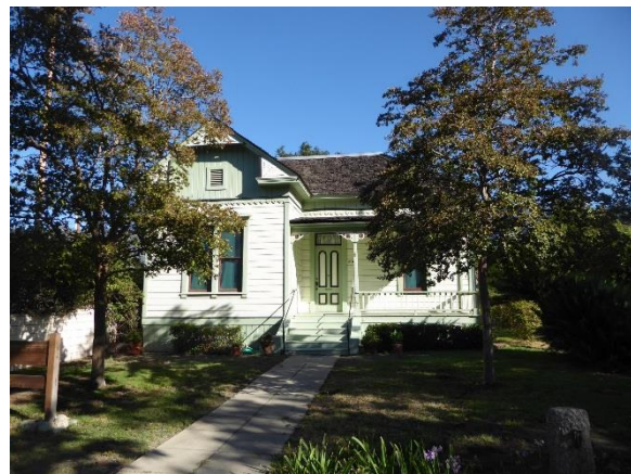
Figure 6.35 South façade of Queen Anne cottage at 215 East Lime Avenue.
