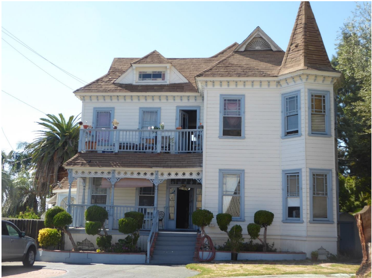
Figure 6.1 Dr. C. Stewart House, an 1887 Folk Victorian with Queen Anne details, looking west.
