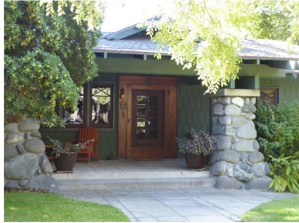
Figure 6.54 Detail of Craftsman bungalow at 316 East Wildrose Avenue, looking south.
