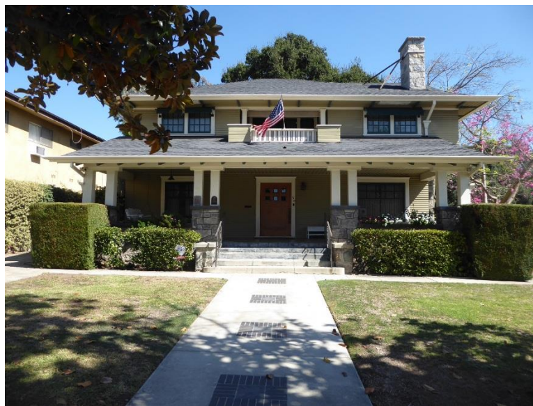
Figure 6.42 West façade of American Foursquare at 130 North Myrtle Avenue.
