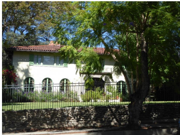
Figure 6.62 South façade of Mediterranean Revival-style home at 131 East Hillcrest Boulevard.
