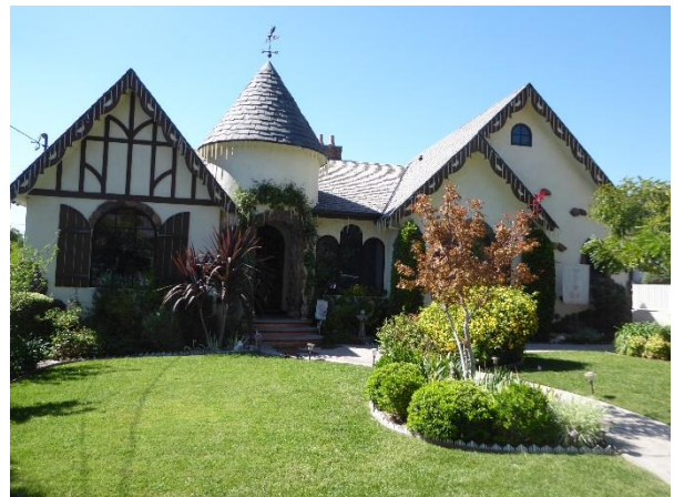
Figure 6.74 East façade of Storybook cottage at 415 North Myrtle Avenue.
