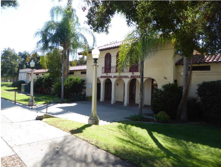
Figure 6.57 Oblique view of Monrovia Historical Museum, looking southeast. An example of the Spanish Colonial Revival style.
