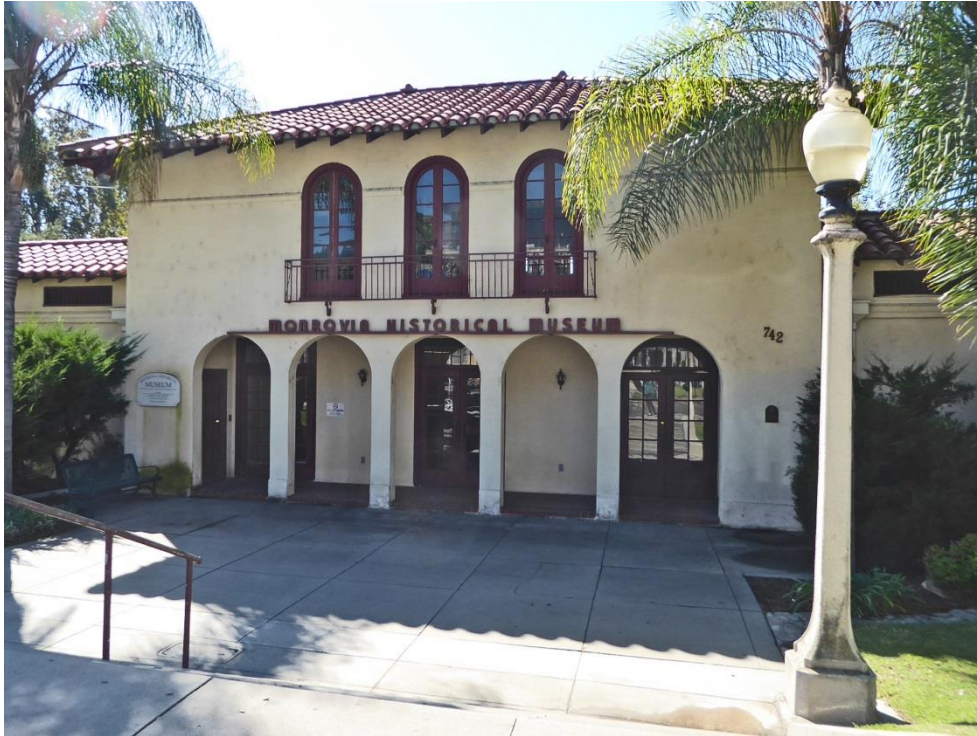
Figure 6.16 Monrovia Historical Museum, formerly the bathhouse for the Municipal Plunge.
