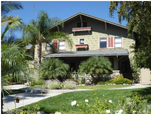
Figure 6.51 South façade of Swiss Chalet-influenced Craftsman at 217 East Greystone Avenue.
