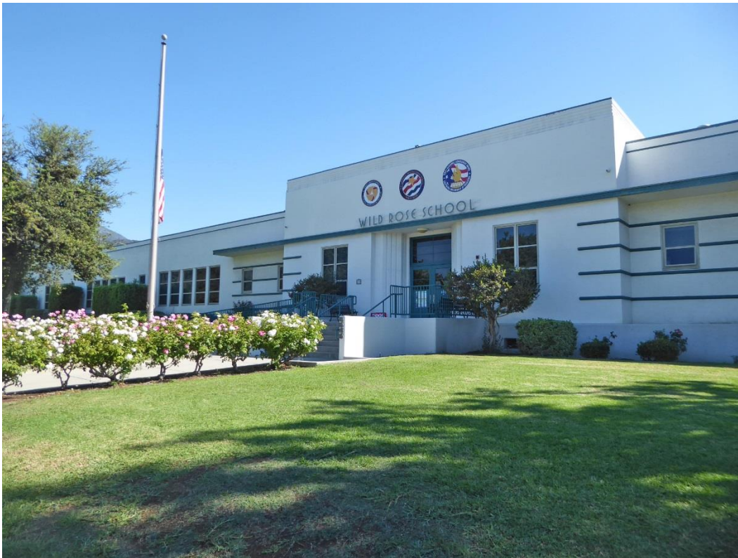
Figure 6.19 Wild Rose School after reconstruction post 1933 Long Beach Earthquake.
