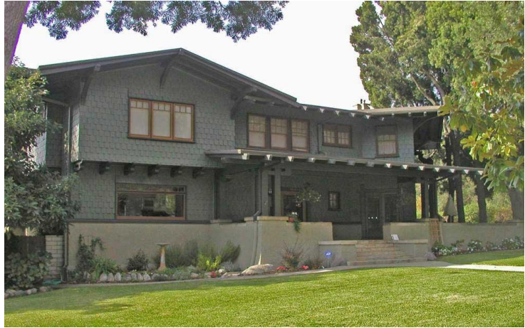
Figure 6.46 Craftsman-style house at 173 Highland Place, looking Northwest.
