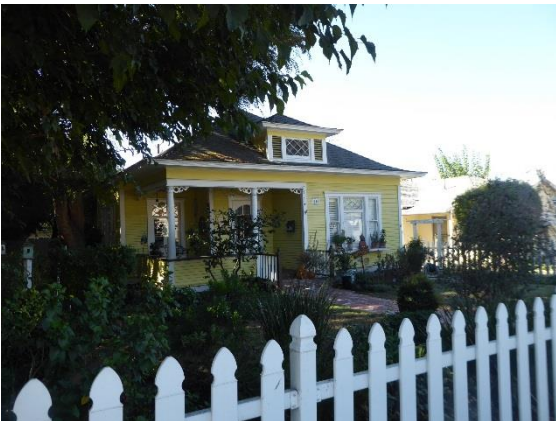
Figure 6.39 Folk Victorian cottage at 234 West Colorado Boulevard, looking southwest.
