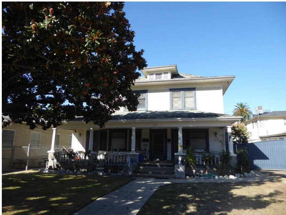
Figure 6.44 American Foursquare at 207 South Magnolia Avenue, looking east.
