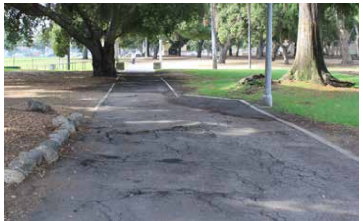
ADA compliance includes having stable surfaces for pathways connecting park amenities. .
