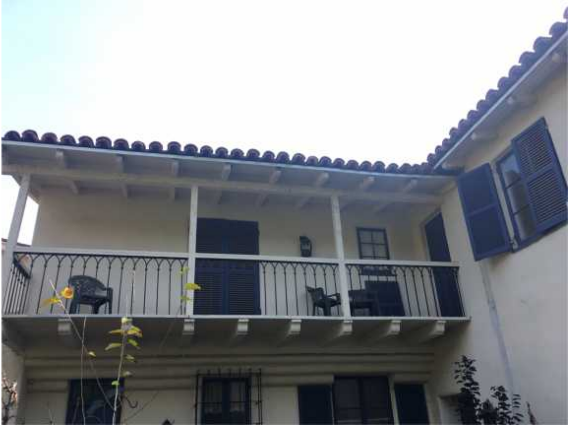
North east corner (facing west) side of the house January 15, 2018.
