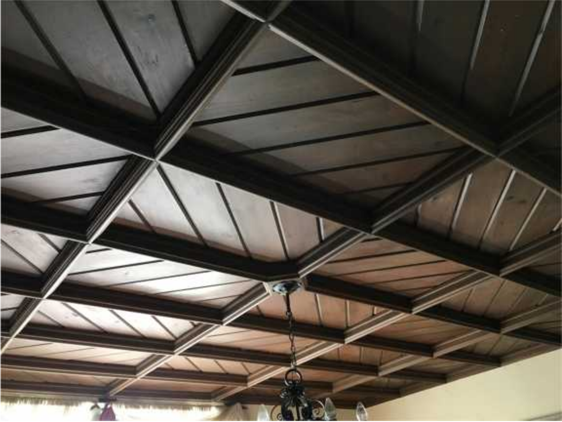
Dining room ceiling close up. January 15, 2018.
