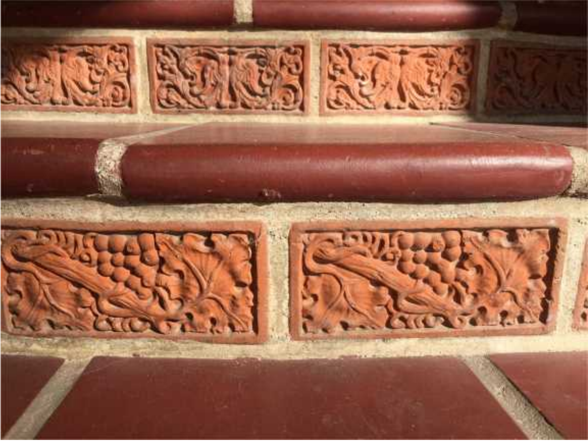
Close up of the outside tile risers January 15, 2018.
