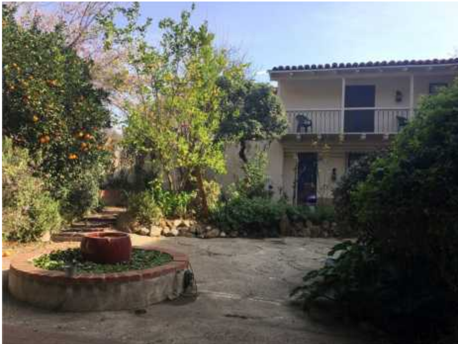
North East corner (facing west) view from the courtyard. (January 2018)
