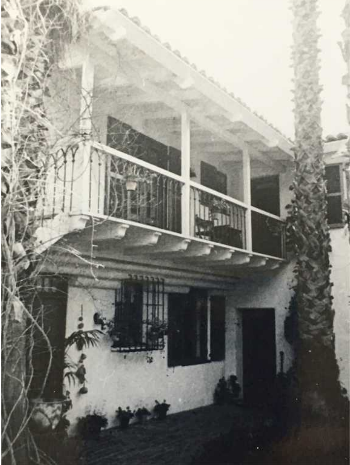
Original view of the North West side of the house.
