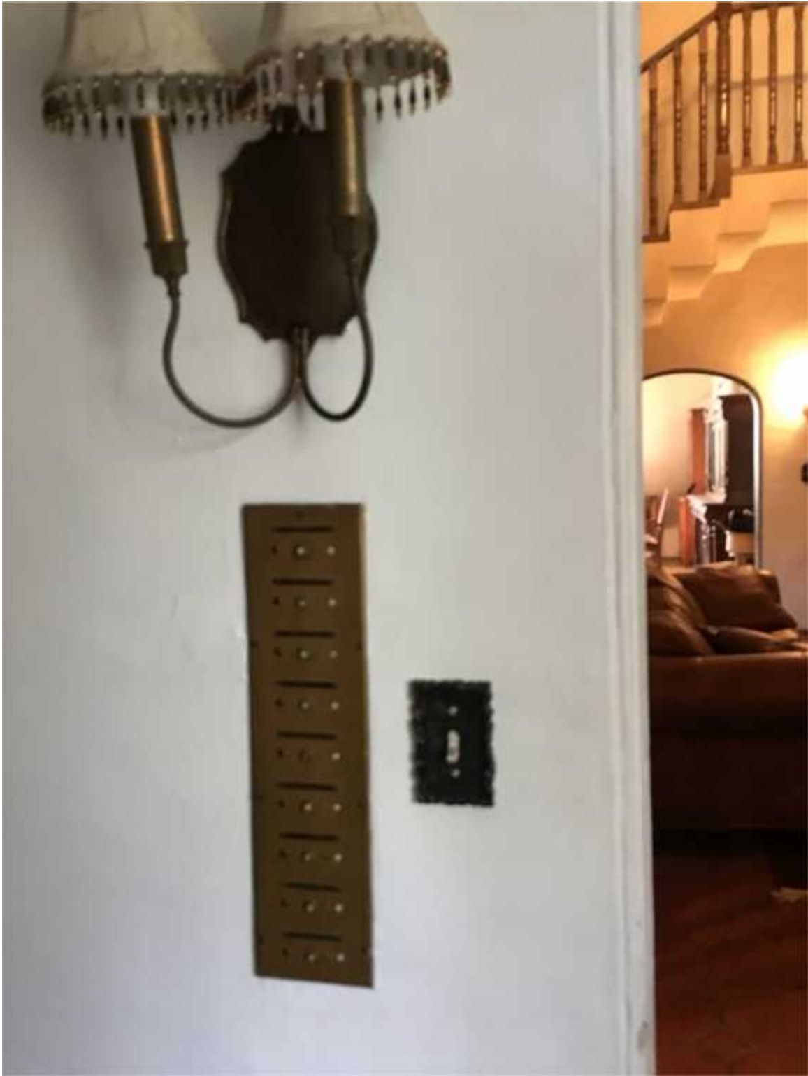
Original call system and light fixture. January 15, 2018.
