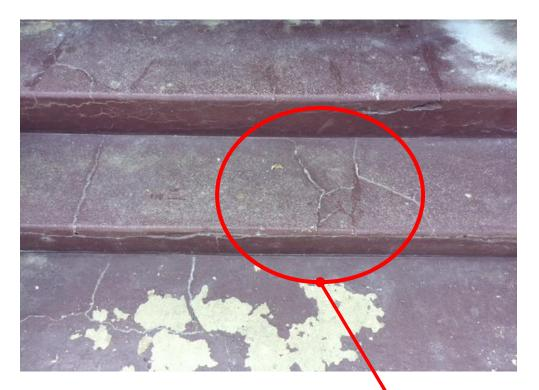
**3. Restoration—Porch Stairs**. Concrete on the steps is cracked. Remove paint, patch with concrete patching compound, and repaint.
