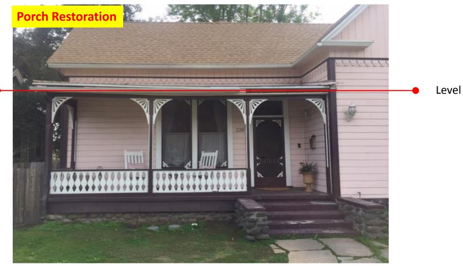
**4.a. Restoration—Porch Roof**. Level roofline of sagging porch. Support pillars of deck in middle have shown evidence of rot, so we would repair these pillars to raise and level roofline. Additionally, we would repair the wood flashing below roofline.
