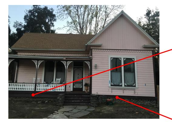
**5. Restoration—Porch Facade**. Make the wooden apron under the window (front right of house) with the same width as the one under the deck (front left side of house). Final width will be determined when porch is complete, likely around 9.0". Aprons around rest of home range from 7.5"- 9.75".
