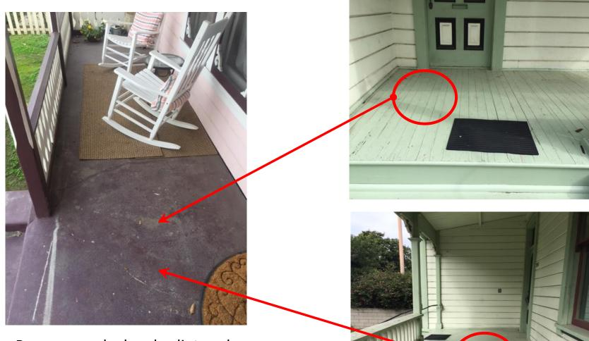
**2. Restoration—Porch Deck.** Remove cracked and splintered concrete topping of front porch and restore deck with Douglas fir planks. Douglas fir is the same material as the original hard wood floors inside home. End goal is to have porch look similar to historical Andersen House on Lime Street (right).
