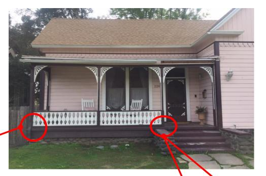
**4.a. Restoration—Porch Roof (continued)**. The posts that support the porch roof sit atop the concrete, but the concrete has cracked and crumbled. The concrete needs to be removed and a level base needs to be established. The posts will be leveled and anchored directly on the new wood porch.
