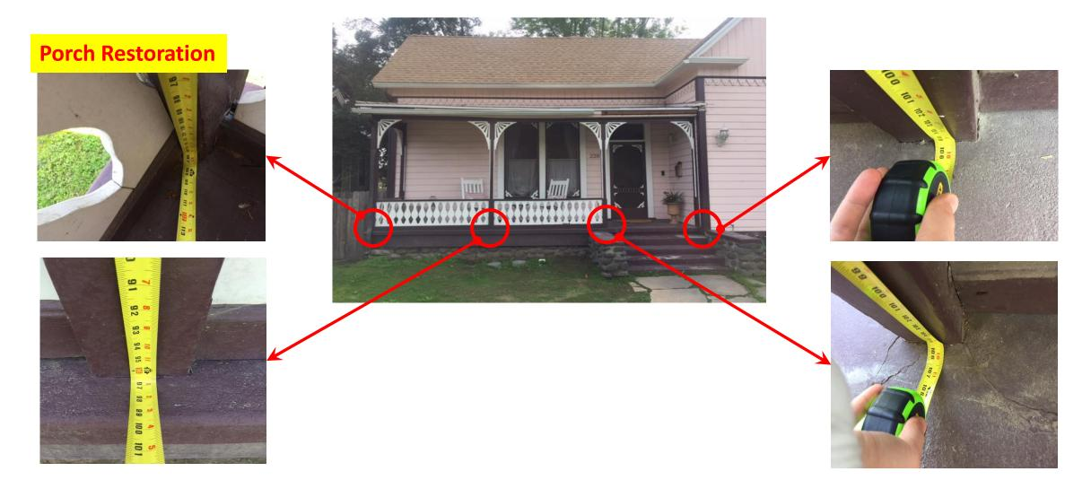
**4.a. Restoration—Porch Roof (continued)**. The posts that hold up the roof are uneven. After a level porch is established, wood blocks would be used to make the posts and the roof an even height.
