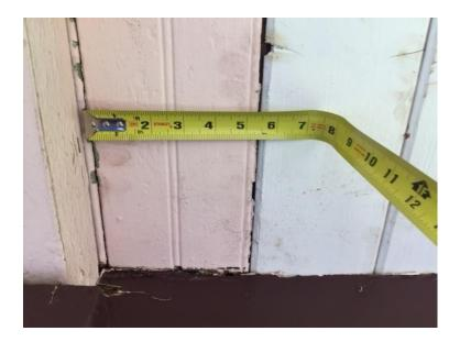
**4.b. Restoration—Porch Ceiling (continued)**. A closer look at wood planking on ceiling. The white patches (top right) would be replaced with in-kind materials cut to match the façade of the existing planks (bottom right) and restore the original character.
