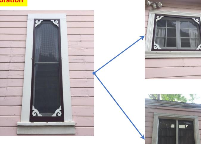
**1. Restoration—Windows (continued)**. The exterior frame, ledge, and apron on the picture above will be replicated on the two windows to right. Material will be red wood.
