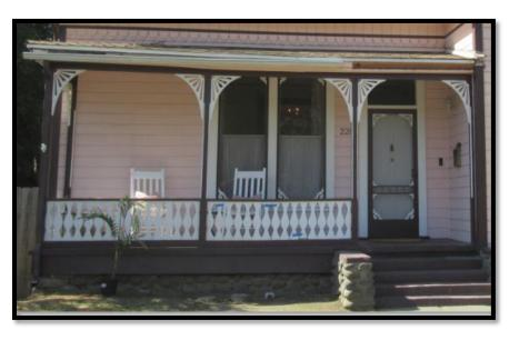
Additionally, the homeowners are proposing to fully restore the front porch, which is a condition of their Mills Act contract. This will include the removal of the concrete floor and installation of Douglas Fir wood planking, repair and shoring of rotting support posts, repair of the concrete stairs, restoration of bead board ceiling planks, and levelling of the sagging porch roofline. The photograph to the left shows the porch in its current condition. Though
