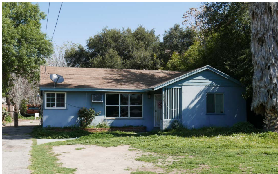
Figure 4. View of Primary (Southern) Façade, 405 Genoa Street
