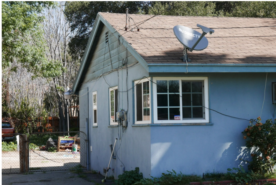
Figure 6. View of Western Façade, 405 Genoa Street SOURCE: Sapphos Environmental, Inc., 2018
