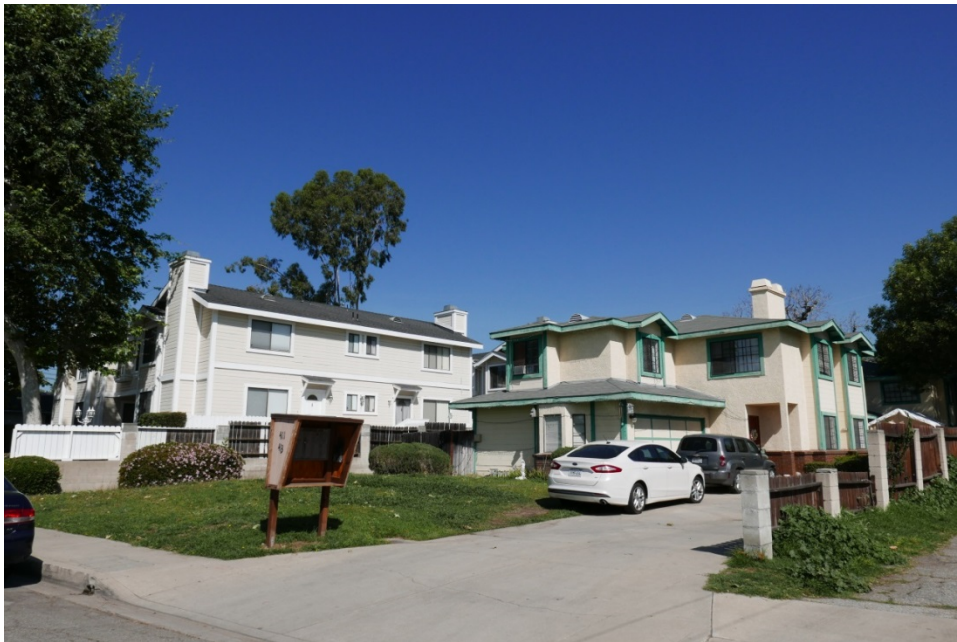
Figure 9. Properties to the West of 405 Genoa Street SOURCE: Sapphos Environmental, Inc., 2018
