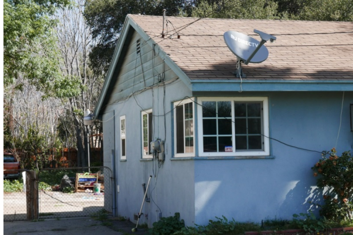
View of Western Facade, 405 Genoa Street
