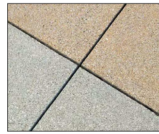
CONCRETE POOL DECK
