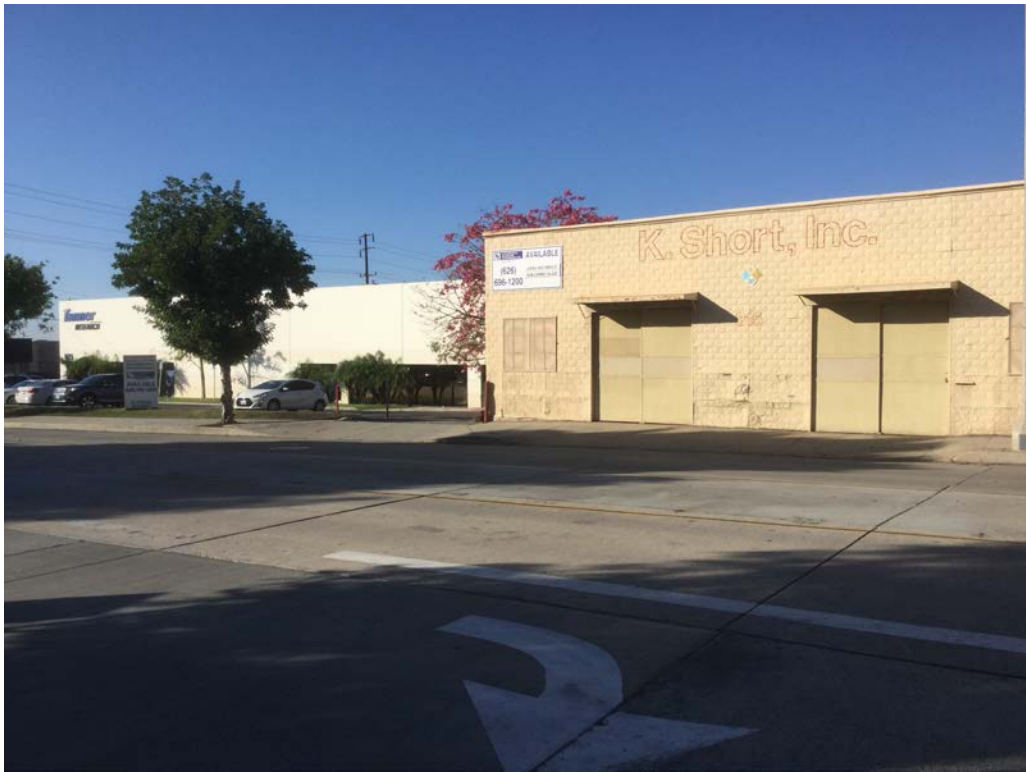
View of subject property to the southwest. 815 & 825 S. Myrtle Avenue, Monrovia, California 91016
