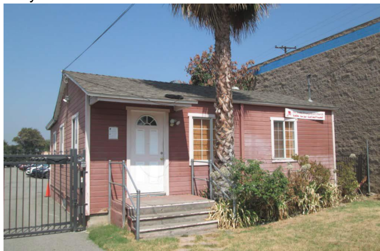
Figure 1. Photo of 1607 South Magnolia as seen from the street. The structure was constructed circa 1910-1930.
