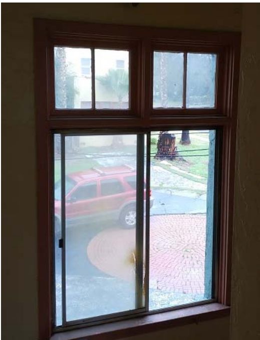
Image 03 - Stairwell Combination Window
