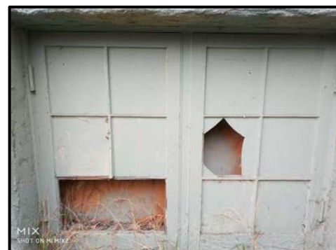
Figure 1 – Last Remaining Original Wood Window
