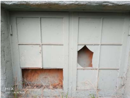
Image 02 - Basement Window Closer View
