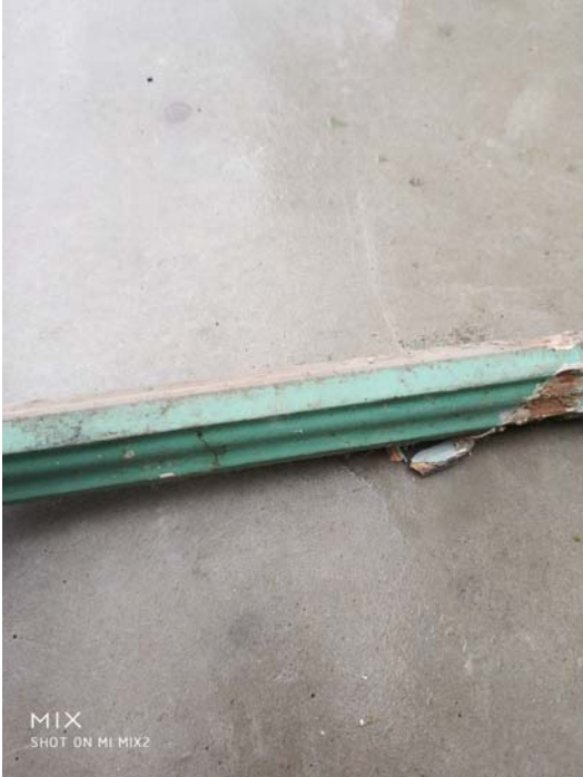
Image 03 - Inside View of Mullion (Grid)
