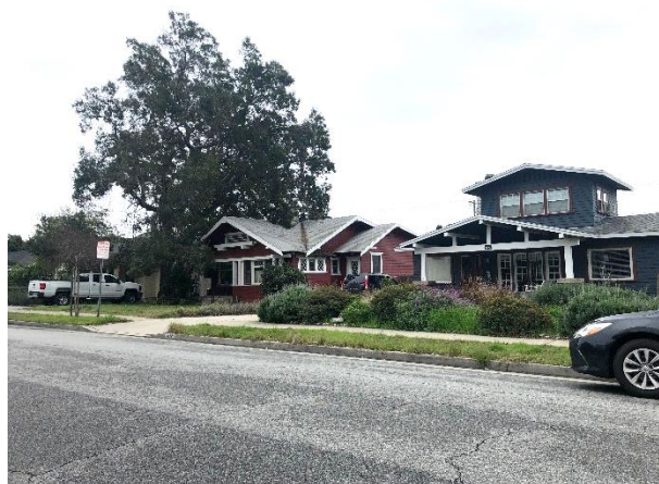
Setting, E. Lemon Avenue Facing West
