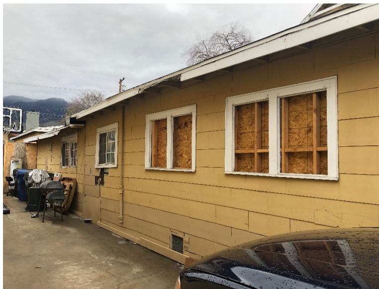
Figure 10. View of Eastern Façade, 511 E. Lemon Avenue SOURCE: Sapphos Environmental, Inc., 2019
