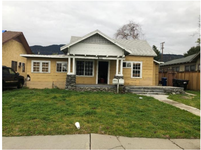
Figure 1 - Primary View of 511 East Lemon Avenue (Facing South), February 2019
