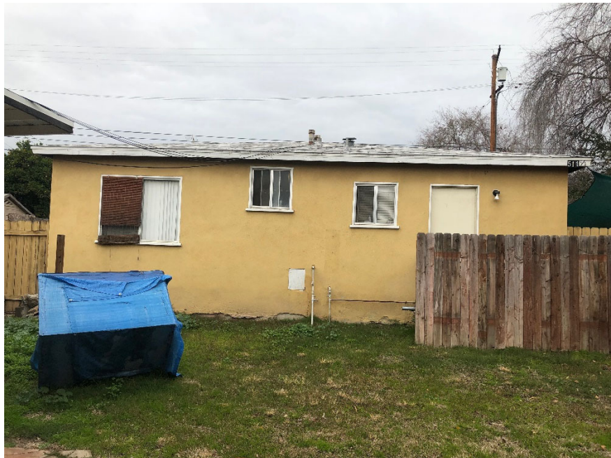
Figure 13. View of Southern Façade, Rear Residence, 511 ½ E. Lemon Avenue SOURCE: Sapphos Environmental, Inc., 2019
