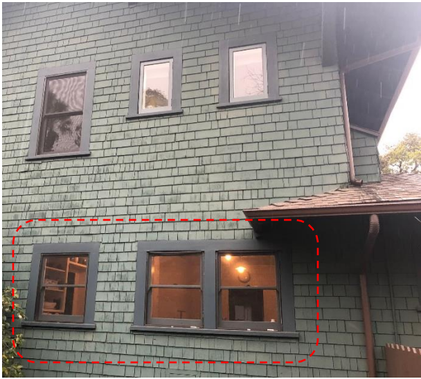
Figure 2. Exterior view: north elevation and kitchen windows on the first floor.
