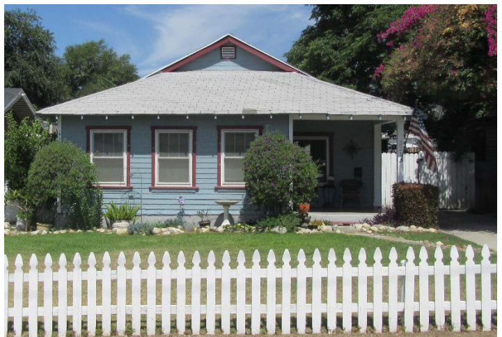
Figure 1. Photo of 221 Norumbega Drive as seen from the street. The structure was originally constructed in 1922 and altered in 1944.
