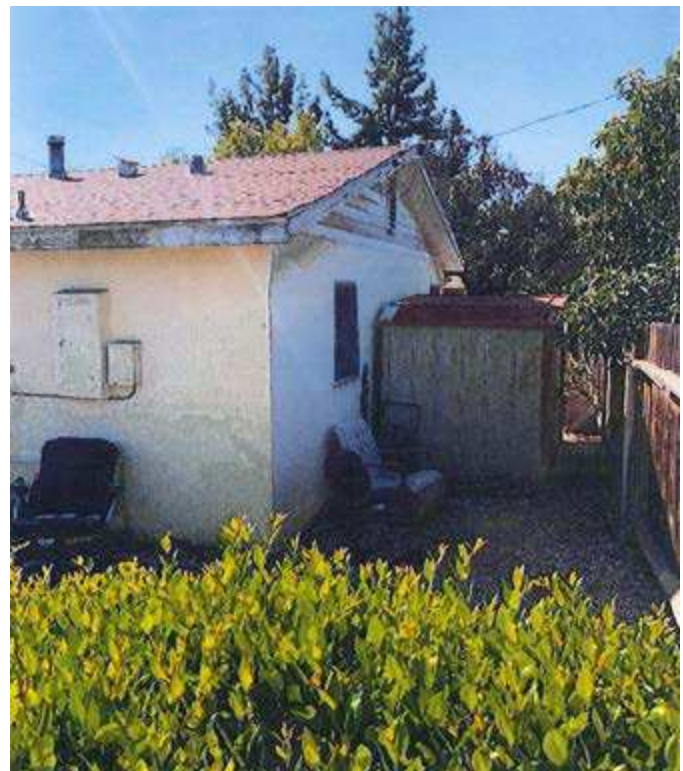
Figure 5. View of Western Facade, 431 ½ W. Lemon Avenue SOURCE: C.B. Home, Inc., 2019
