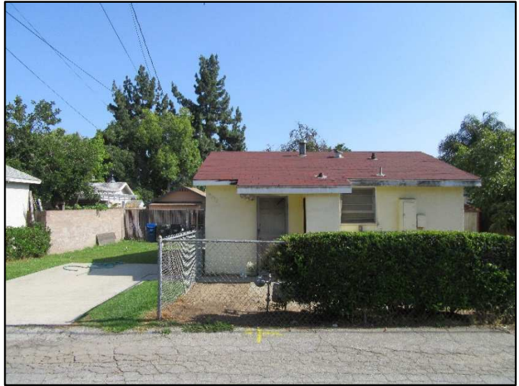
Figure 2. Photo of 431 ½ West Lemon Avenue as seen from the alley. The structure was constructed in 1947.
