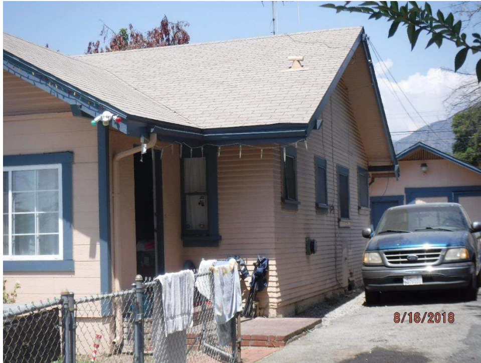
Figure 9. View of Eastern Façade, 431 W. Lemon Avenue SOURCE: Sapphos Environmental, Inc., 2018
