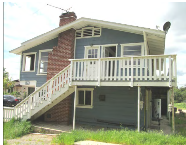
Northeast elevation, view to the southwest (4/5/19)
