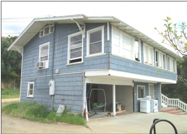
Southwest elevation, view to the northeast (4/5/19)
