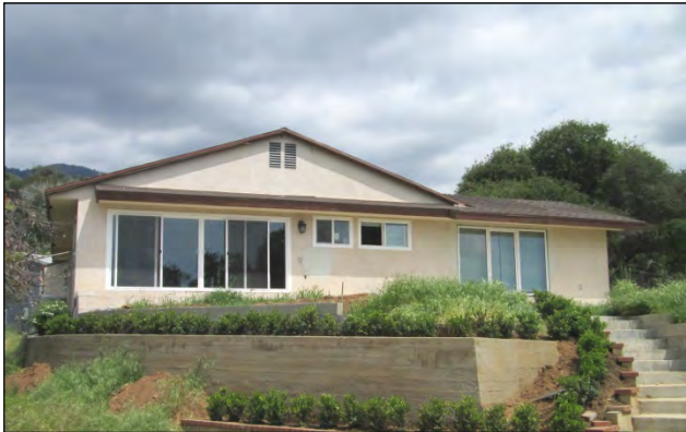
Southeast elevation, view to the northeast.
