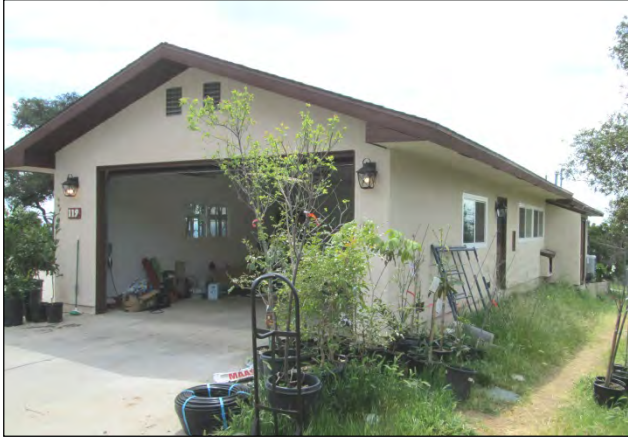
Northeast and northwest elevations (partial), view to the south.
