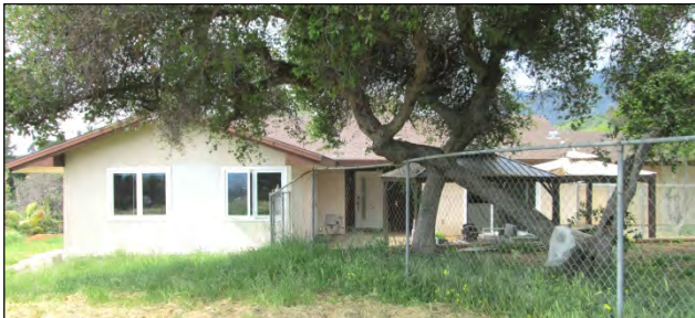
Southeast elevation (partial), view to the northwest.
