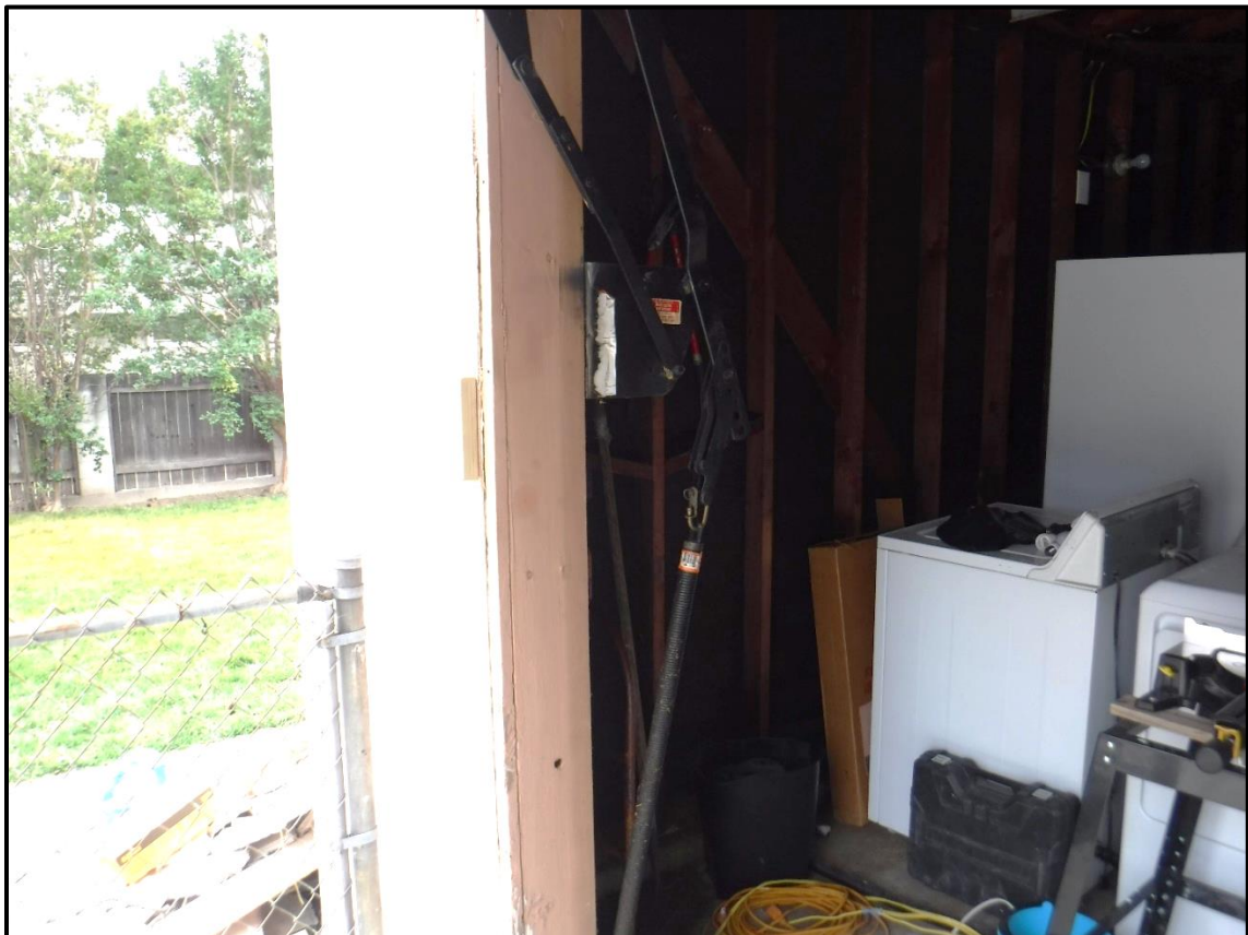
Spring Action within Garage, 1213 S. California Avenue, Monrovia, CA (SW)
