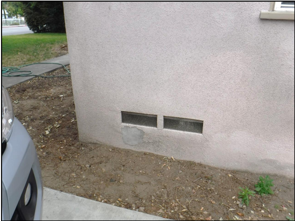
Floor Vents, North Elevation, 1213 S. California Avenue, Monrovia, CA (SSE)
