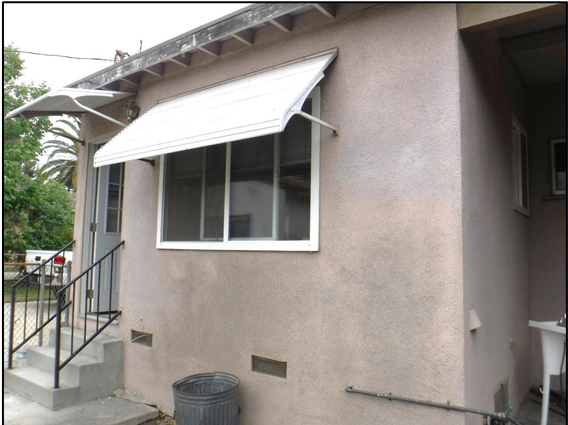
Window Detail, West Elevation, 1213 S. California Avenue, Monrovia, CA (NE)
