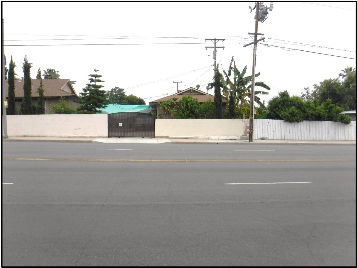
402 E. Cypress Avenue; West Elevation on S. California Avenue, Monrovia, CA (1965-70; E)
