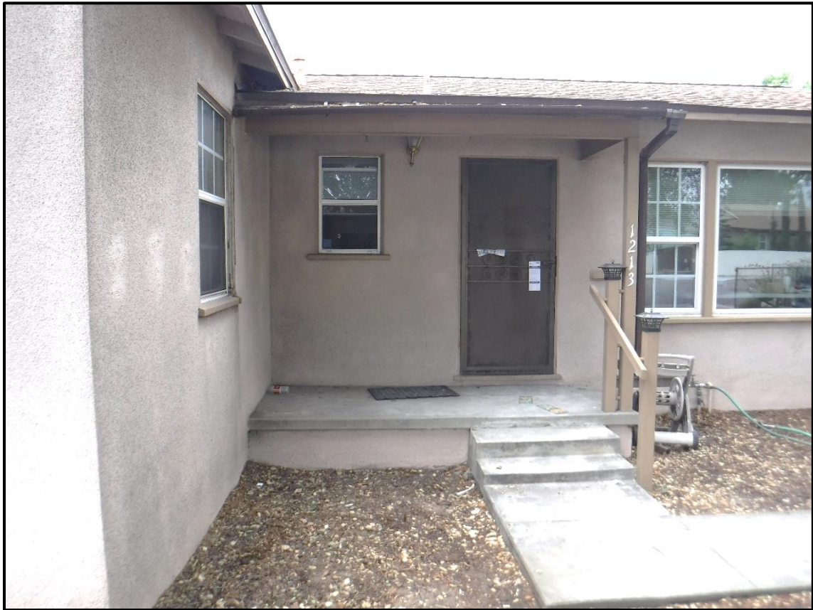
East Elevation, 1213 S. California Avenue, Monrovia, CA (W)
