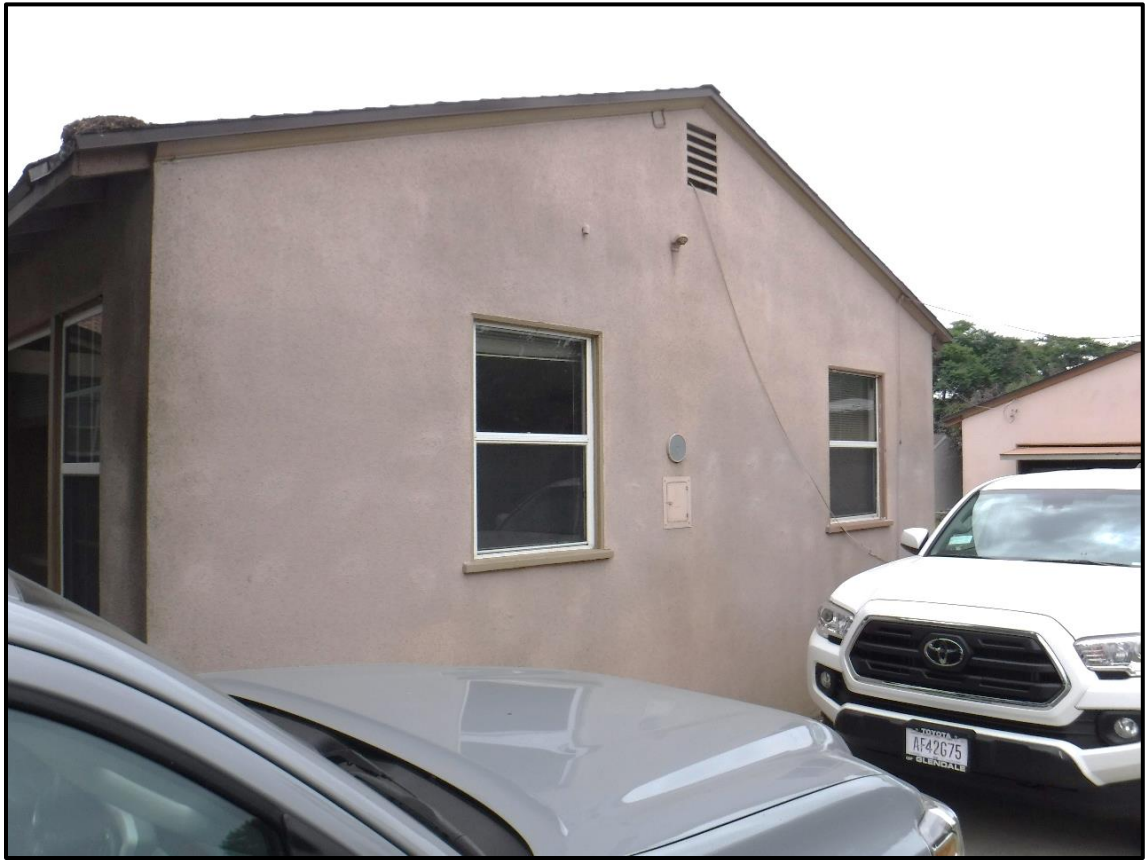
North Elevation, 1213 S. California Avenue, Monrovia, CA (SW)
