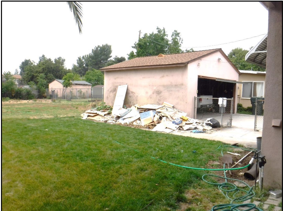
South Elevation of Garage, 1213 S. California Avenue, Monrovia, CA (NW)
