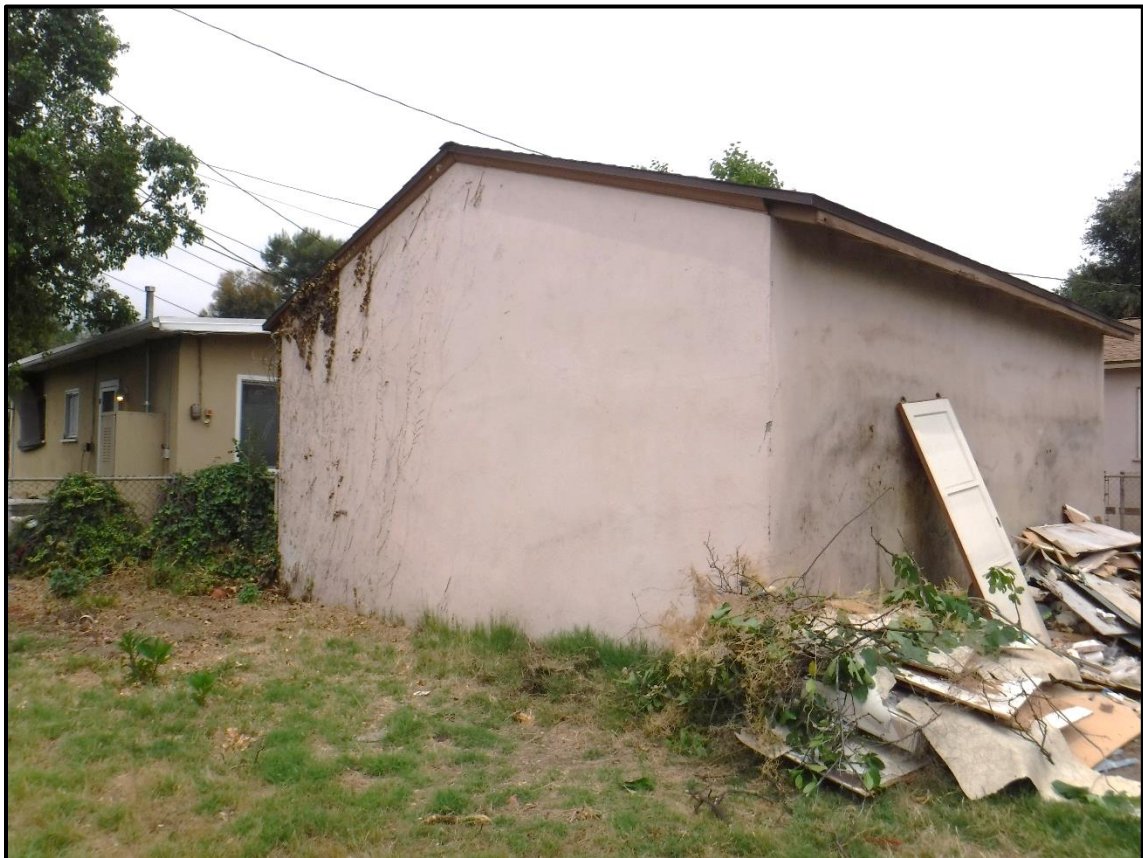
West Elevation of Garage, 1213 S. California Avenue, Monrovia, CA (NE)
