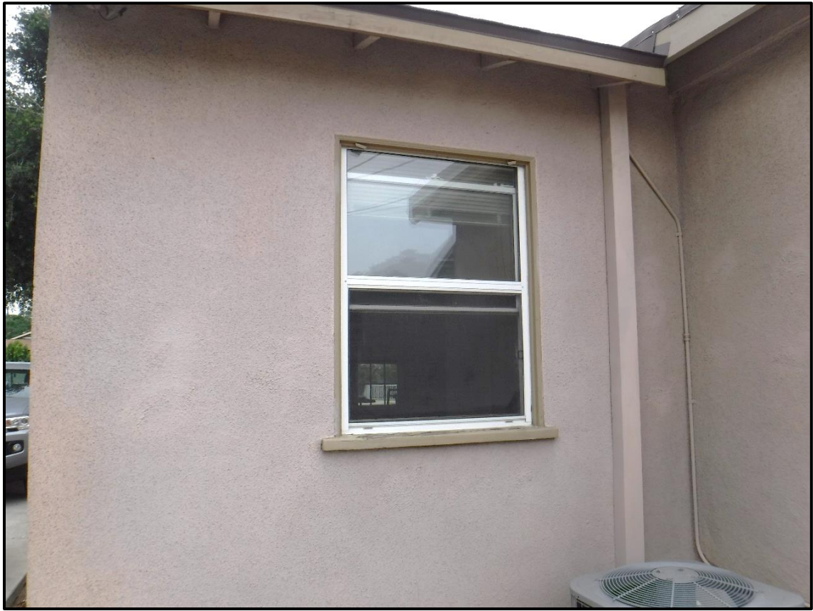
Window Detail, West Elevation, 1213 S. California Avenue, Monrovia, CA (ESE)
