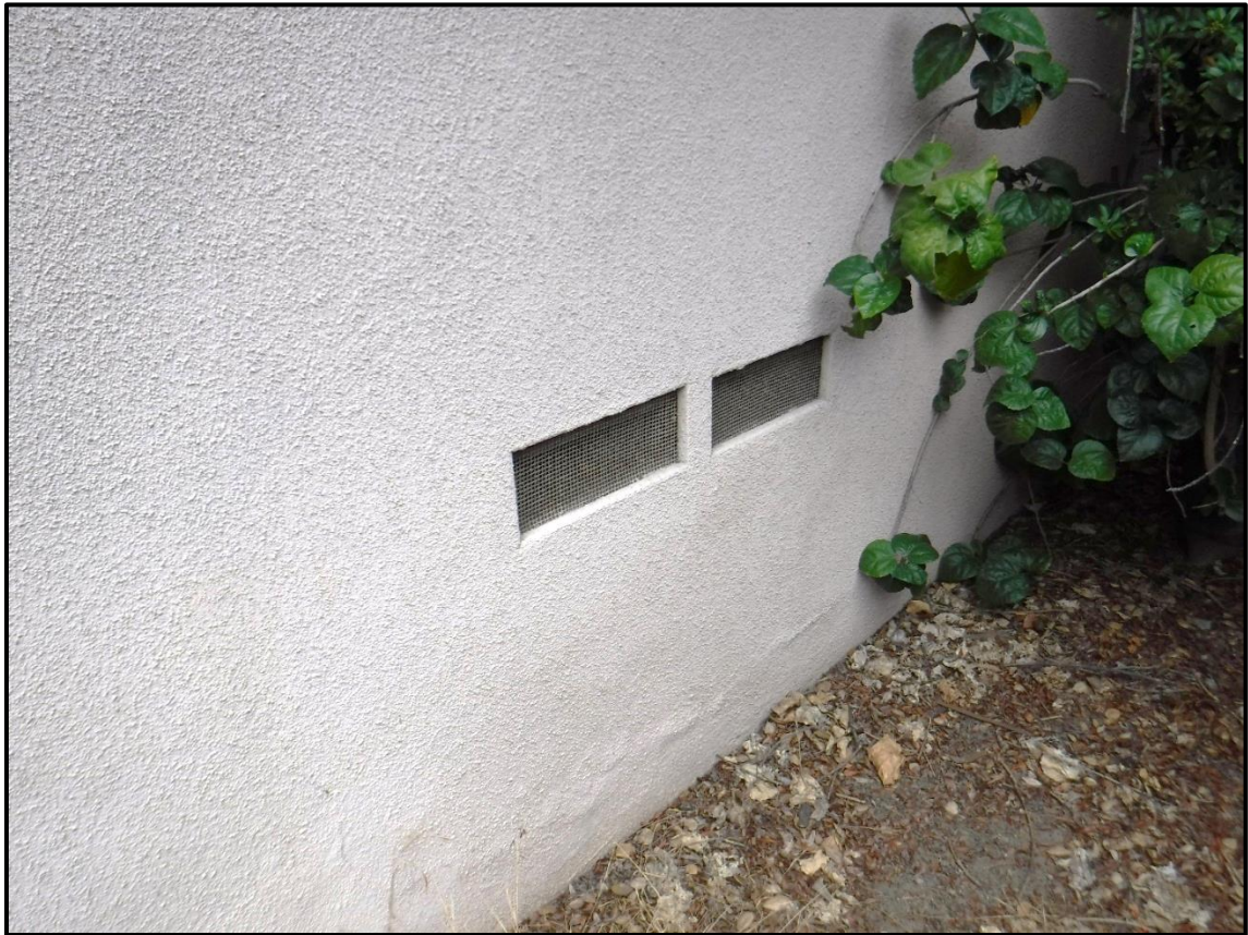
Floor Vents, South Elevation, 1213 S. California Avenue, Monrovia, CA (NE)
