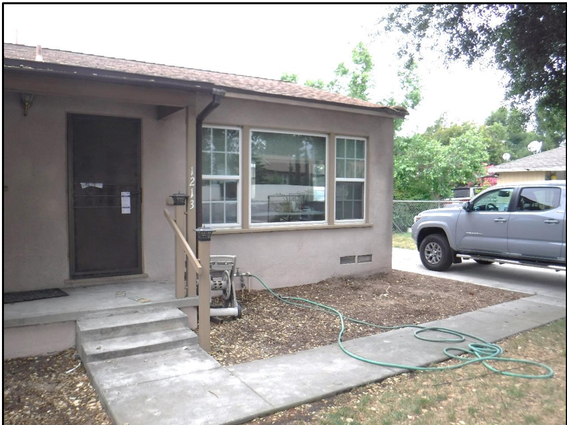
East Elevation, 1213 S. California Avenue, Monrovia, CA (SW)
