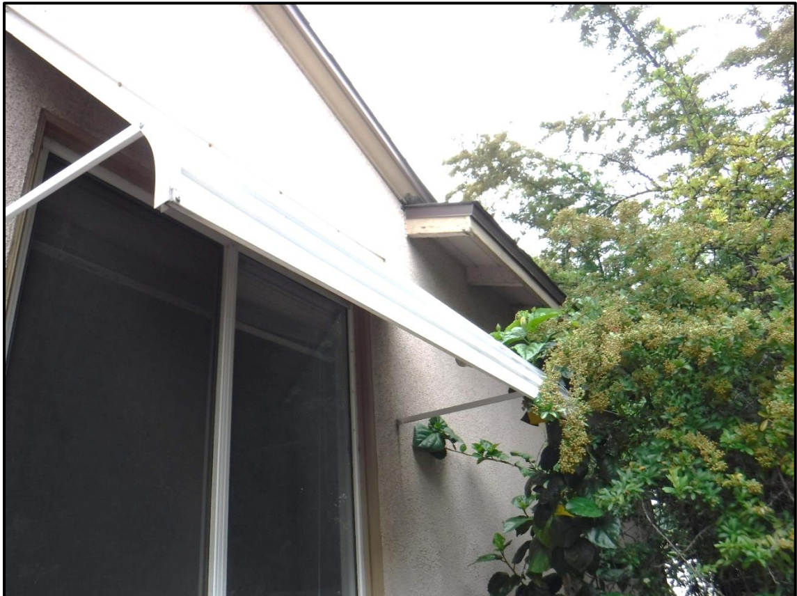
Window Detail (w/awning), South Elevation, 1213 S. California Avenue, Monrovia, CA (ENE)
