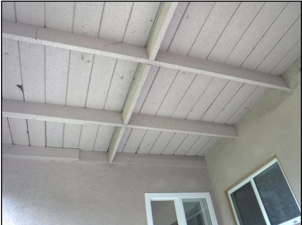
Roofing above Rear Patio, 1213 S. California Avenue, Monrovia, CA (NNE)
