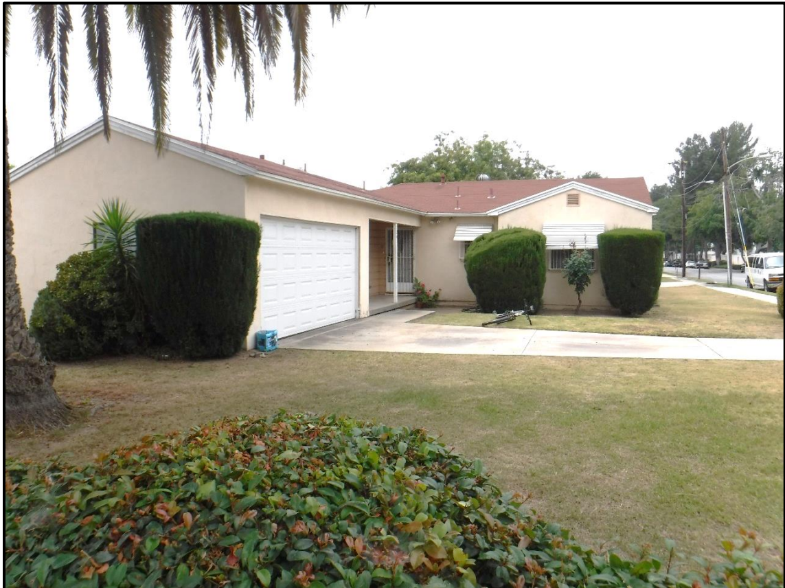
Residence at 1201 S. California Avenue, Monrovia, CA (1955-56; NW)
