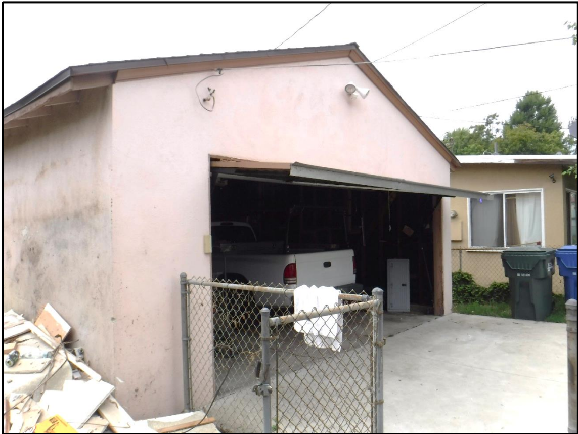
East Elevation of Garage, 1213 S. California Avenue, Monrovia, CA (NW)
