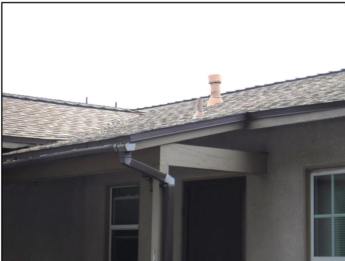
Roof Line, West Elevation, 1213 S. California Avenue, Monrovia, CA (SW)
