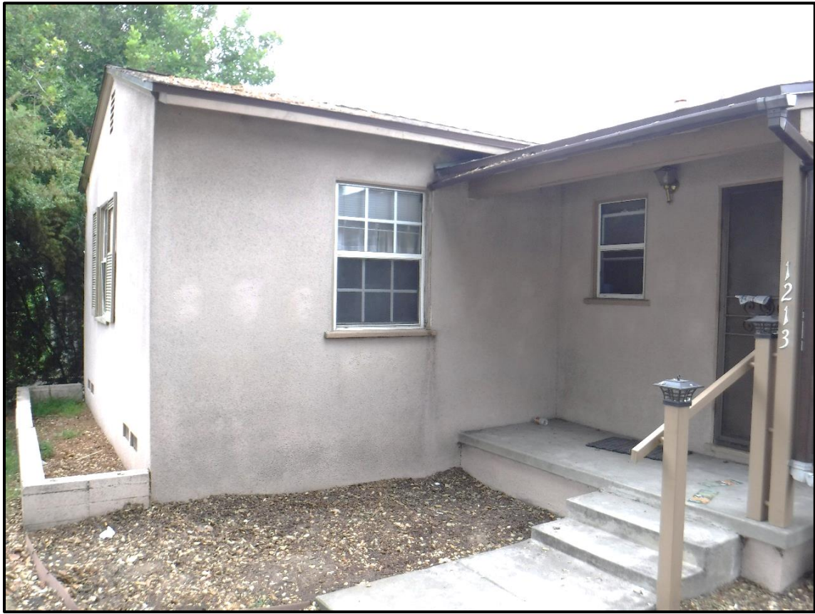
East and North Elevations, 1213 S. California Avenue, Monrovia, CA (SW)
