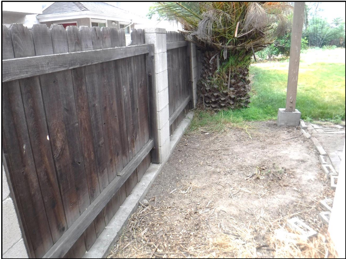
Fencing on South Boundary, 1213 S. California Avenue, Monrovia, CA (WSW)
