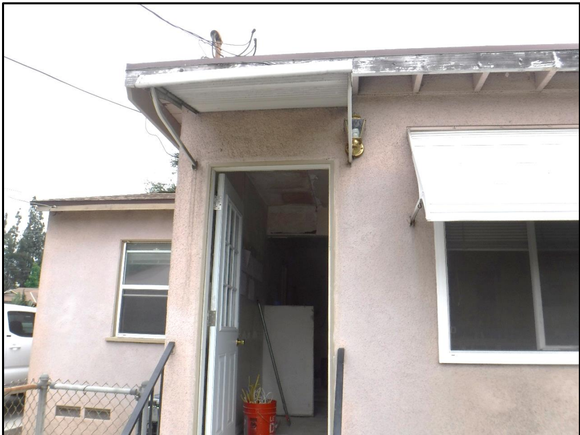
Secondary Doorway on West Elevation, 1213 S. California Avenue, Monrovia, CA (E)
