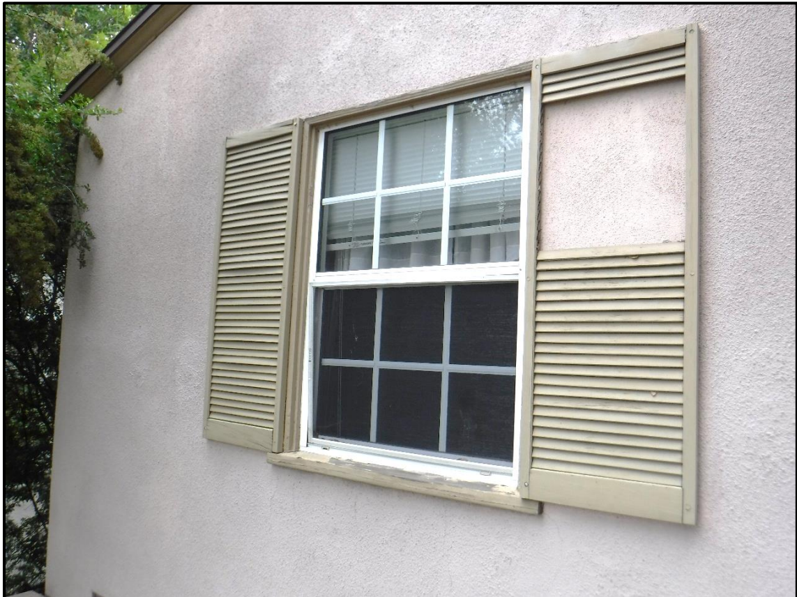
Window Detail, East Elevation, 1213 S. California Avenue, Monrovia, CA (SW)
