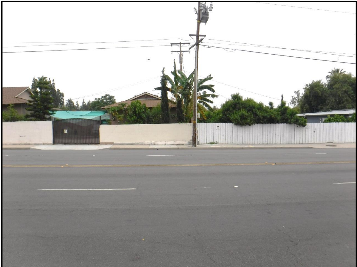
402 E. Cypress Avenue; West Elevation on S. California Avenue, Monrovia, CA (1965-70; E)
