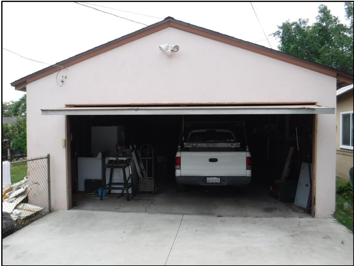
East Elevation of Garage, 1213 S. California Avenue, Monrovia, CA (W)
