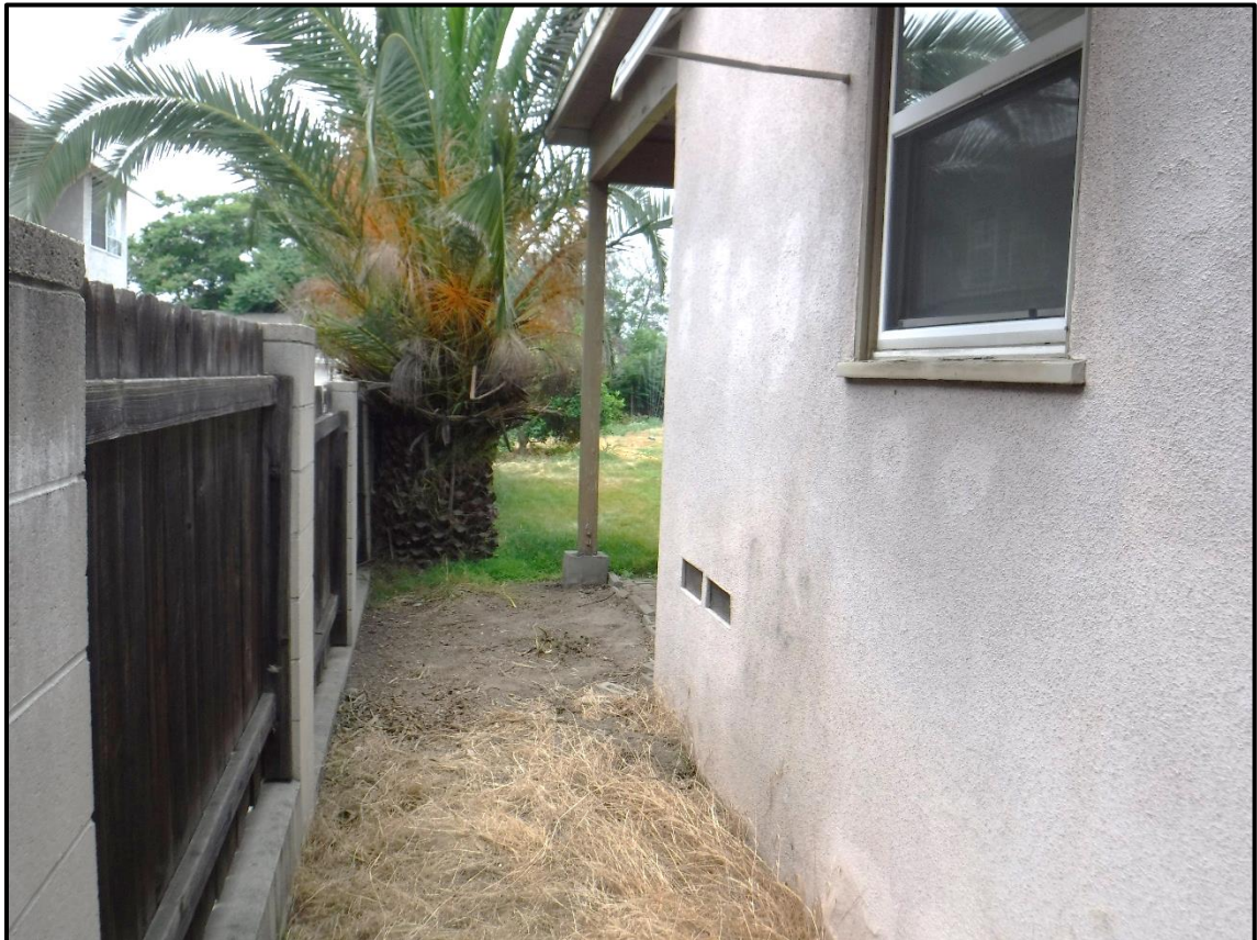
South Property Boundary, 1213 S. California Avenue, Monrovia, CA (W)
