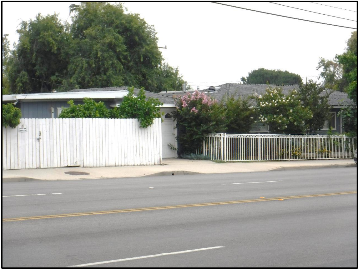
401 E. Cherry Avenue; West Elevation on S. California Avenue, Monrovia, CA (1950-60; SE)
