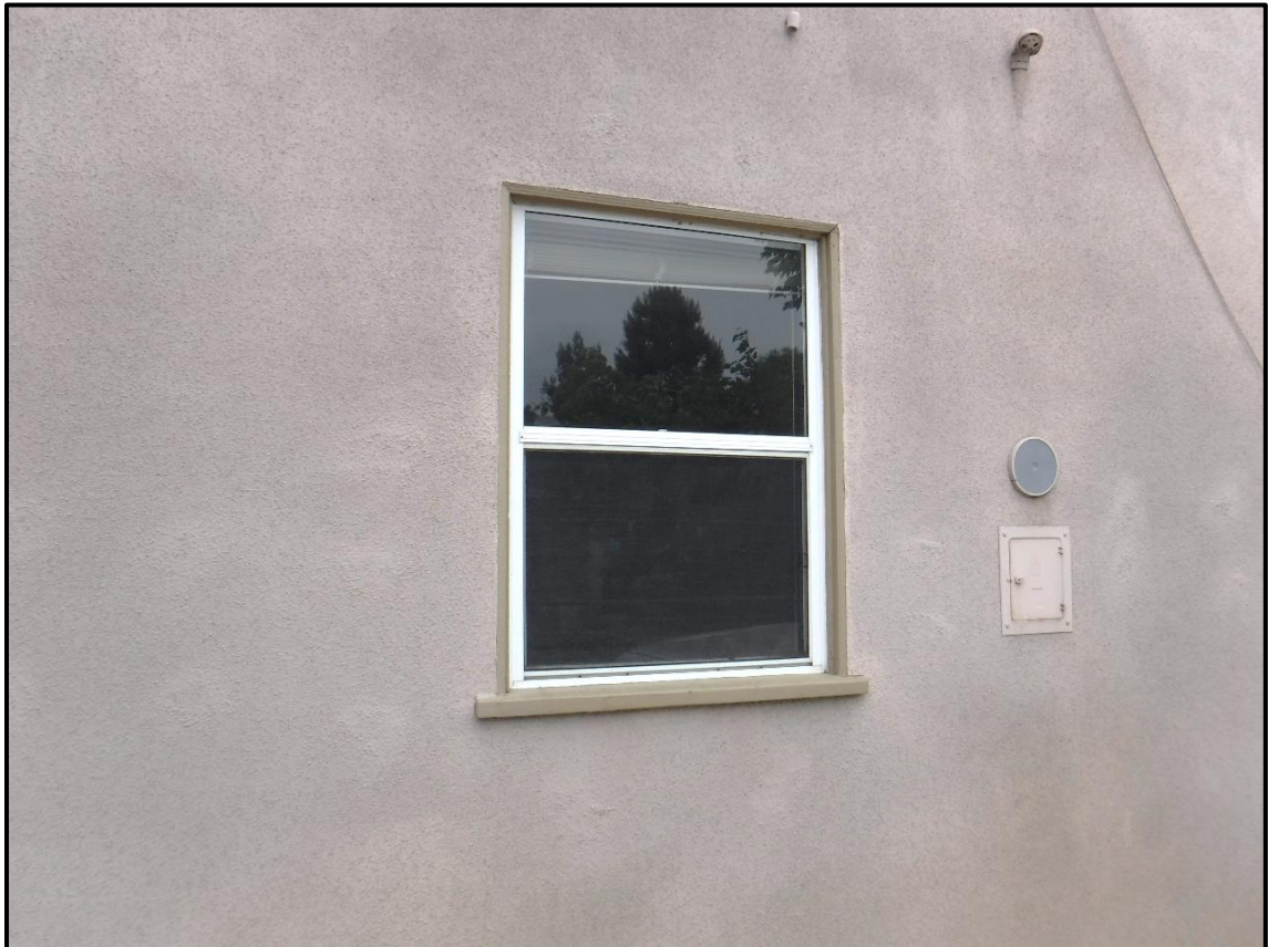
Window Detail, North Elevation, 1213 S. California Avenue, Monrovia, CA (SW)
