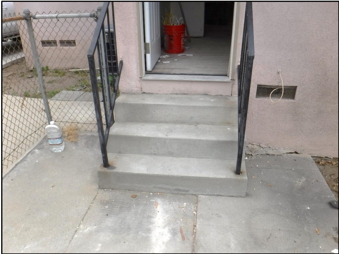
Rear Entry Stoop, West Elevation, 1213 S. California Avenue, Monrovia, CA (E)
