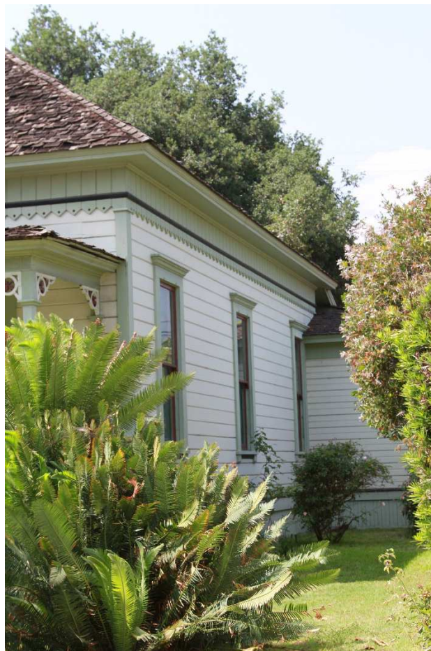
East side of house
