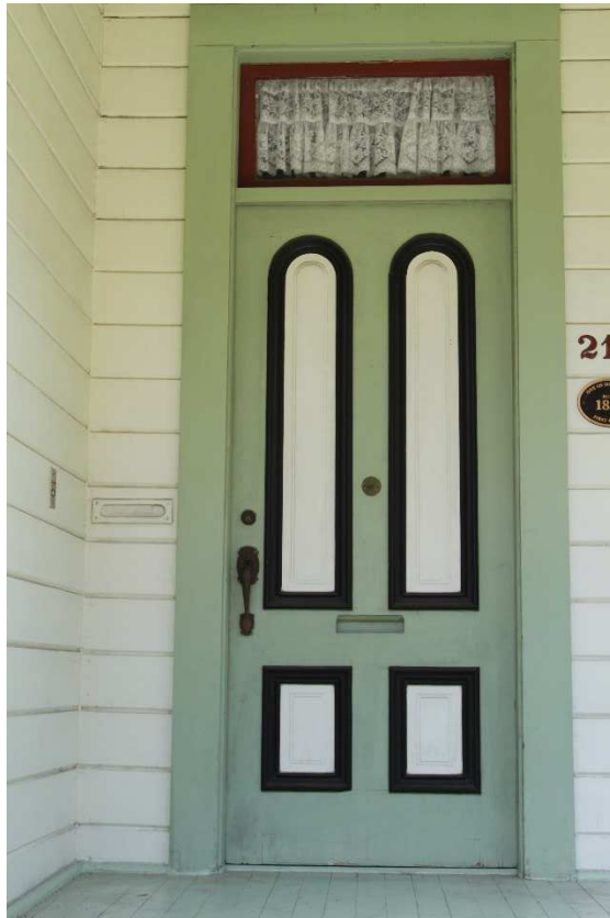
Front door with transom
