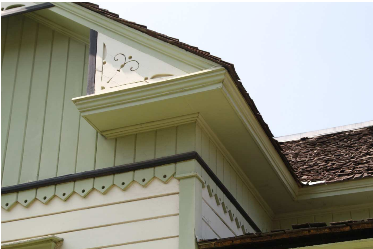
Detail of perforated pickets near roof line
