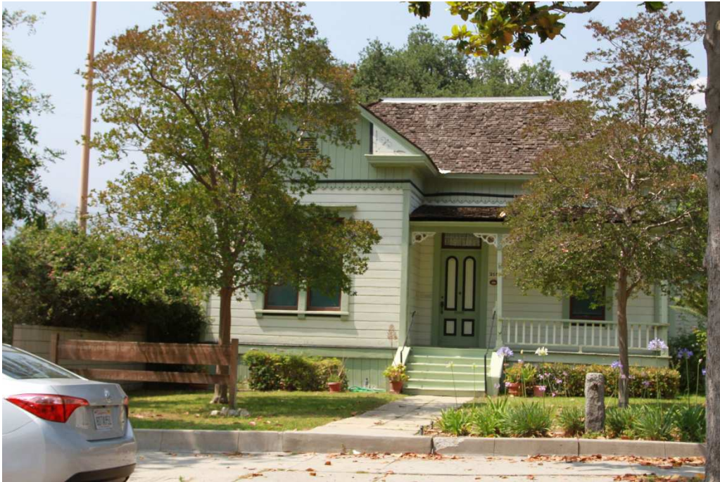
Front Façade --Looking North
