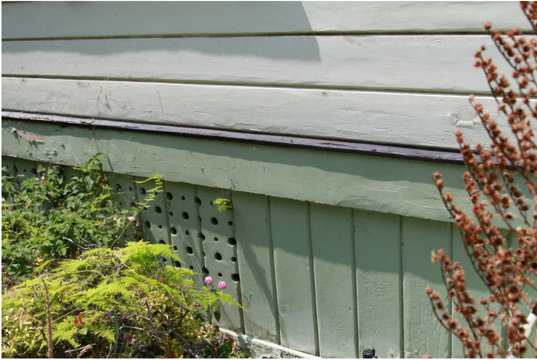
Vent holes in foundation skirting
