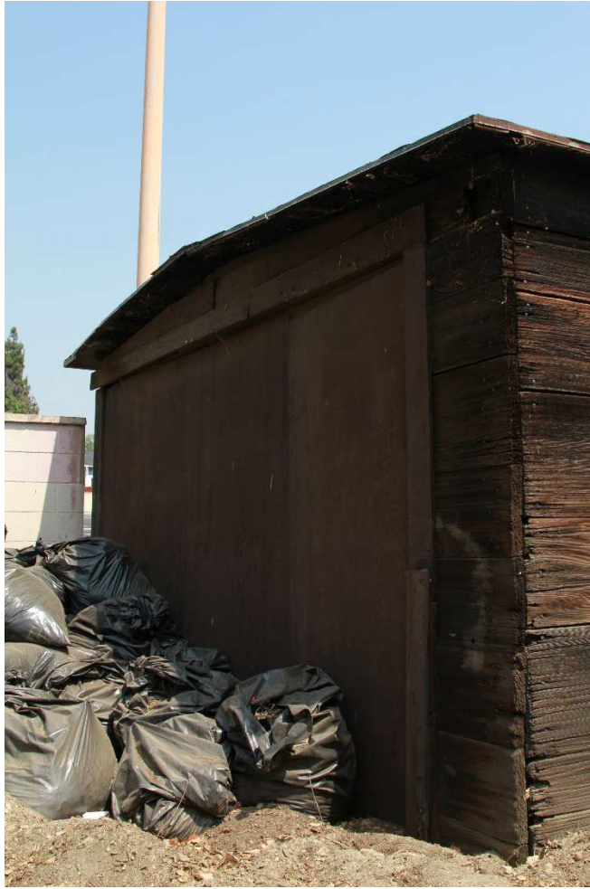
North side of older portion
