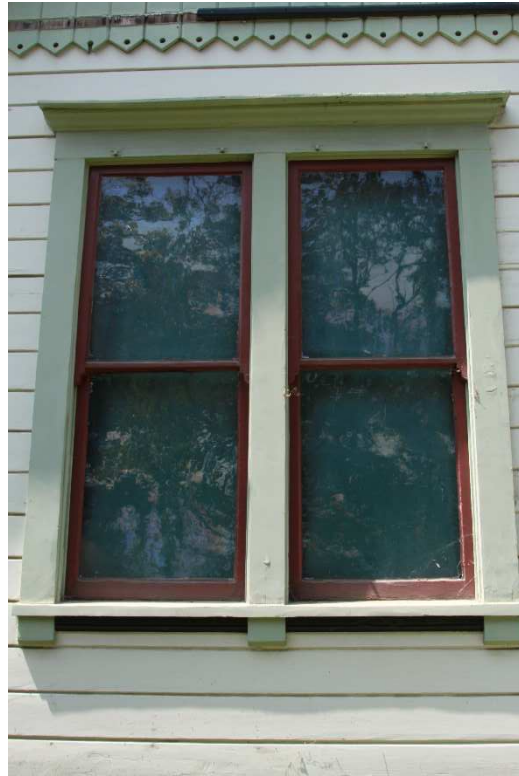
Double-hung windows with simple molding
