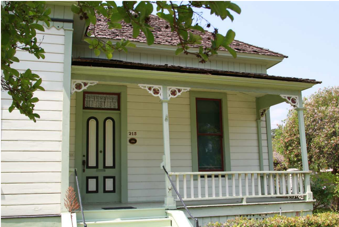
Covered Porch with simple railing
