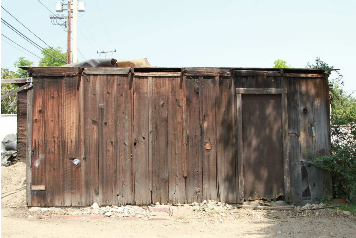
South side of "addition"
