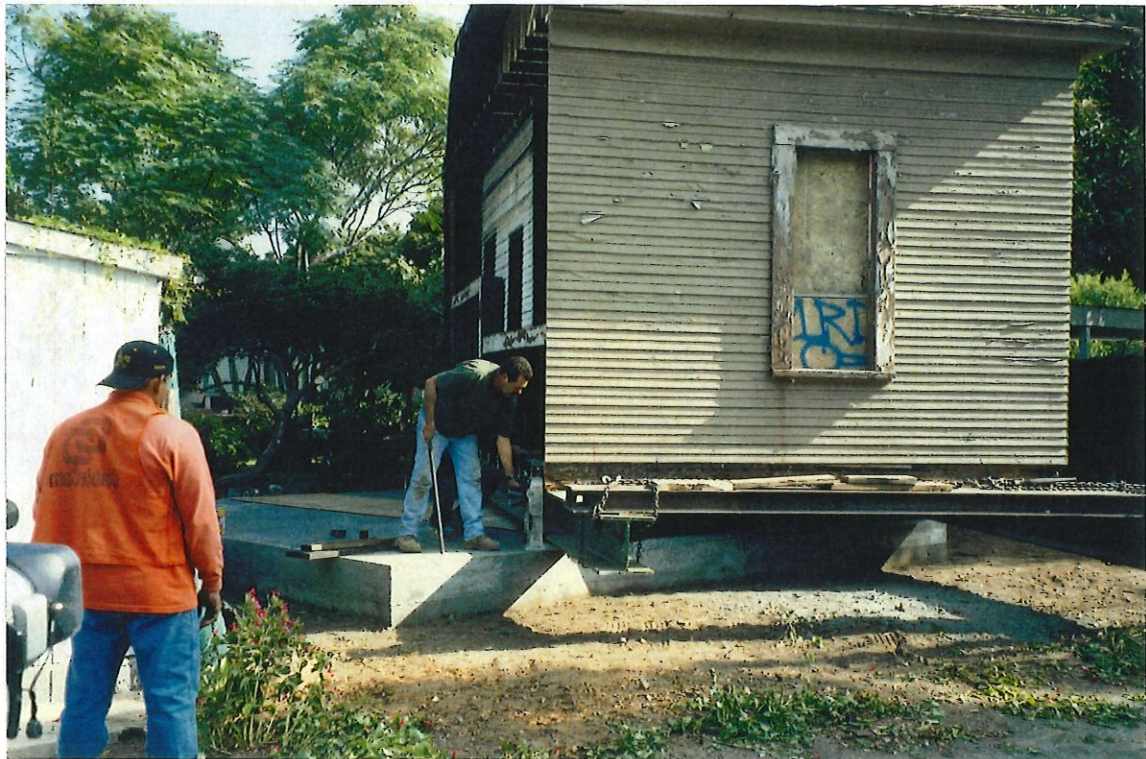
Moving the structure to new foundation.
