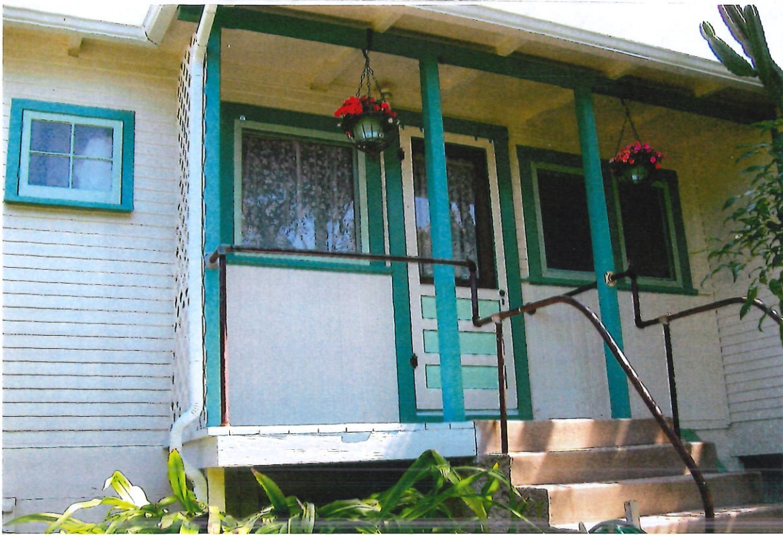
The back of the house after the renovation.
