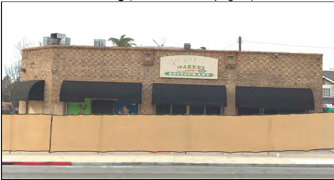
East elevation, view to the west (1/13/19)
