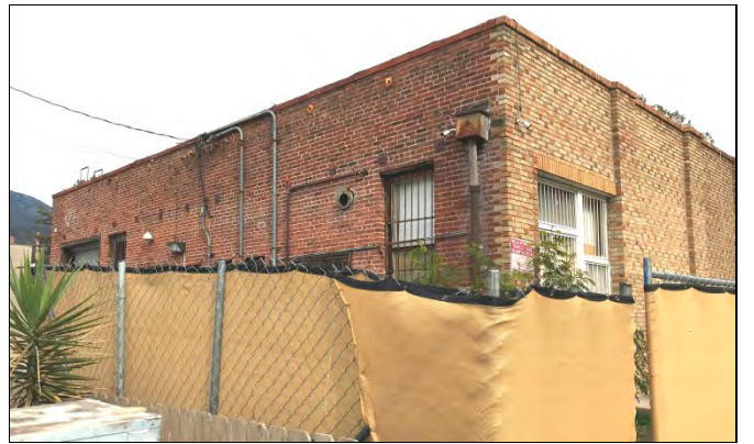
West elevation, view to the northeast (1/13/19)
