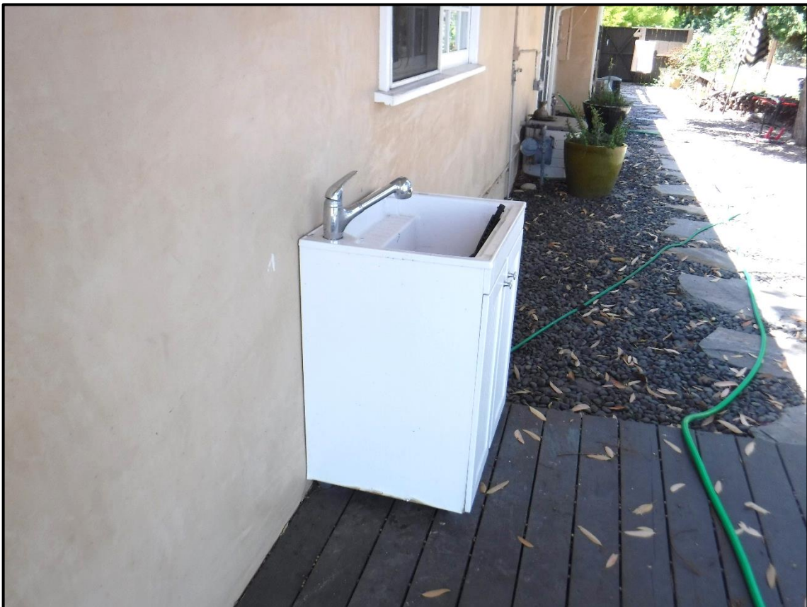
Outdoor Sink in East Elevation of Residence, 1104 Briarcliff Road, Monrovia (NNE)
