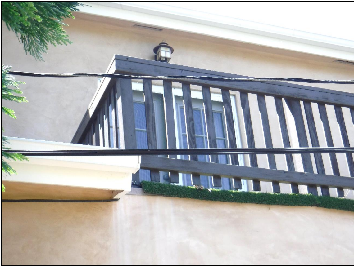
Balcony, Second Story Apartment above Garage, 1104 Briarcliff Road, Monrovia (WNW)
