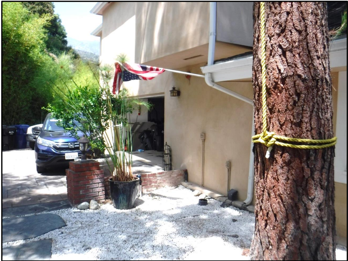
Overview to Attached Garage, 1104 Briarcliff Road, Arcadia (NE)
