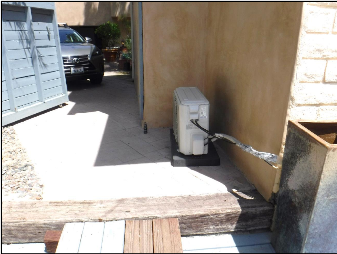
Based of 1970 Addition with A/C Unit, 1104 Briarcliff Road, Monrovia (NE)
