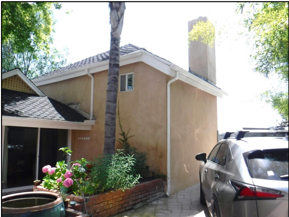
Addition to Residence, 1104 Briarcliff Road, Arcadia (ca. 1970; SW)
