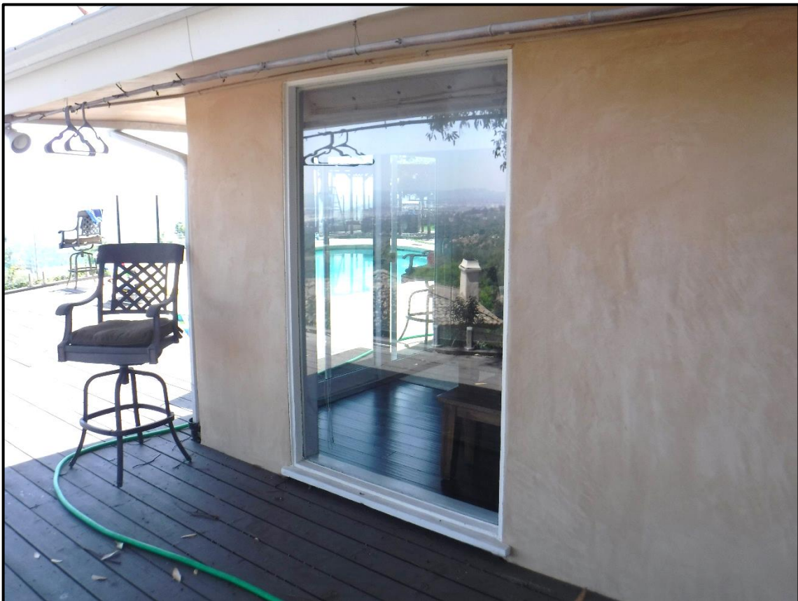
Fixed Window on East Elevation, 1104 Briarcliff Road, Monrovia (SSW)
