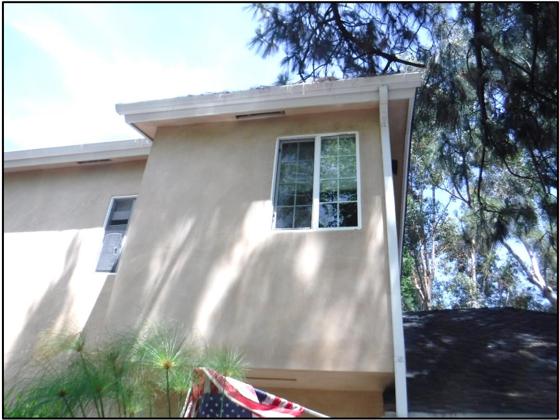
West Elevation of Apartment above Garage, 1104 Briarcliff Road, Arcadia (E)
