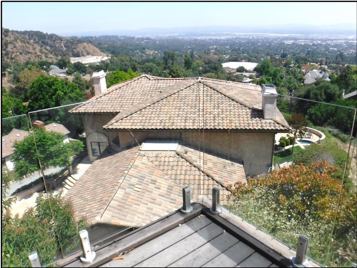
Overview from Rear Deck, 1104 Briarcliff Road, Monrovia (S)
