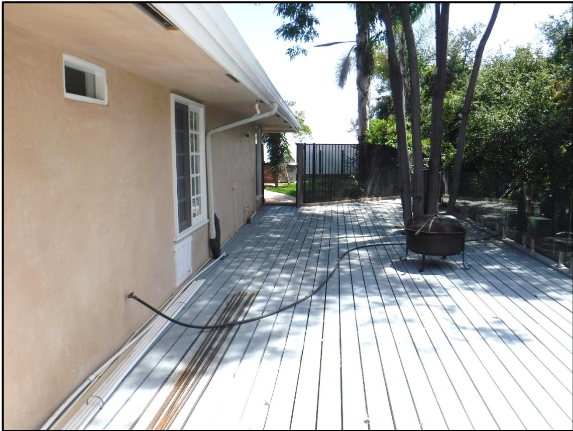
South Elevation along Rear Deck, 1104 Briarcliff Road, Monrovia (ENE)
