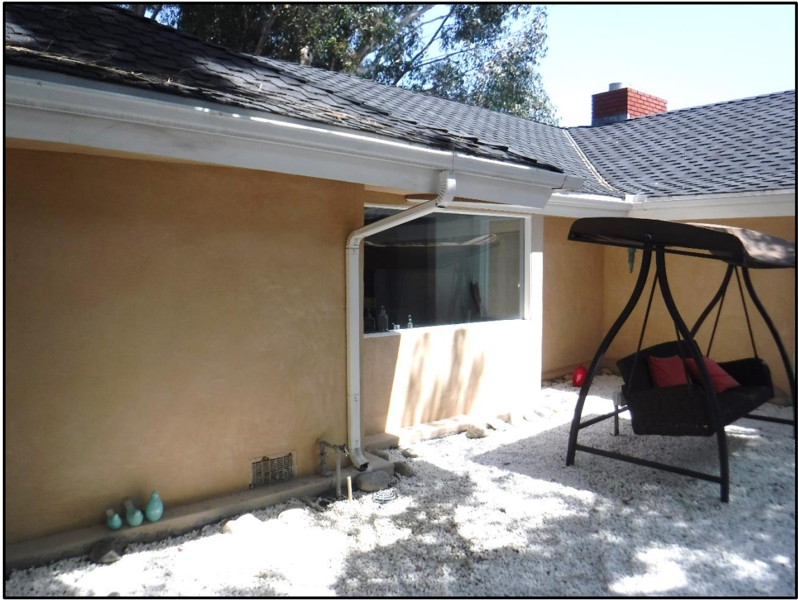
West Elevation of Residence, 1104 Briarcliff Road, Arcadia (SE)
