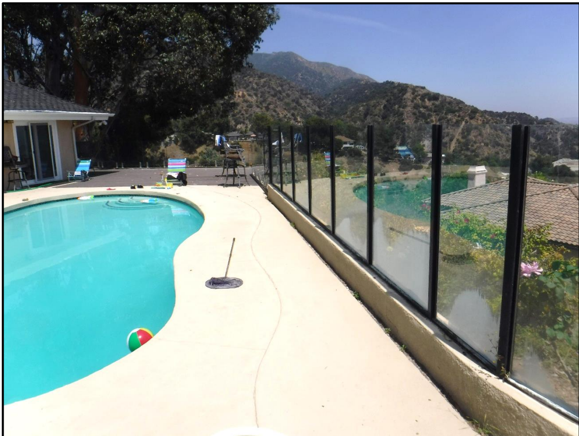
Overview of ca. 1967 Pool, 1104 Briarcliff Road, Monrovia (ENE)
