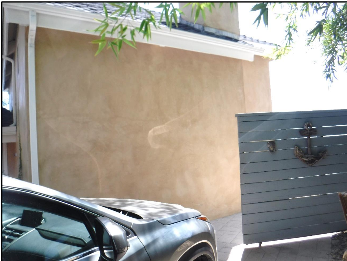
North Elevation of 1970 Addition, 1104 Briarcliff Road, Arcadia (ESE)
