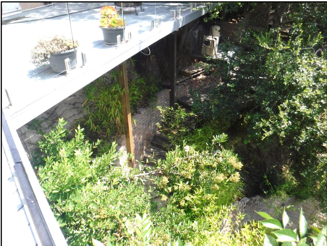
Support System for Rear Deck, 1104 Briarcliff Road, Monrovia (ENE)
