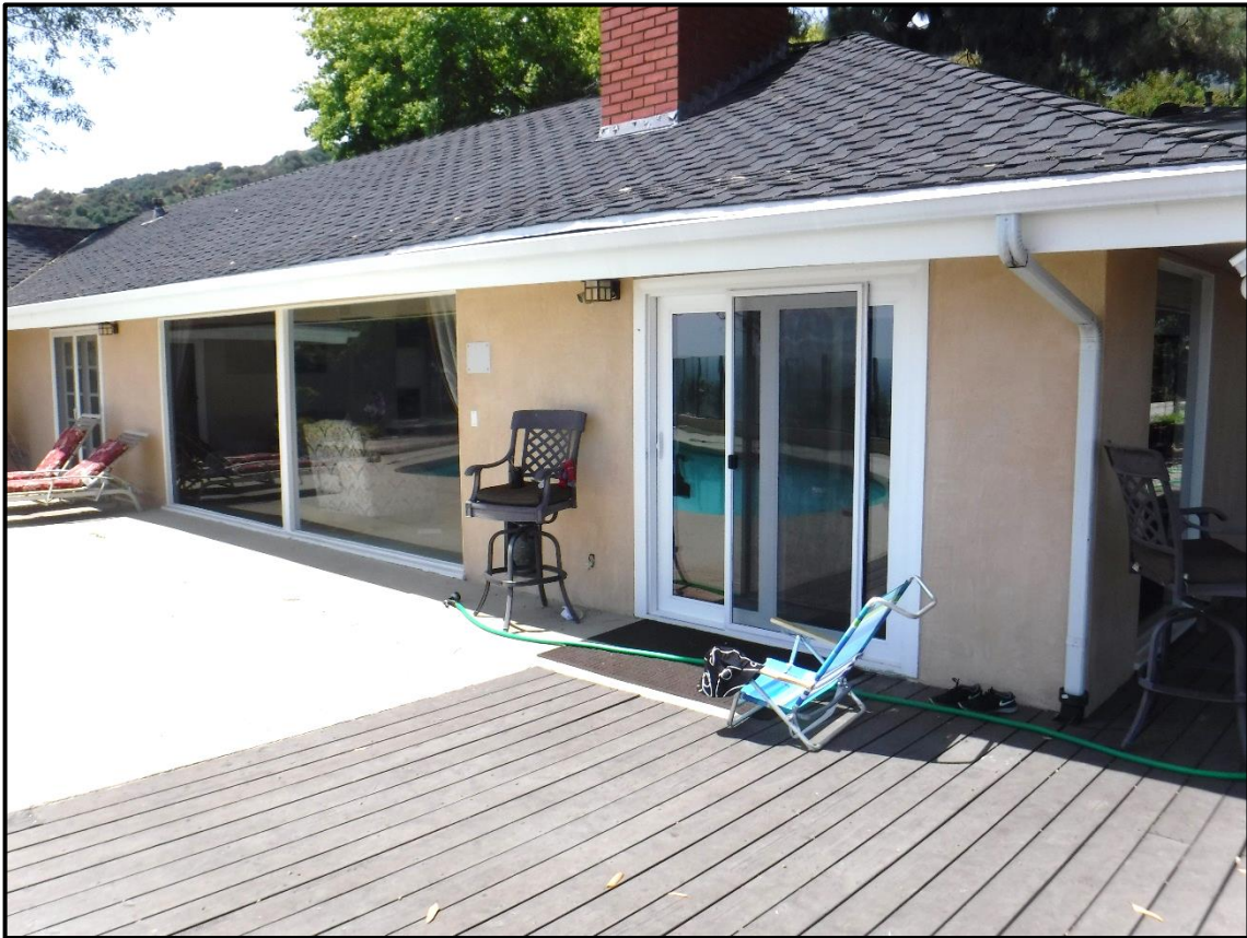
Overview of South Elevation of Residence, 1104 Briarcliff Road, Monrovia (NNW)
