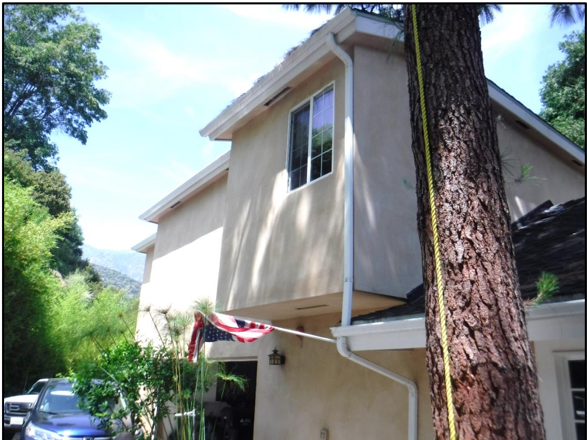
Attached Garage and Apartment, 1104 Briarcliff Road, Arcadia (NE)
