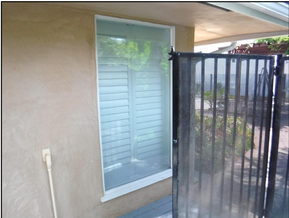
Window Detail, South Elevation, 1104 Briarcliff Road, Monrovia (ENE)
