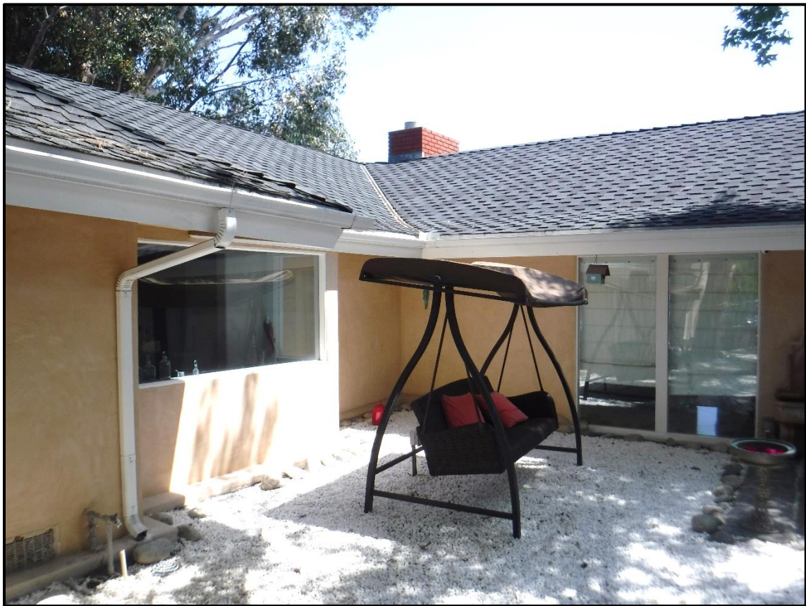
West and North Elevations of Residence, 1104 Briarcliff Road, Arcadia (SSE)
