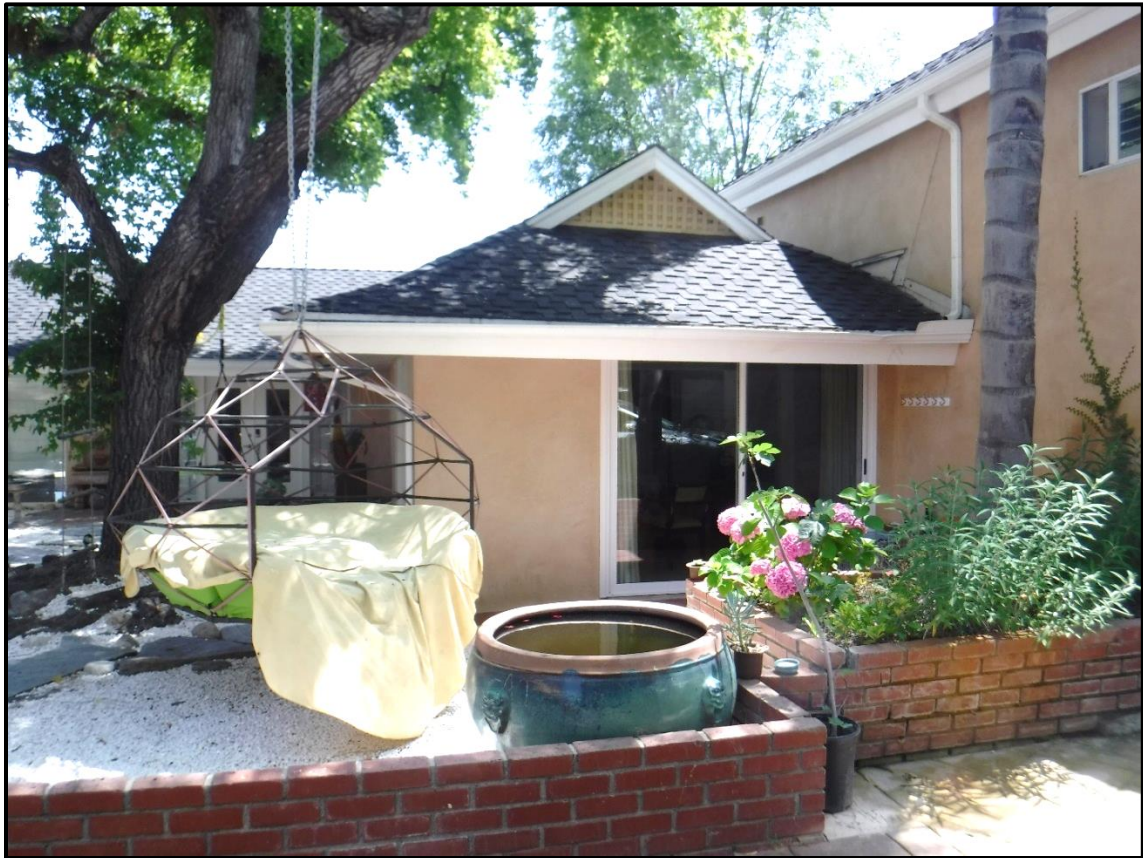
Original Construction, North Elevation, 1104 Briarcliff Road, Arcadia (SW)
