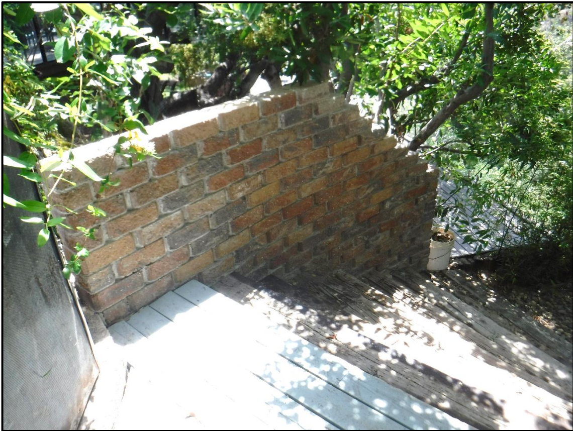
Stepped Entry to Southern Portion of Property, 1104 Briarcliff Road, Monrovia (W)
