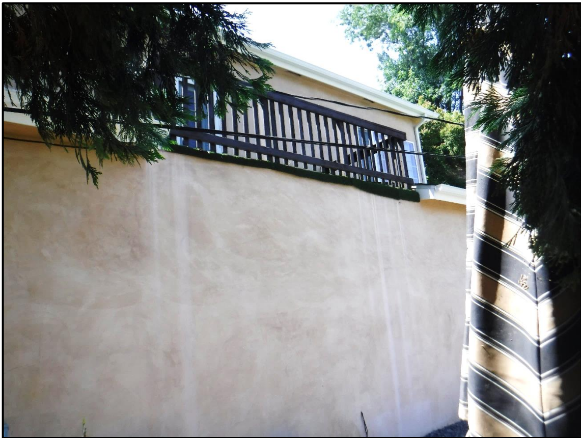
Apartment Balcony, East Elevation, 1104 Briarcliff Road, Monrovia (N)
