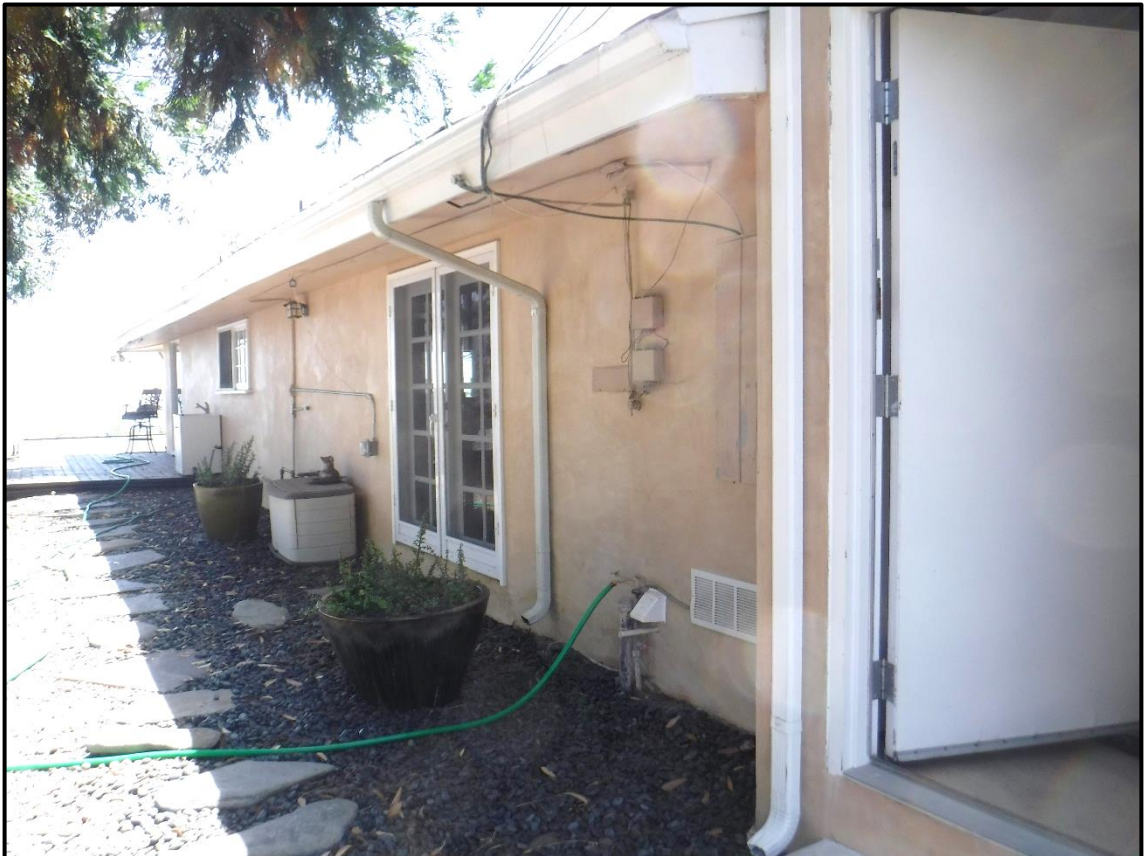
East Elevation of Residence, 1104 Briarcliff Road, Monrovia (SE)
