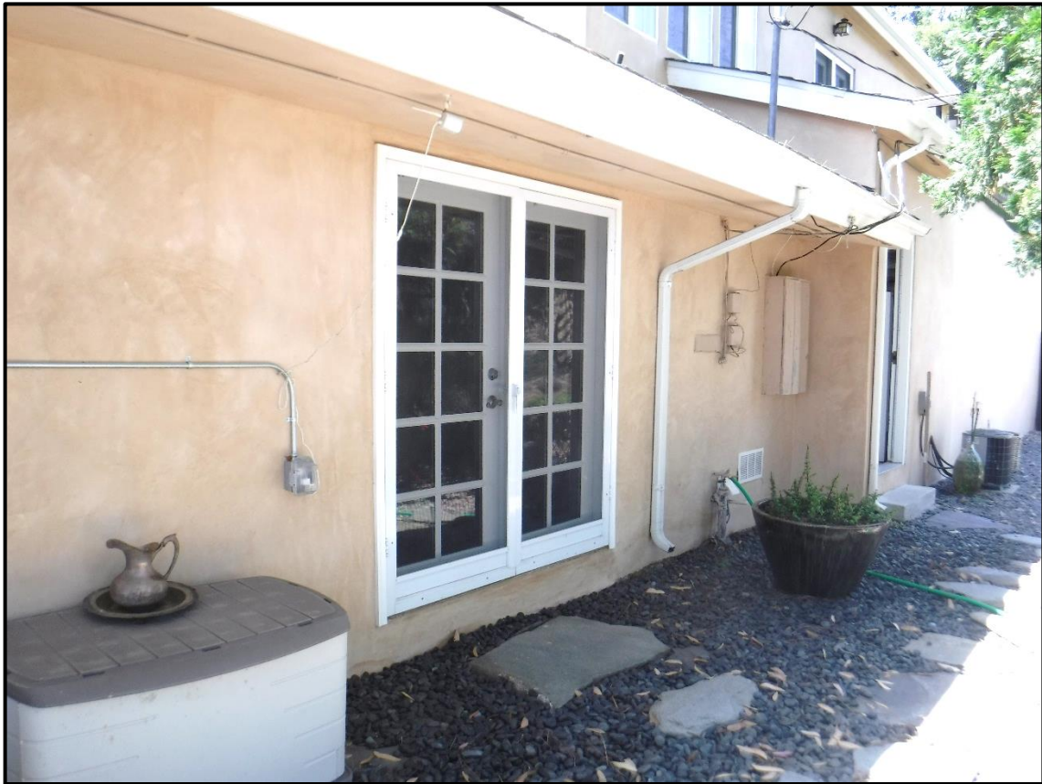
Doorway on East Elevation, 1104 Briarcliff Road, Monrovia (N)
