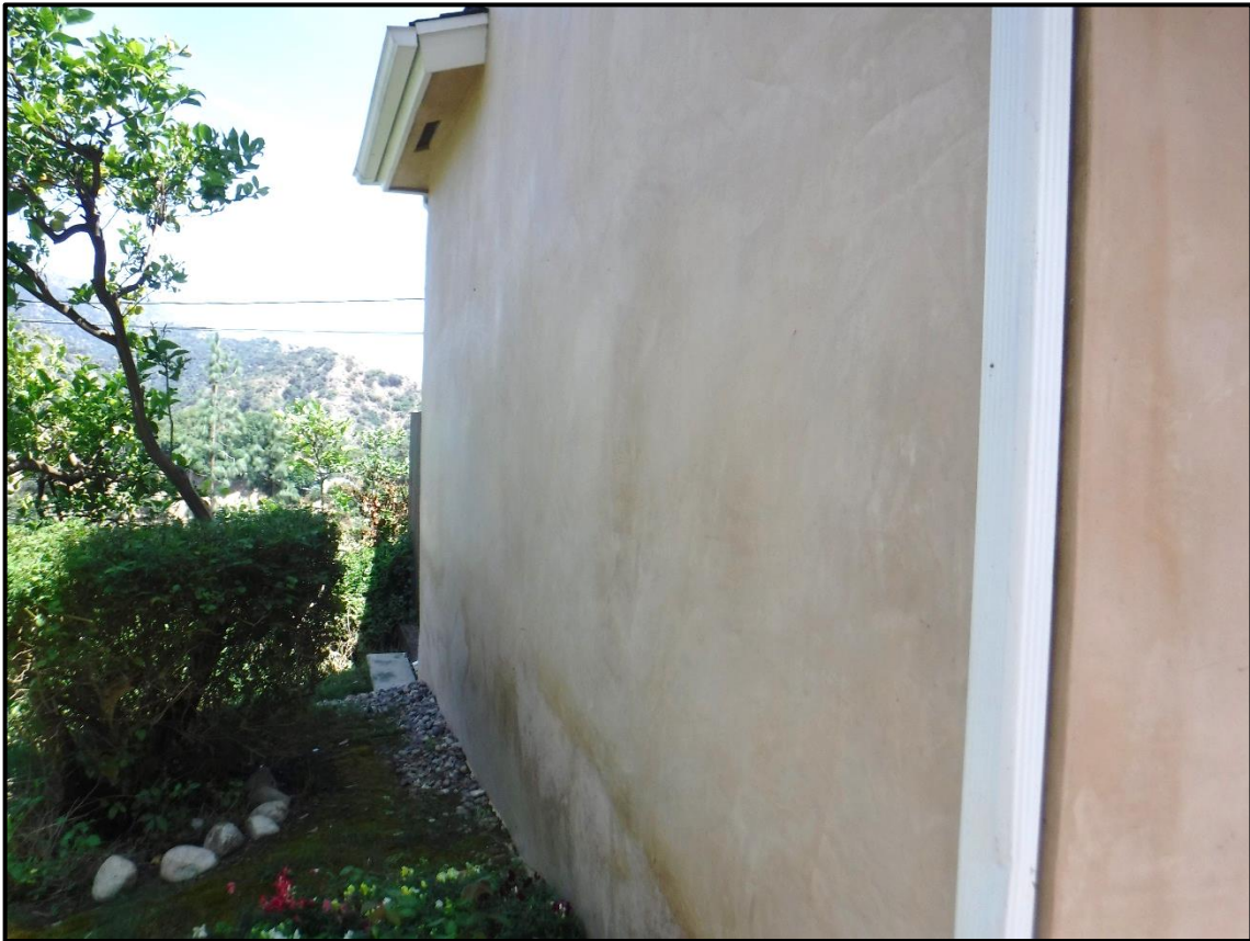
North Elevation of 2004 Garage, 1104 Briarcliff Road, Monrovia (ESE)
