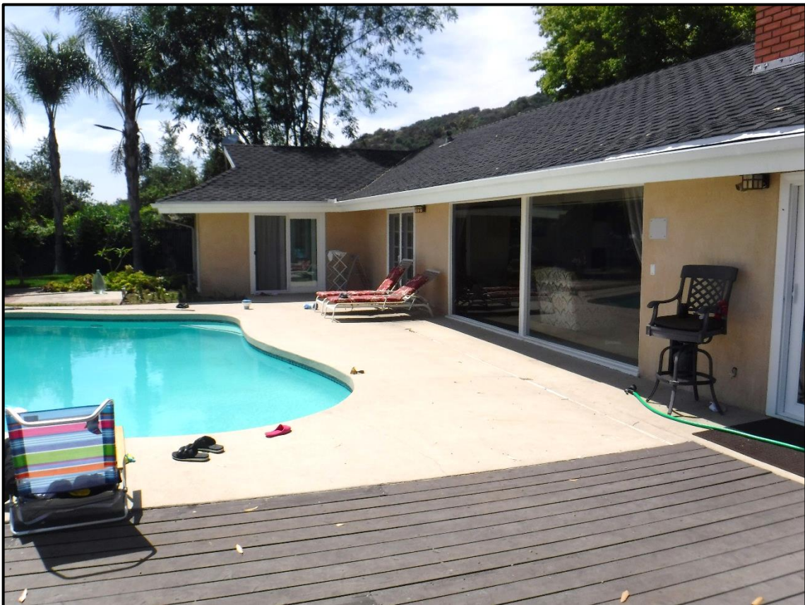
Overview of South Elevation of Residence, 1104 Briarcliff Road, Monrovia (NW)
