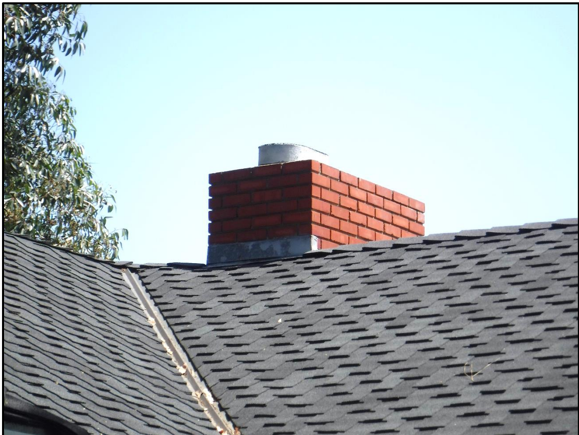
Original Brick Chimney, 1104 Briarcliff Road, Arcadia (SSE)
