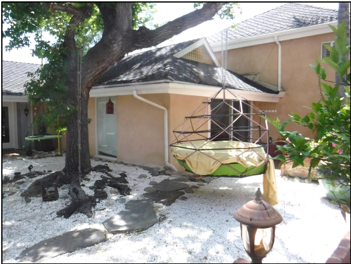
Original Construction and Addition, 1104 Briarcliff Road, Arcadia (SW)
