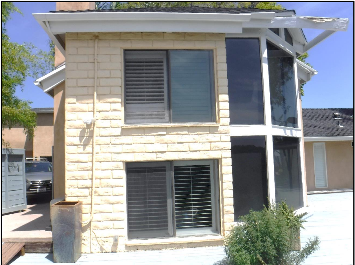
South Elevation of 1970 Addition, 1104 Briarcliff Road, Monrovia (NE)
