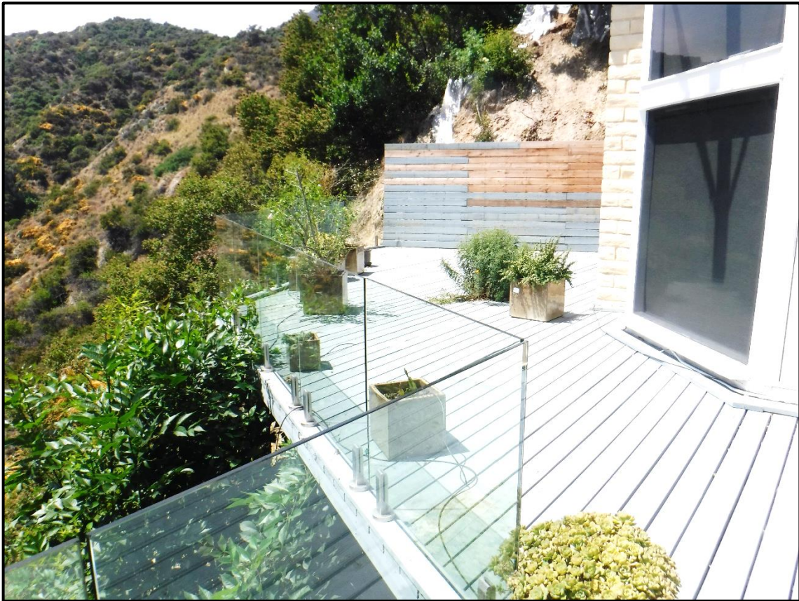
Overview of Rear Deck at 1970 Addition, 1104 Briarcliff Road, Monrovia (SW)
