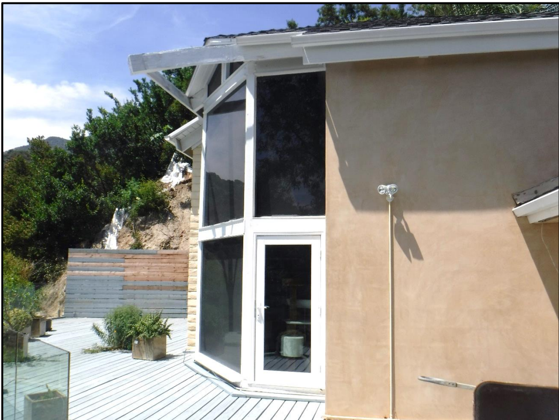
South and East Elevations of 1970 Addition, 1104 Briarcliff Road, Monrovia (WSW)
