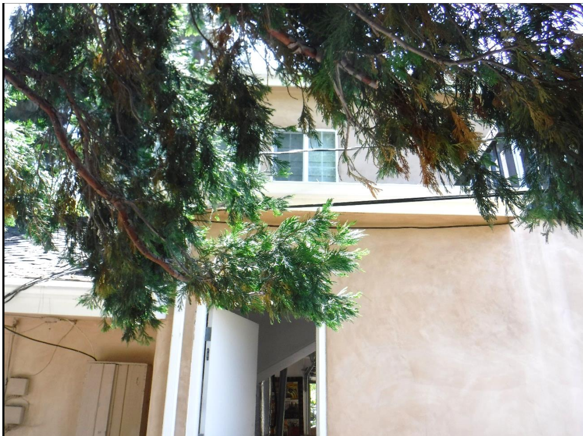
Second Story Apartment above Garage, East elevation, 1104 Briarcliff Road, Monrovia (WNW)
