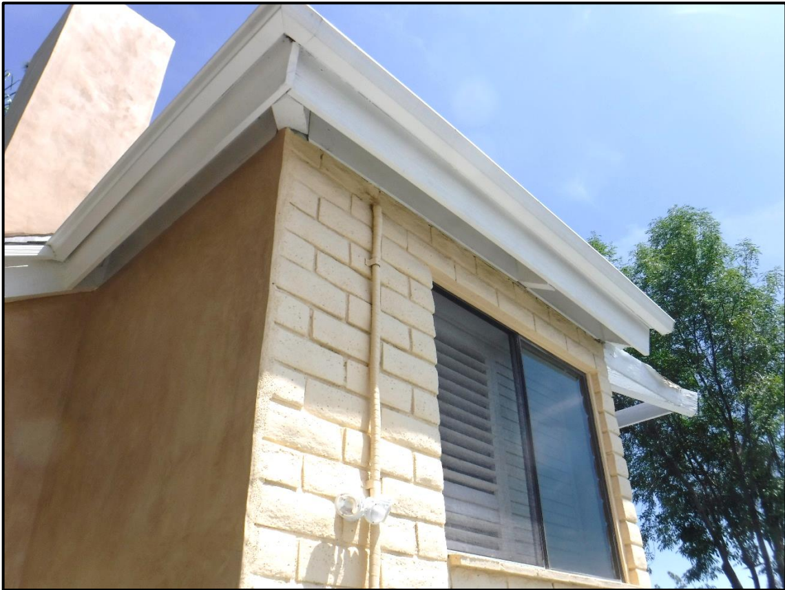
West and South Elevations of 1970 Addition, 1104 Briarcliff Road, Monrovia (N)
