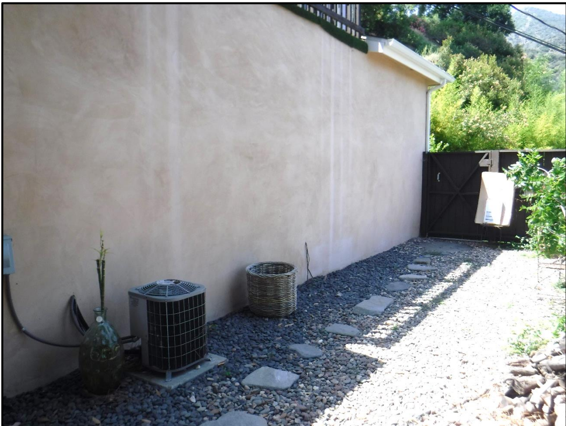
East Elevation of 2004 Garage, 1104 Briarcliff Road, Monrovia (NNE)
