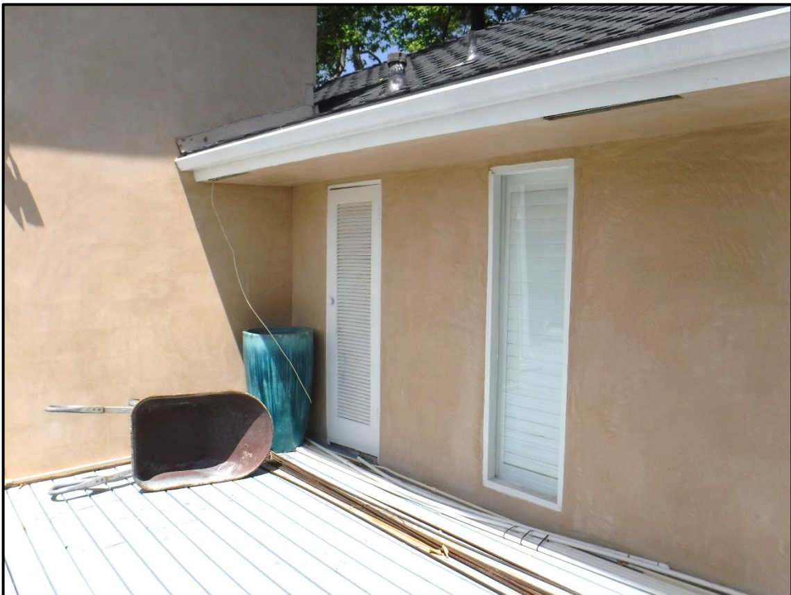
Interface with Original Residence and 1970 Addition, 1104 Briarcliff Road, Monrovia (NNW)
