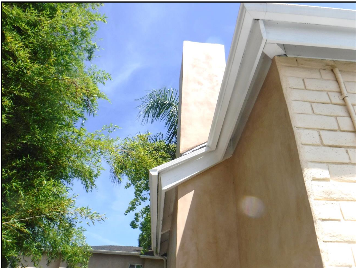
Chimney on 1970 Addition, 1104 Briarcliff Road, Monrovia (NE)
