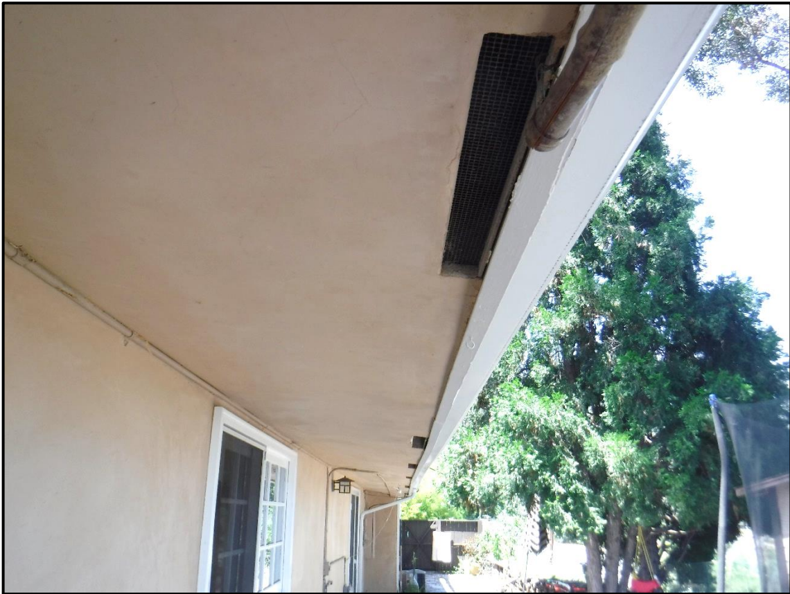
Eave along East Side of Residence, 1104 Briarcliff Road, Monrovia (NNE)
