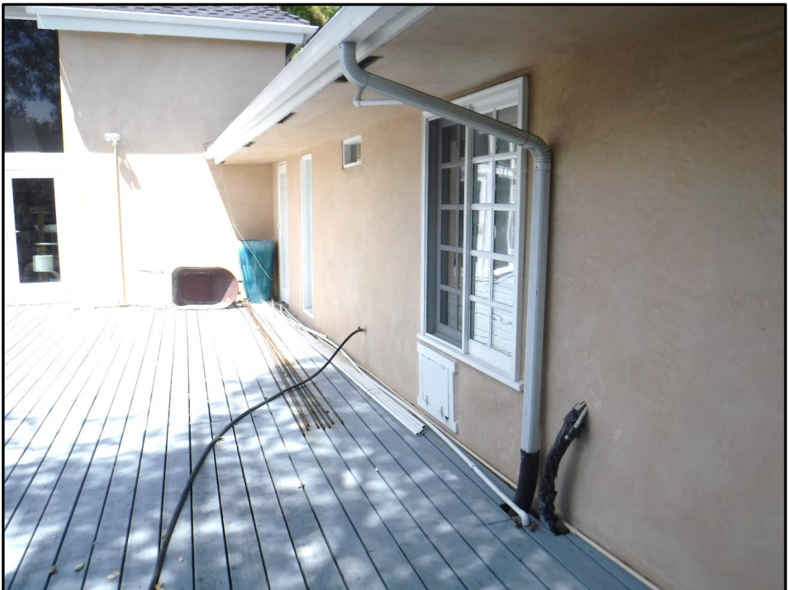
Overview of South Elevation, 1104 Briarcliff Road, Monrovia (SW)
