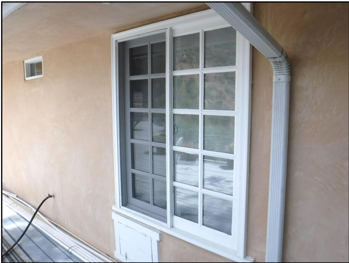
Window Detail, South Elevation, 1104 Briarcliff Road, Monrovia (N)
