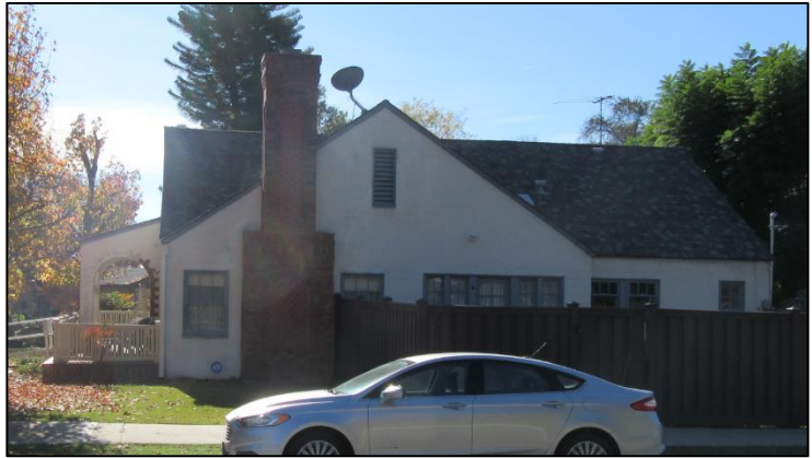
Figure 2. Photo of 307 Stedman Place as seen from Greystone Avenue.
