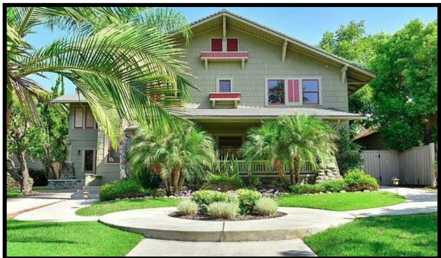
Figure 1. View of the front (south) elevation of Landmark No. 116. The project will build an outdoor kitchen in the backyard.
