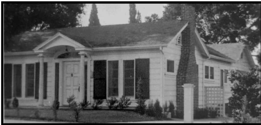
Figure 2. Front elevation of the American Colonial Revival home at 234 West Greystone Avenue from 1923. The original porch columns and brick chimney can be seen.
