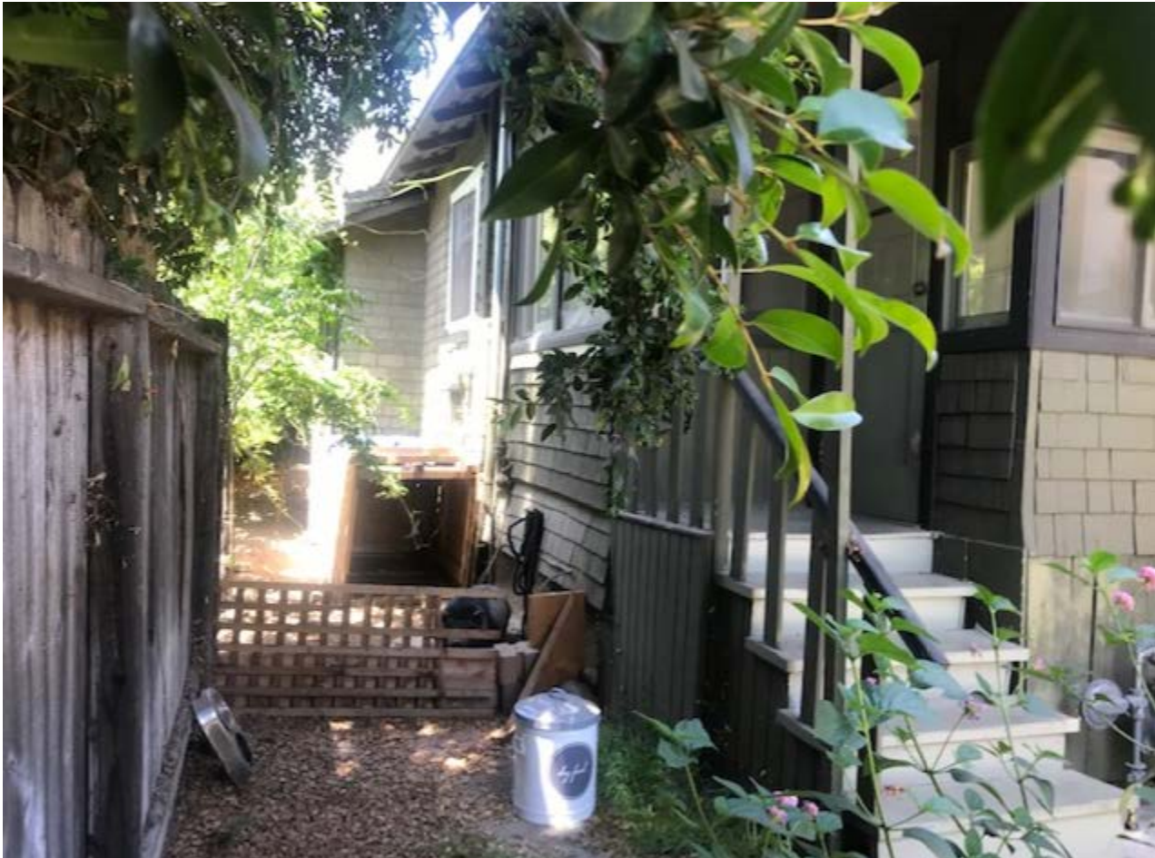
Partial View of West (Side) Elevation - View Looking North
