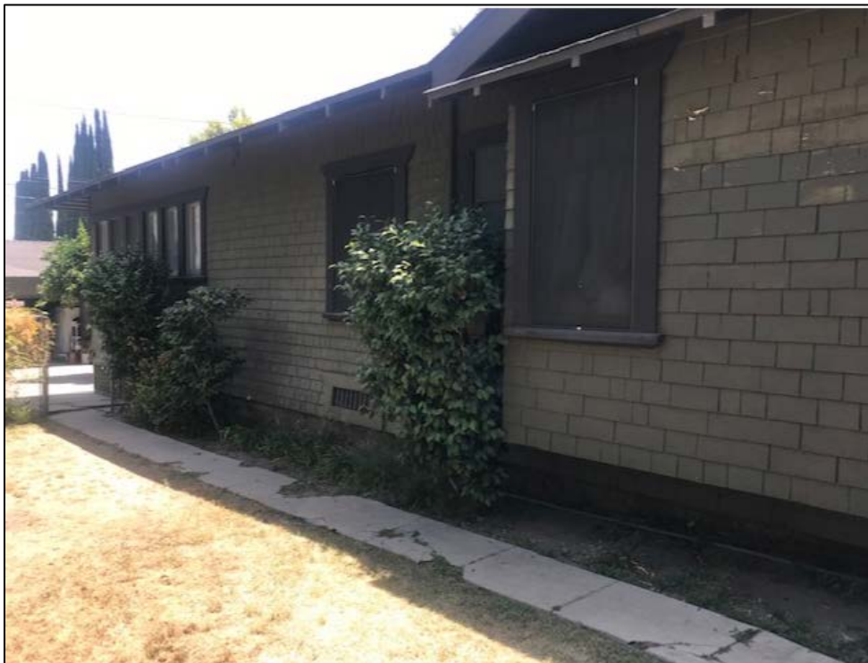
East (Side) Elevation (View Looking Southwest)
