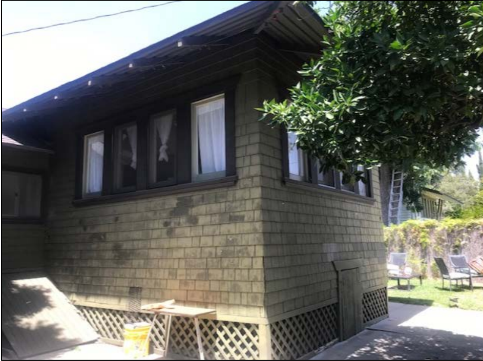
South (Rear) Elevation (1912 Sleeping Porch Addition - View Looking Northeast)
