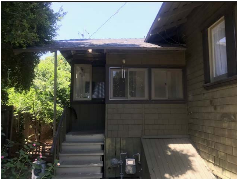
South (Rear) Elevation (Back porch - View Looking North)
