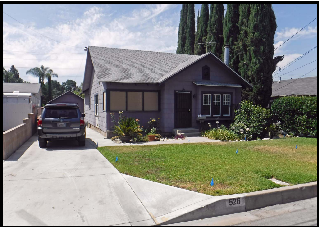
Residence at 526 W. Walnut Avenue, Monrovia, CA (1923; SSW)
