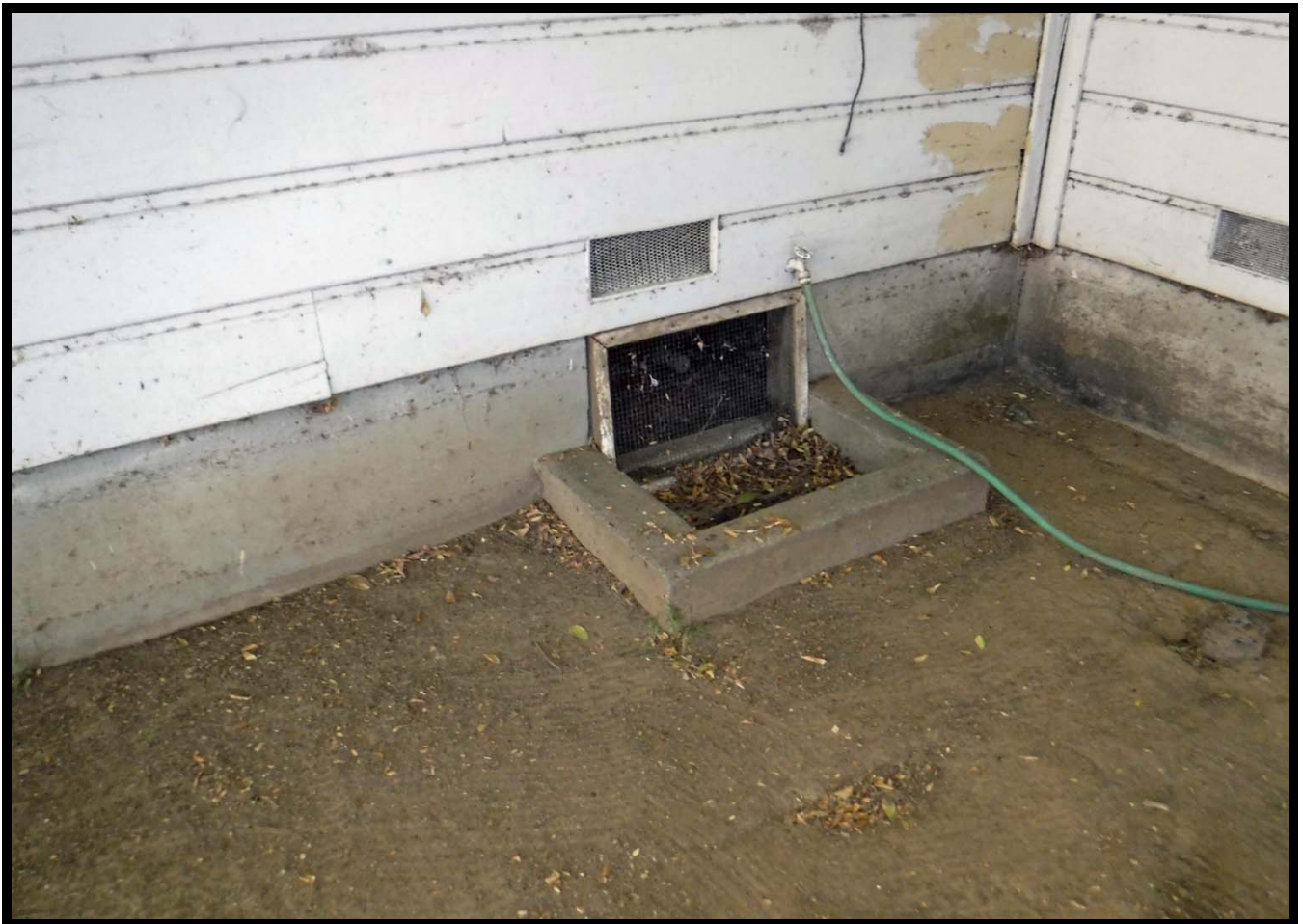
Crawl Space, West Elevation, 610 W. Walnut Avenue, Monrovia, CA (SE)
