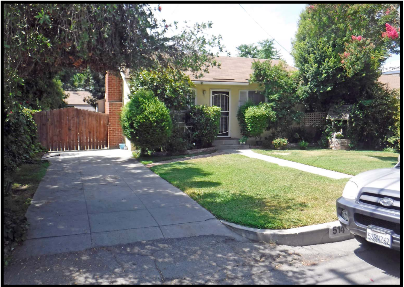
Residence at 514 W. Walnut Avenue, Monrovia, CA (1939-1966; SSW)
