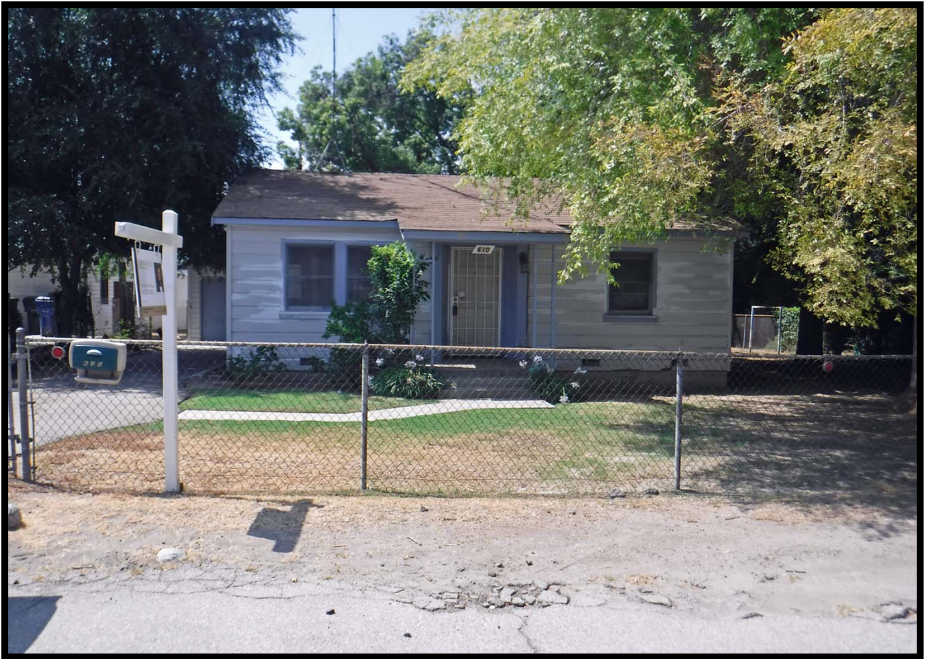
North Elevation of 610 W. Walnut Avenue, Monrovia, CA (S)
