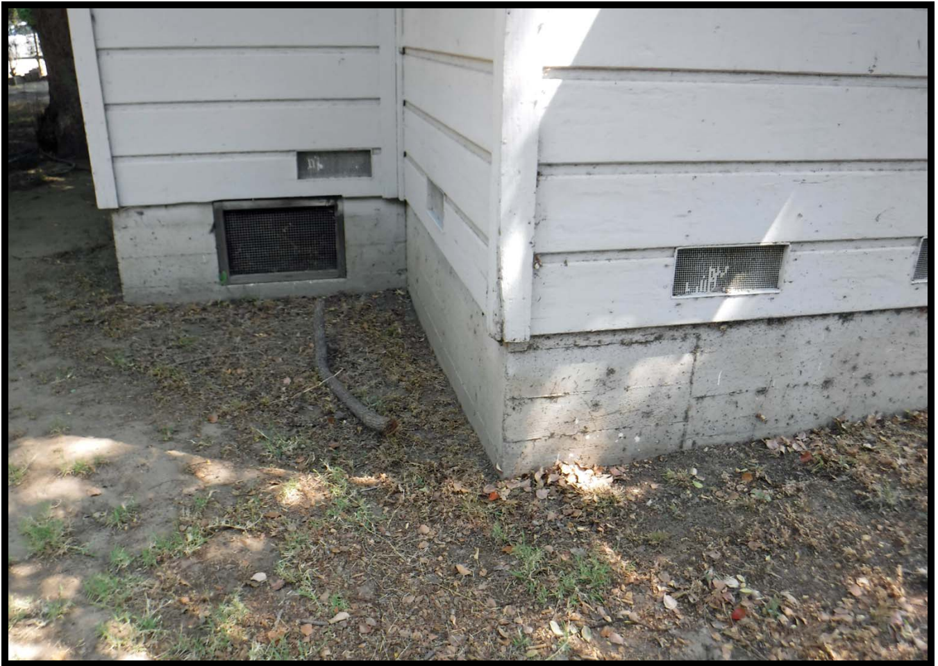
Foundation on South Elevation, 610 W. Walnut Avenue, Monrovia, CA (N)
