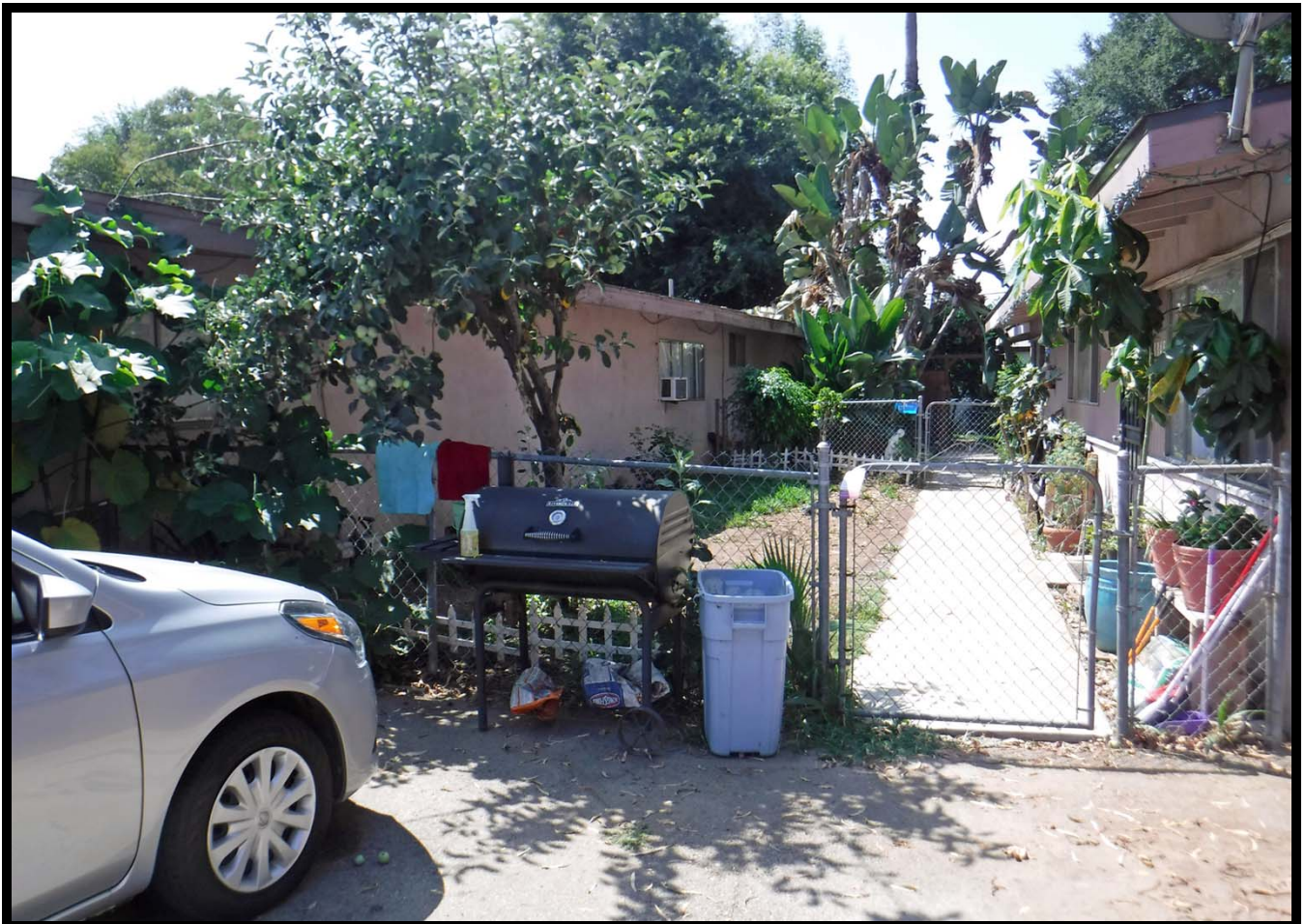
Courtyard at Units F & G and West Elevation of 634 W. Olive Avenue, Units D & E, Monrovia, CA (1965; S)
