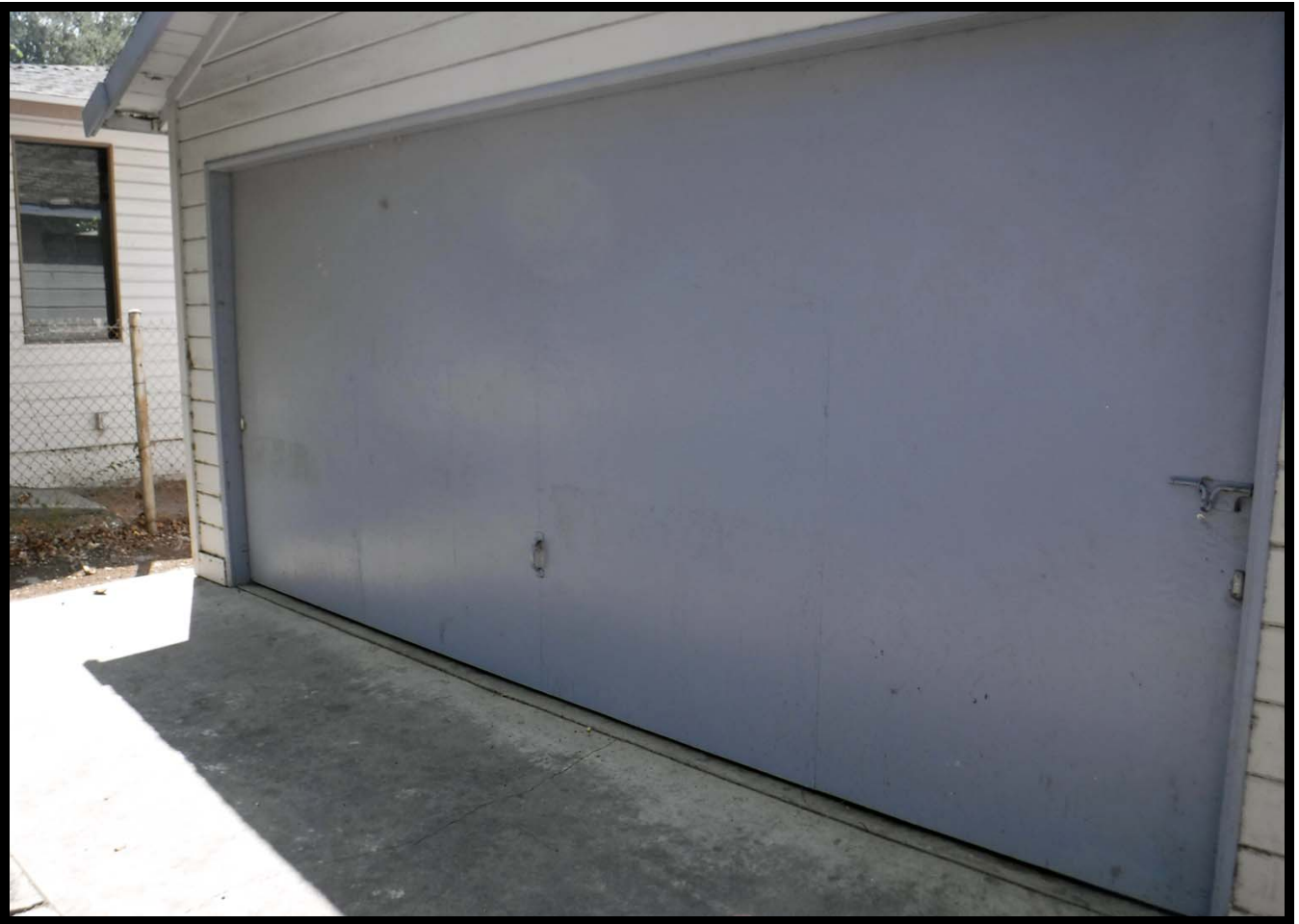
Garage Bay Door, 610 W. Walnut Avenue, Monrovia, CA (ESE)
