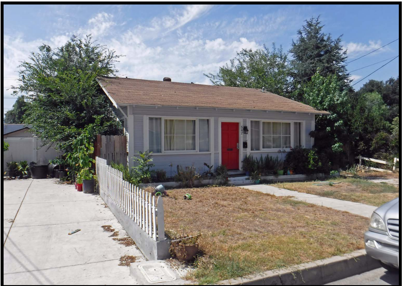
Residence at 542 W. Walnut Avenue, Monrovia, CA (1924-1937; SSW)
