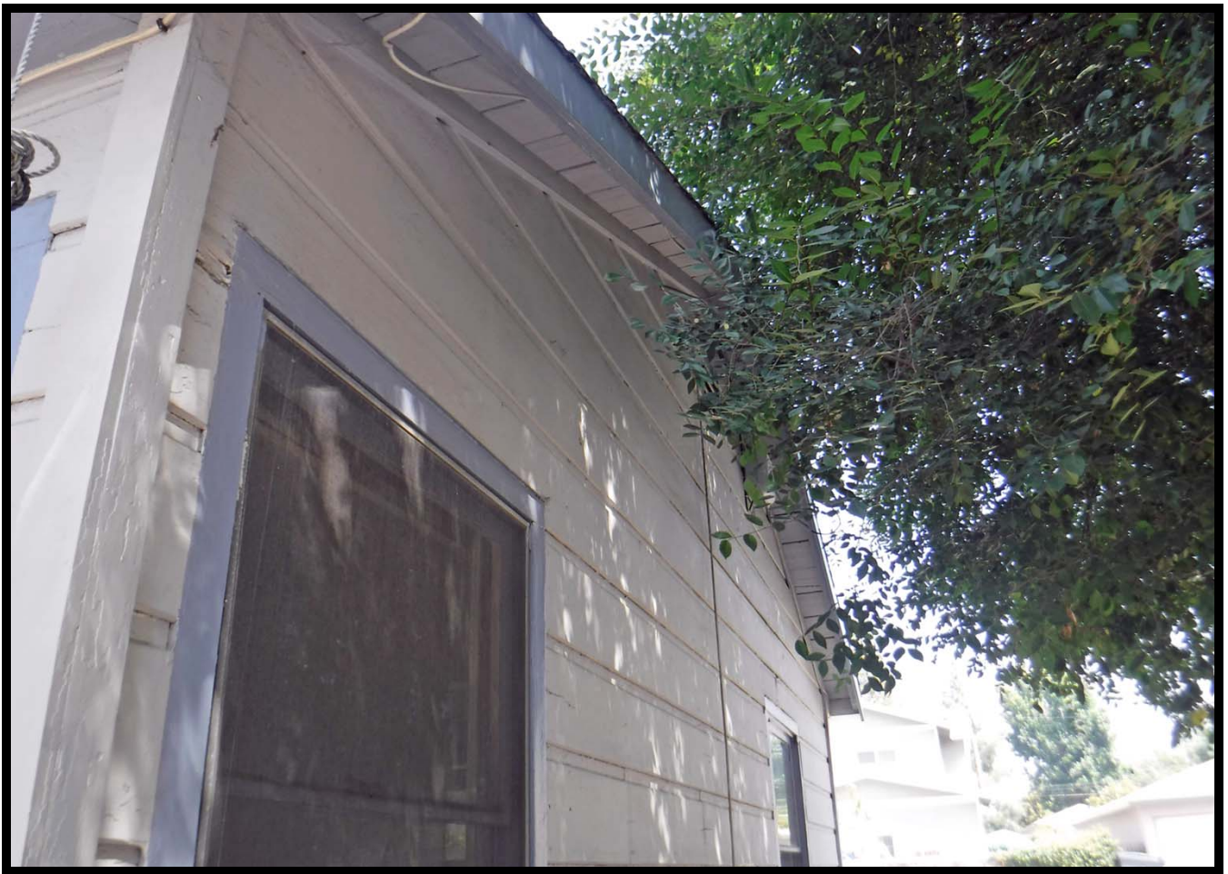
East Elevation, 610 W. Walnut Avenue, Monrovia, CA (NW)
