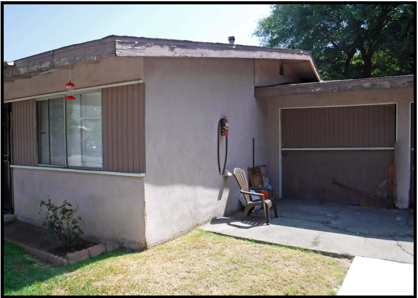
Garage and South Elevation of 634 W. Olive Avenue, Unit B, Monrovia, CA (1965; ENE)
