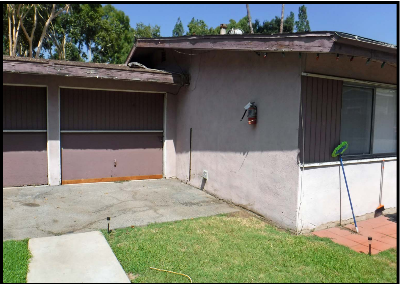
South Elevation of 634 W. Olive Avenue, Unit D, Monrovia, CA (1965; WNW)
