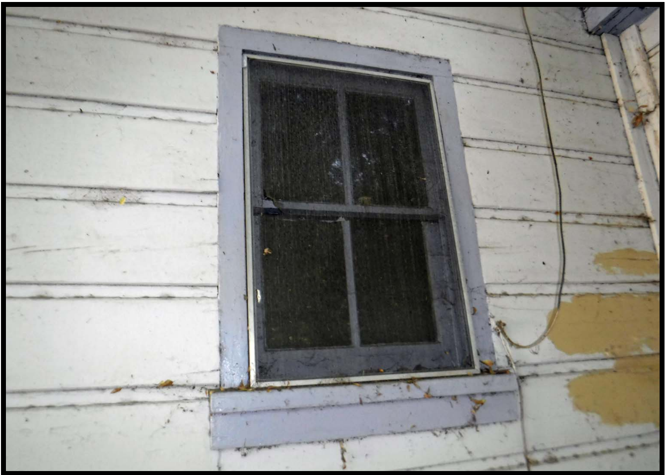
Window Detail, West Elevation, 610 W. Walnut Avenue, Monrovia, CA (ESE)
