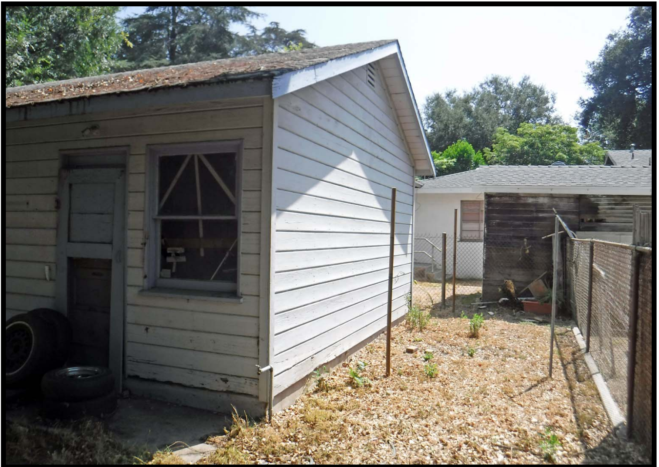
South Elevation of Garage, 610 W. Walnut Avenue, Monrovia, CA (ENE)
