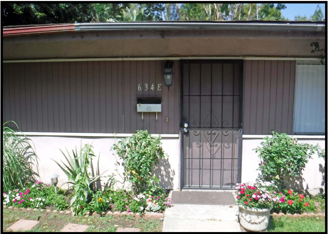
East Elevation of 634 W. Olive Avenue, Unit E, Monrovia, CA (1965; W)
