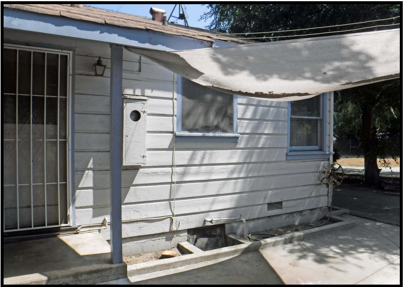
South Elevation, 610 W. Walnut Avenue, Monrovia, CA (NE)
