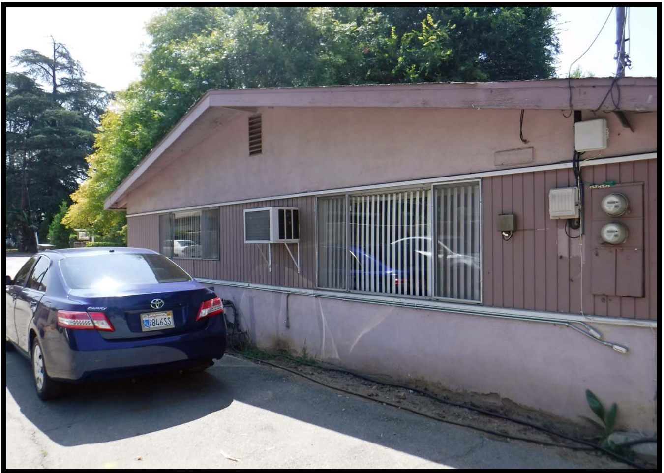
North Elevation of 634 W. Olive Avenue, Unit B, Monrovia, CA (1965; ESE)
