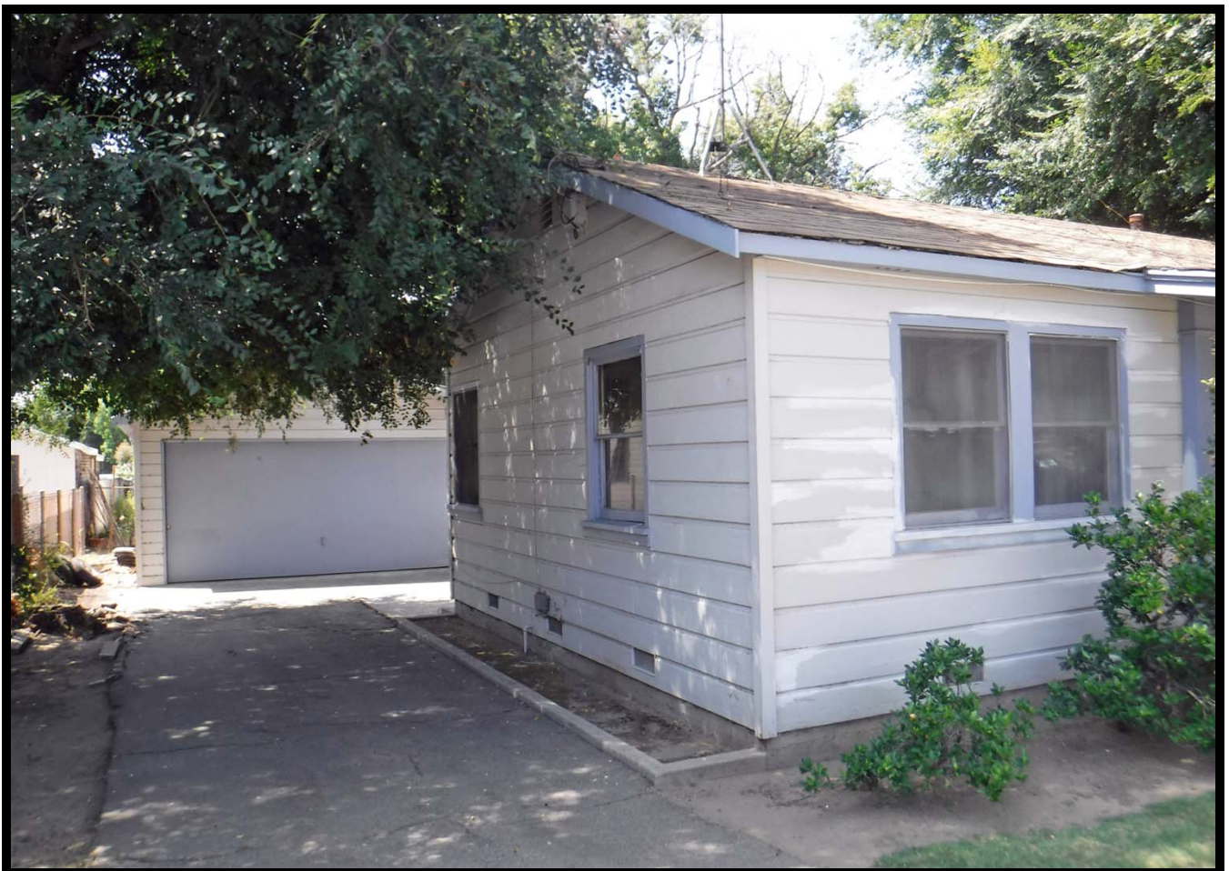
East and North Elevations, 610 W. Walnut Avenue, Monrovia, CA (SSW)
