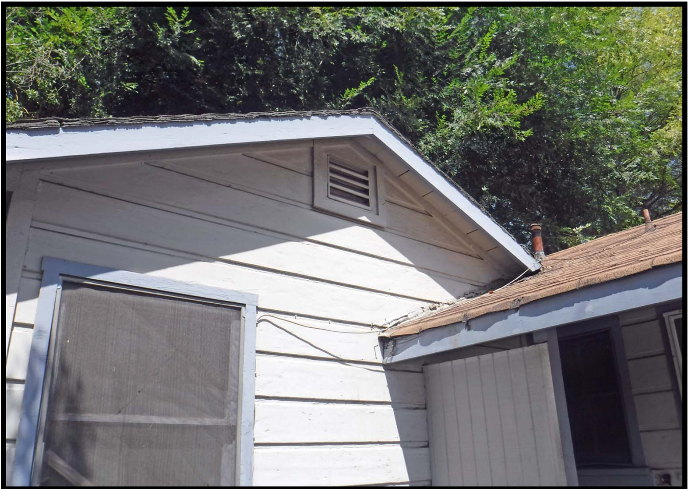
Part of East Elevation, 610 W. Walnut Avenue, Monrovia, CA (NW)
