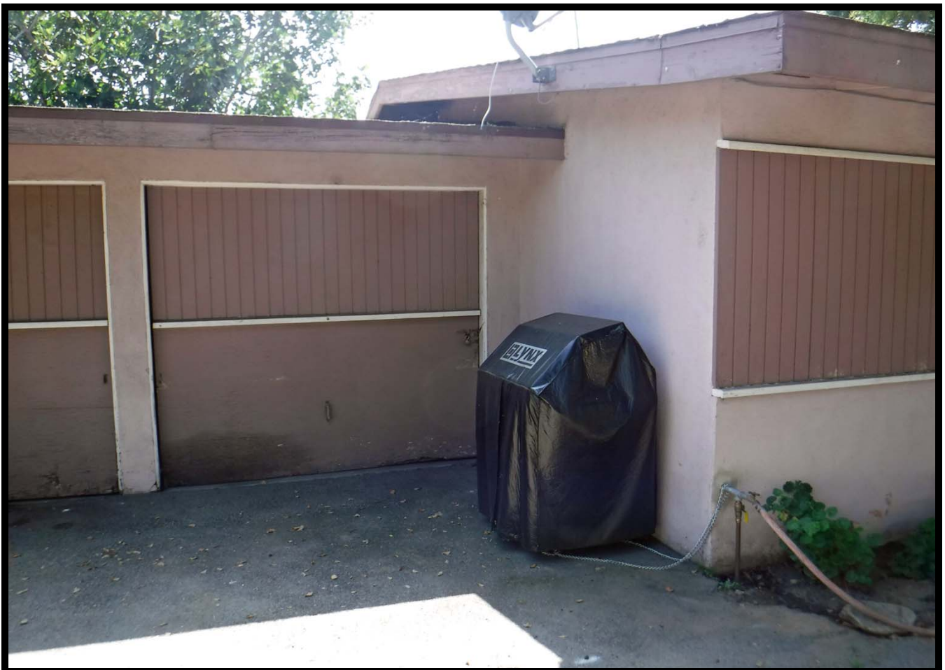
Garage at 634 W. Olive Avenue, Unit A, Monrovia, CA (ESE)
