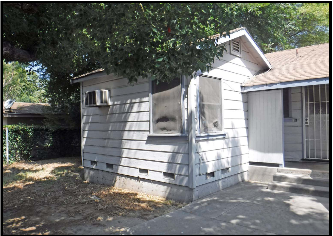
South Elevation, 610 W. Walnut Avenue, Monrovia, CA (NW)
