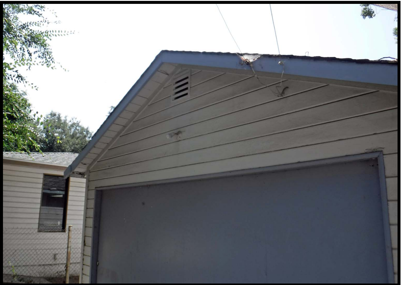
Roofline of Garage, North Elevation, 610 W. Walnut Avenue, Monrovia, CA (SE)
