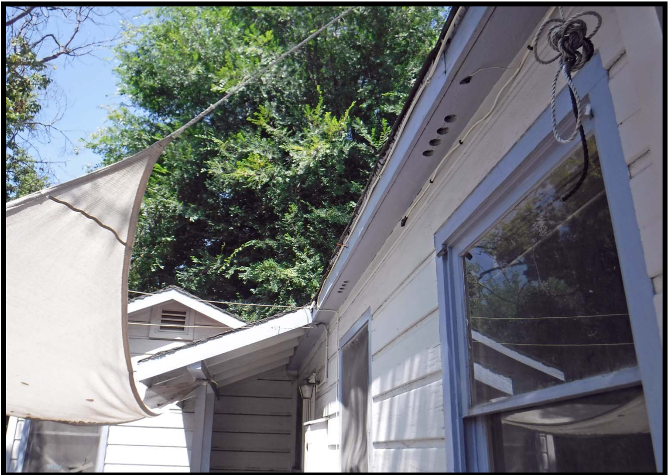
Shallow Eave of South Elevation, 610 W. Walnut Avenue, Monrovia, CA (WNW)
