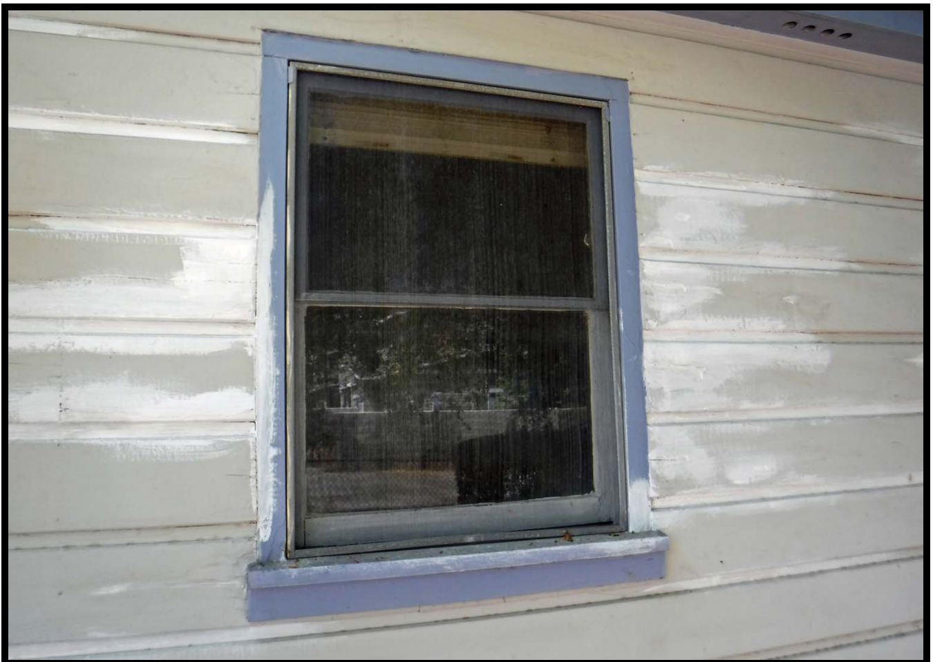
Window Detail, North Elevation, 610 W. Walnut Avenue, Monrovia, CA (SW)
