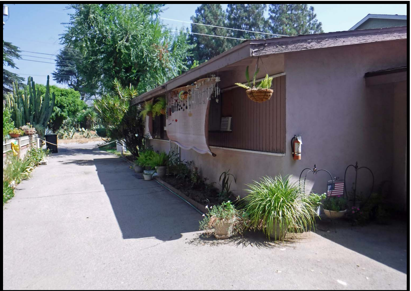
Residential Unit at 634 W. Olive Avenue, Monrovia, CA (NNE)
