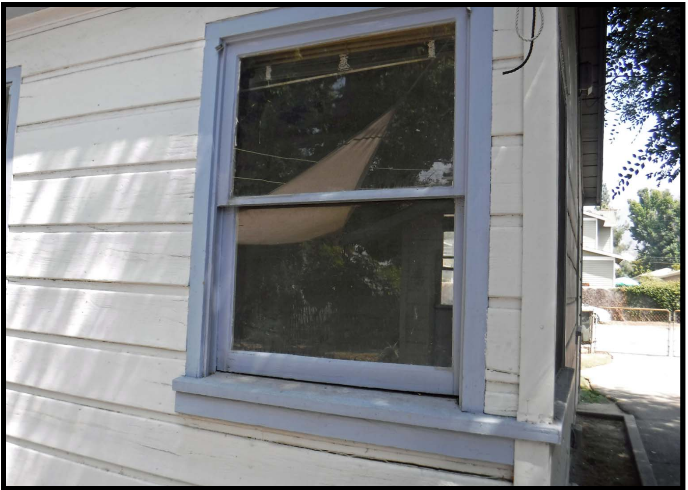
Window Detail, South Elevation, 610 W. Walnut Avenue, Monrovia, CA (NW)
