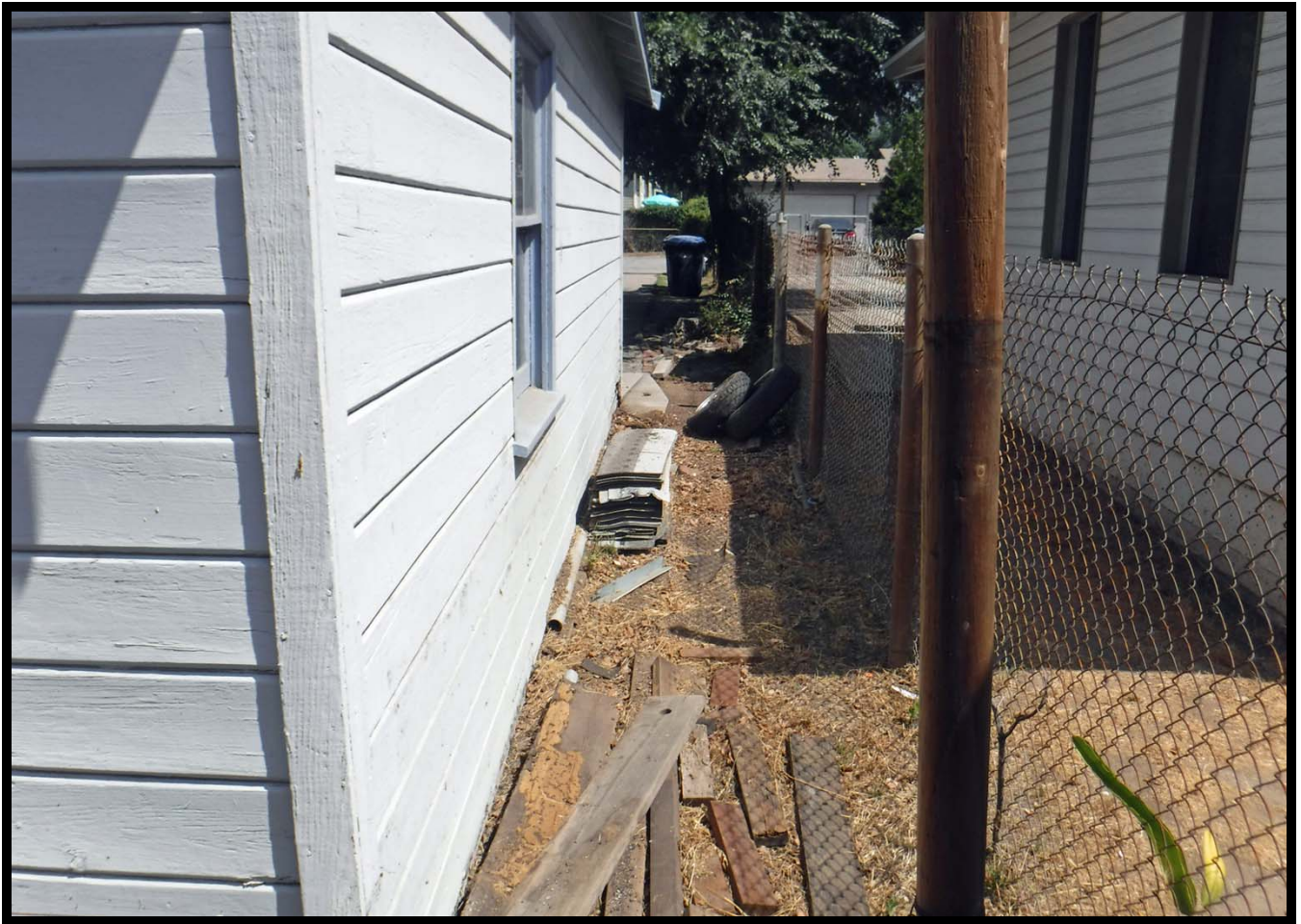
East Elevation of Garage (and Property Line), 610 W. Walnut Avenue, Monrovia, CA (N)
