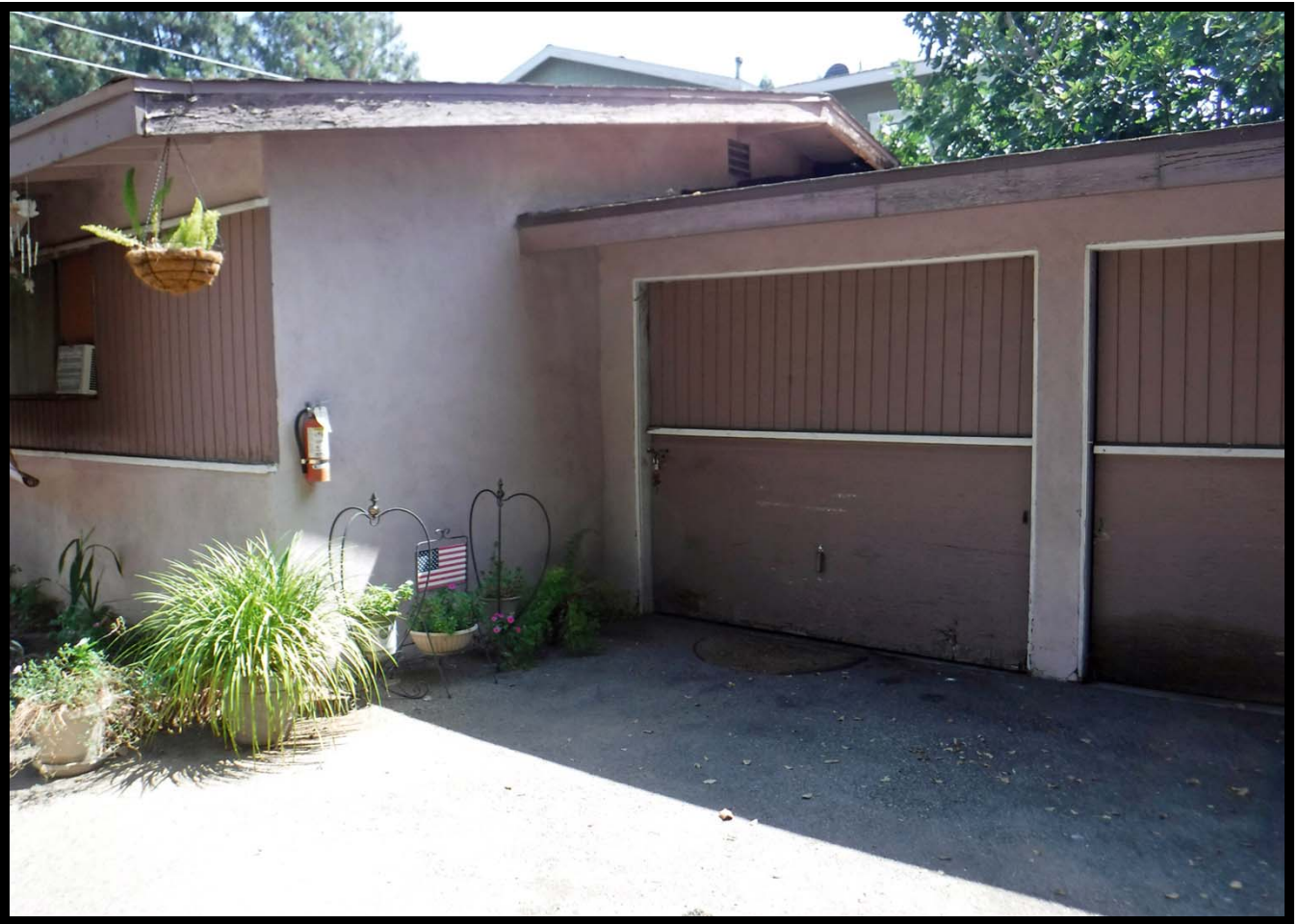
Garage at 634 W. Olive Avenue, Monrovia, CA (ENE)
