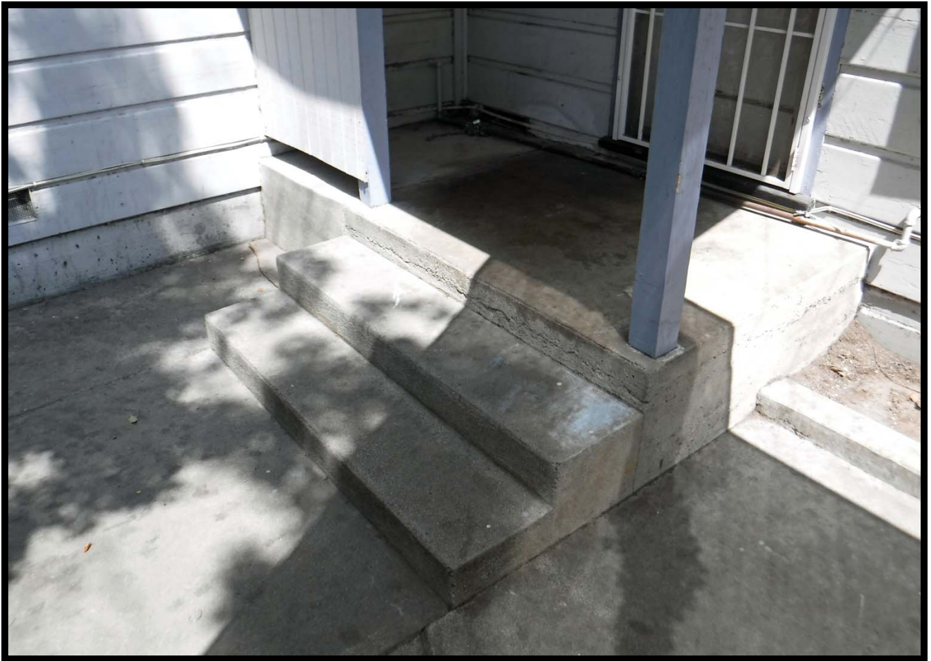
Rear Stoop, South elevation, 610 W. Walnut Avenue, Monrovia, CA (NW)
