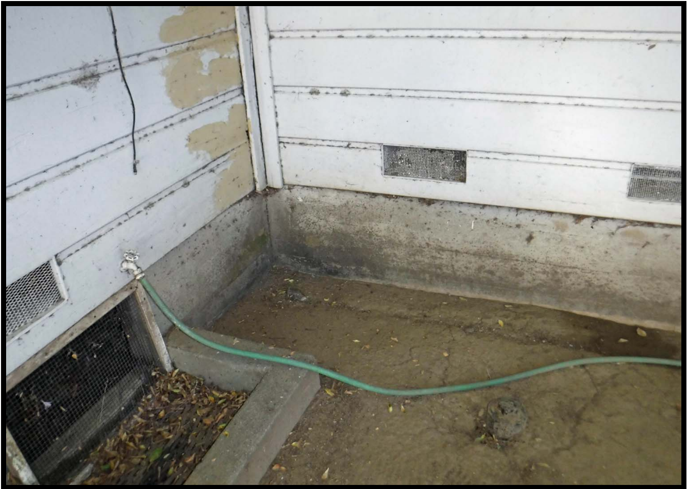
Foundation on West Elevation, 610 W. Walnut Avenue, Monrovia, CA (SE)
