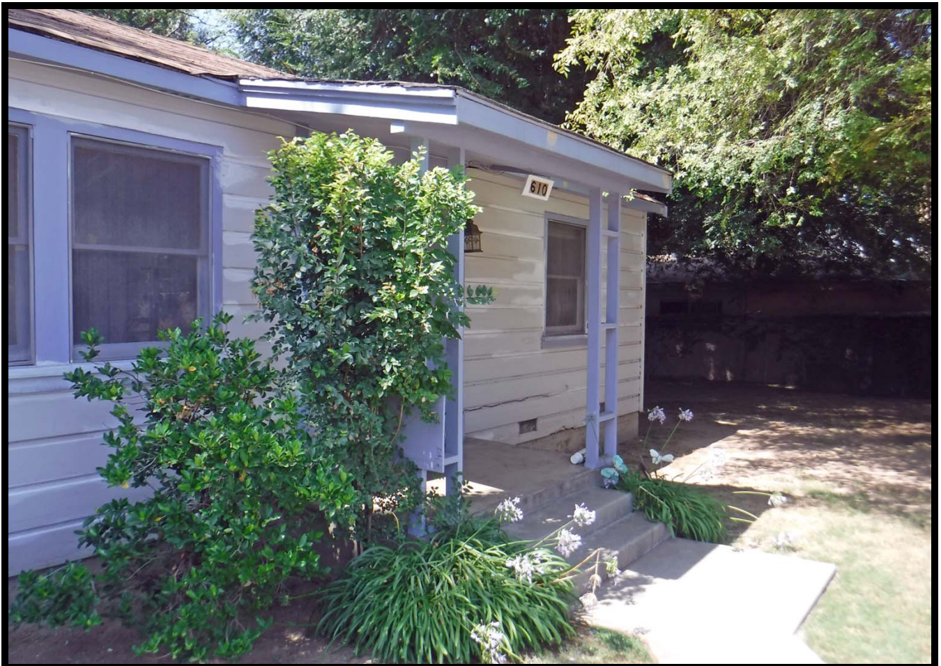
North Elevation, 610 W. Walnut Avenue, Monrovia, CA (WSW)
