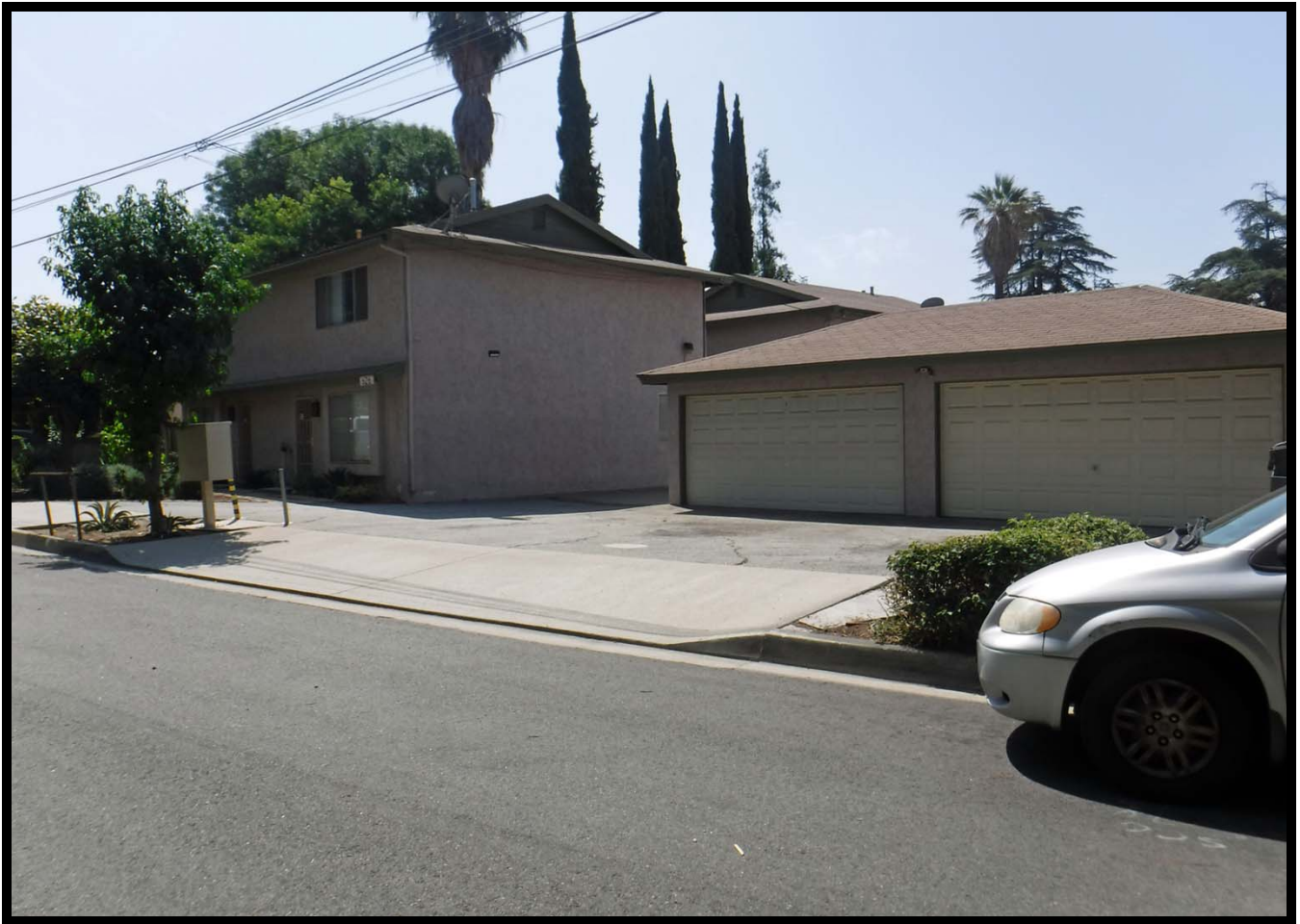
Residential Complex at 626 W. Olive Avenue, Monrovia, CA (1977; SE)
