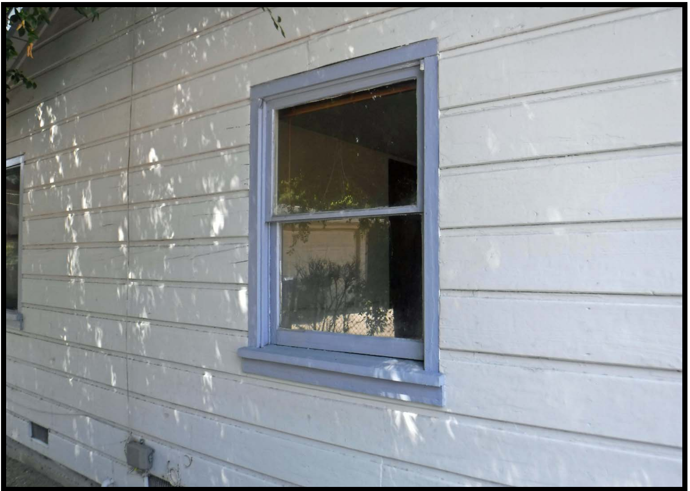
Window Detail, East Elevation, 610 W. Walnut Avenue, Monrovia, CA (SW)
