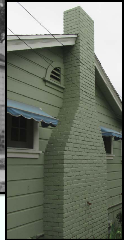
Restore Brick Chimney
