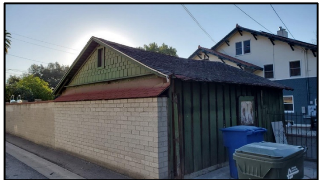
Figure 3. View of existing garage (North and East Elevation).
