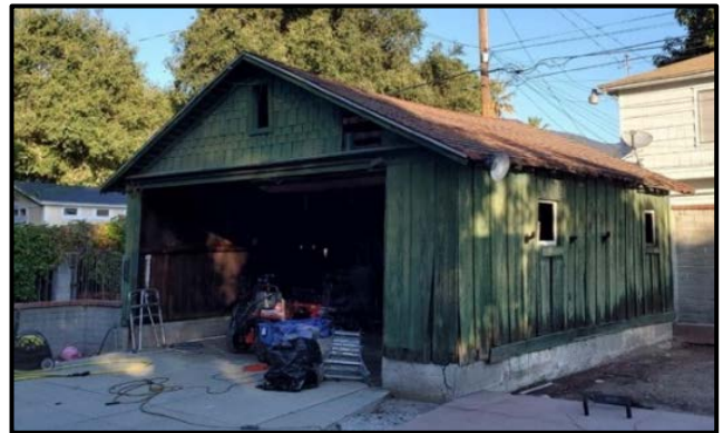
Figure 2. View of the south and east elevations of the existing garage.
