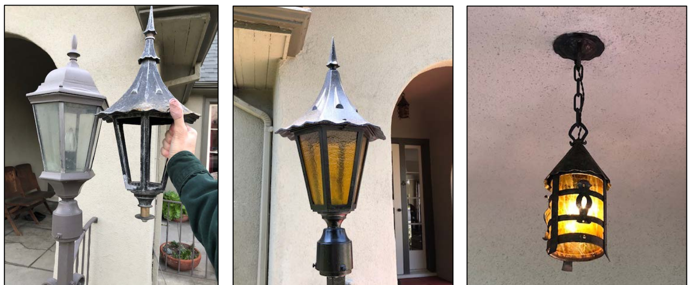
Figure 2. The owners installed antique light fixtures. The photo to the left shows the comparison between the previous 1960's era light and the "period appropriate" light. The center photo shows the light fixture restored with amber glass. Notice that the middle portion of the spire was removed to reduce the overall height; the original height made it appear out of proportion to the lamp posts. The photo to the right is a matching porch light.
