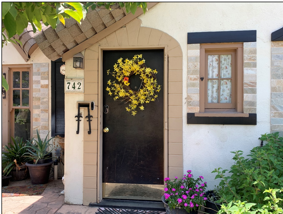
Front (North) elevation view of front entrance sheltered within the front-gabled roof.
