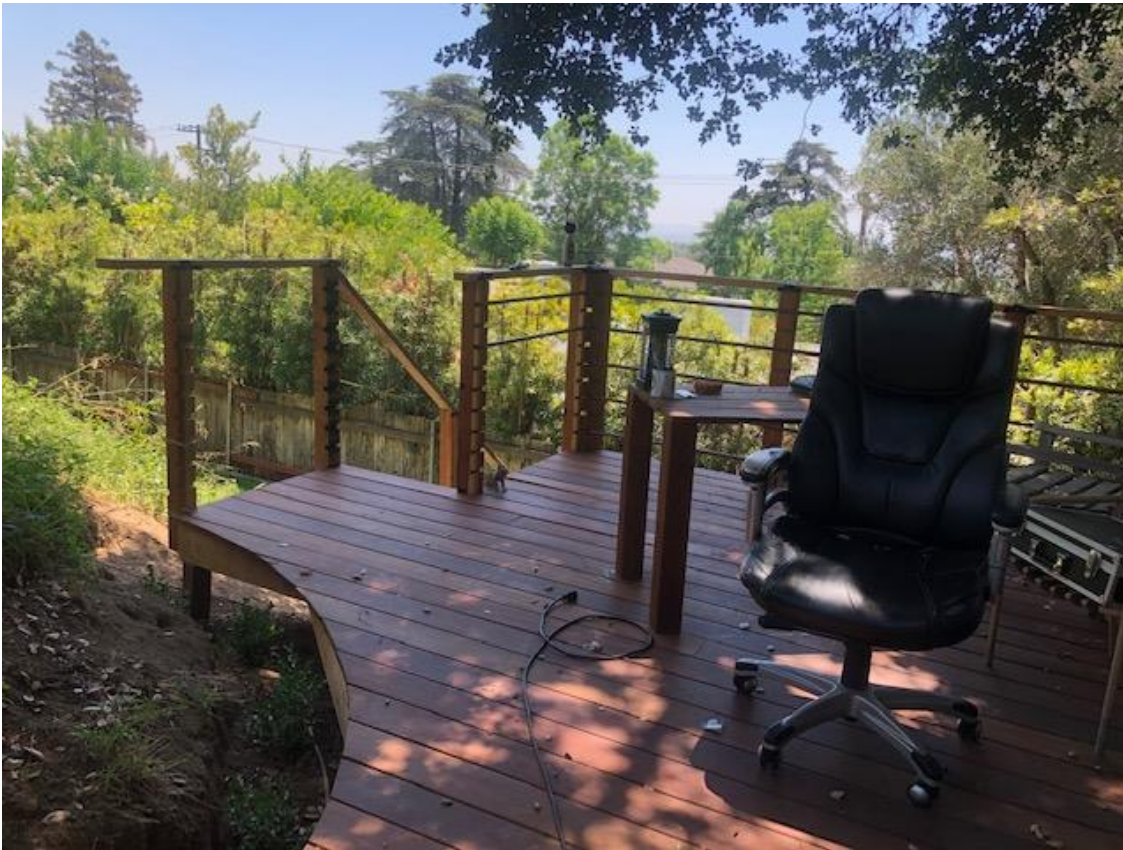
This is the stairway to the bottom of my property that starting this deck/treehouse.
