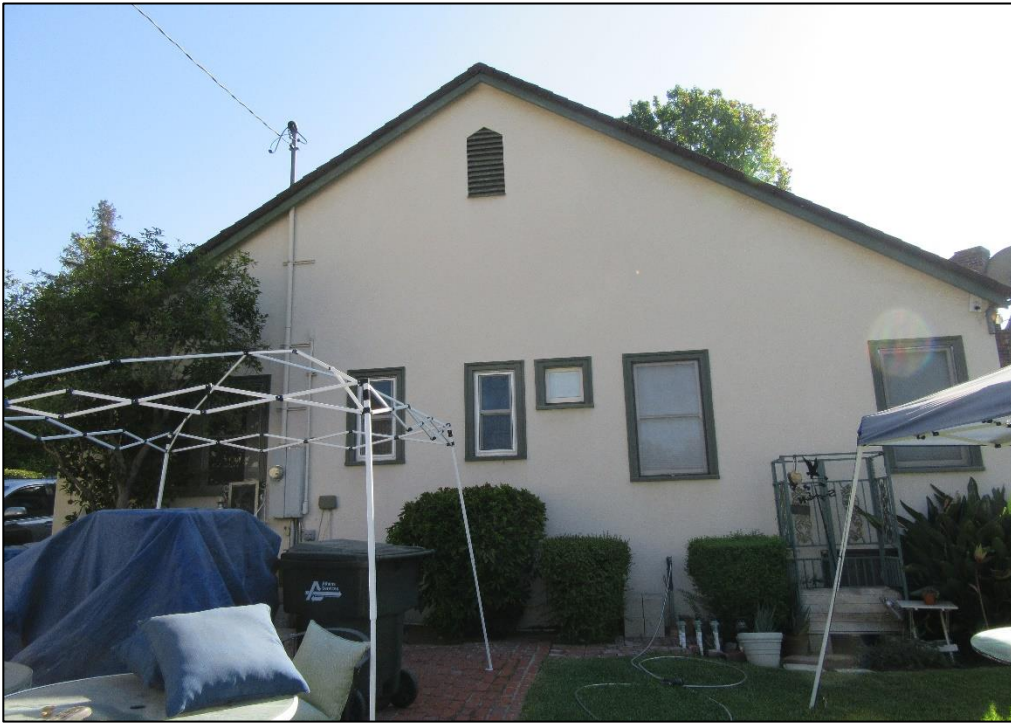
View of west (rear) side of the house.
