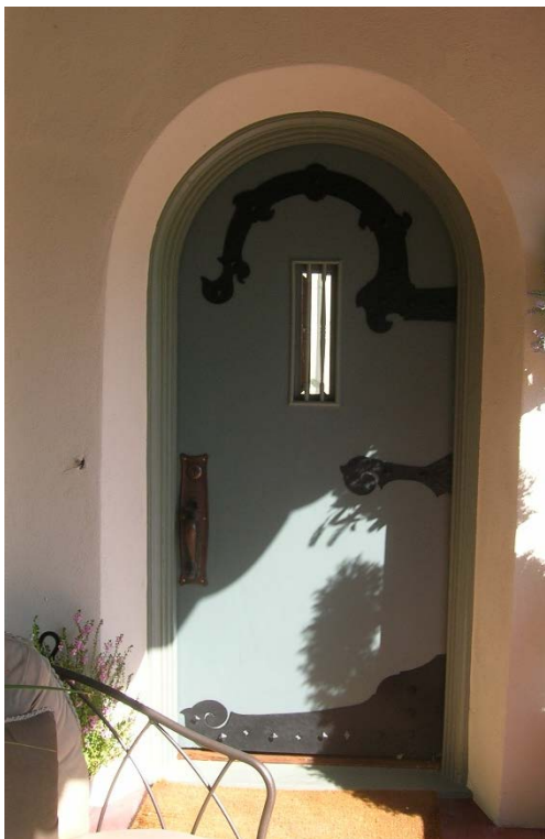
View of original front entrance door.
