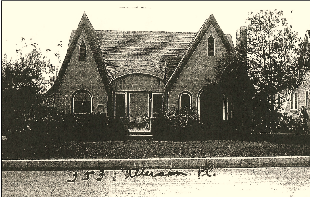
Figure 2. Street view of the English Tudor Revival style house as it appeared in 1933.
