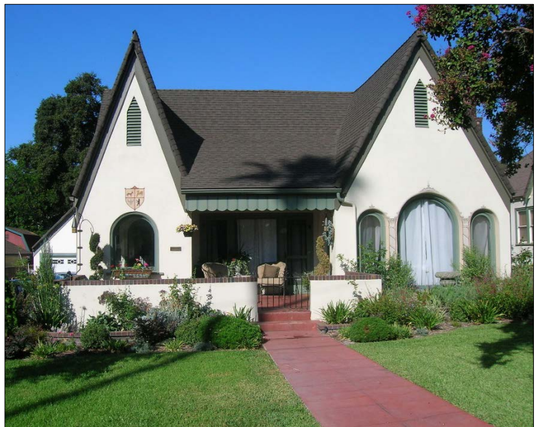
Figure 1. Street view of the English Tudor Revival style house located at 353 Patterson Drive. The building was built in 1927.
