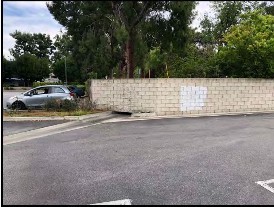
View along the southern property boundary, facing east.
