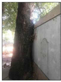
As you can see the tree has already done damage to the block wall which will have to be repaired. The leaning block wall and angle of trunk also show how this is more of a park/ city tree and should be saved.
