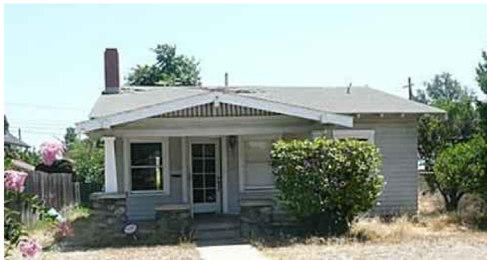
EXISTING FRONT UNIT
