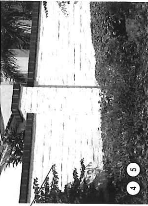
4 Slump brick wall with sack finish and painted white to match existing building.
