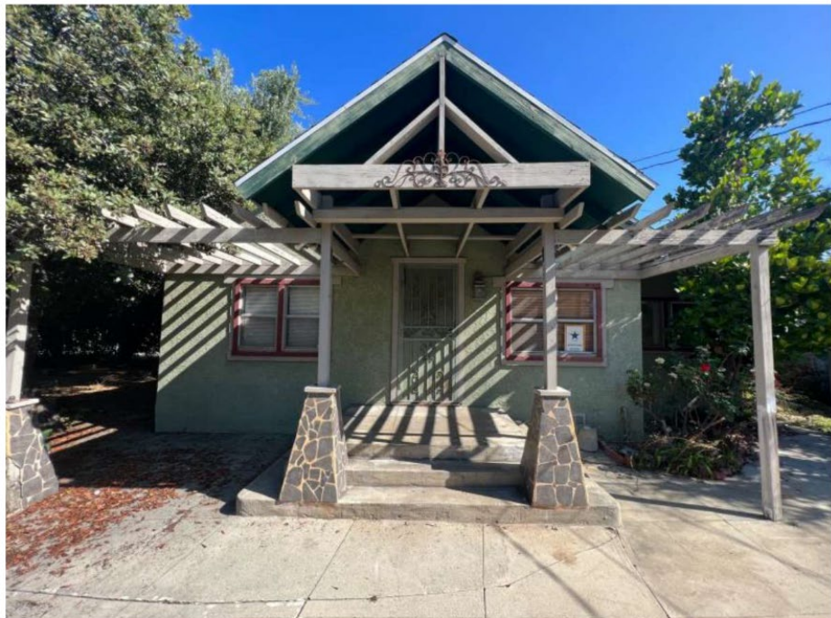
Figure 11. Primary/Southern Façade, 619½ E Walnut Avenue SOURCE: Sapphos Environmental, Inc., 2023
