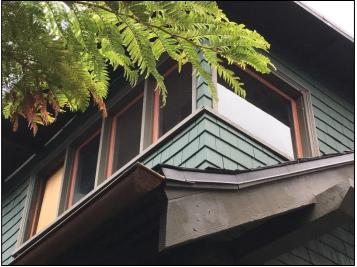
The photograph to the right shows the five sunroom windows where dual glazing is proposed. As shown in the photo, one of these window is currently boarded up with plywood.
