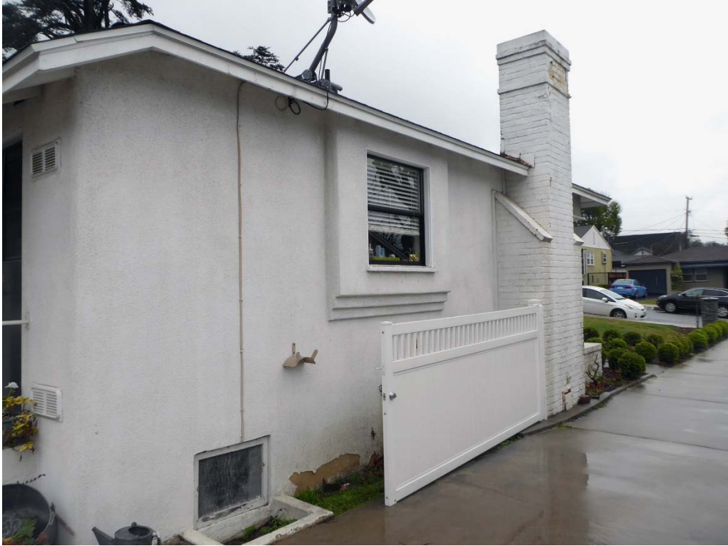
Figure 8. View of the south façade looking northeast.
