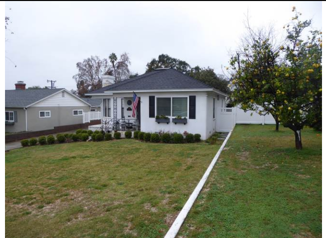
Image 4. View of the northeast oblique looking southwest.
