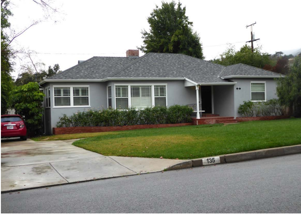
Figure 20. View of 135 N. Madison Avenue.
