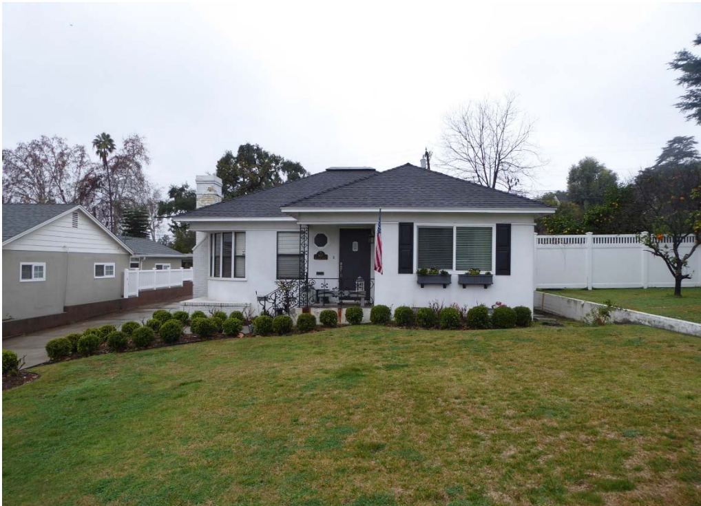
Figure 4. View looking west at the east façade of the house.
