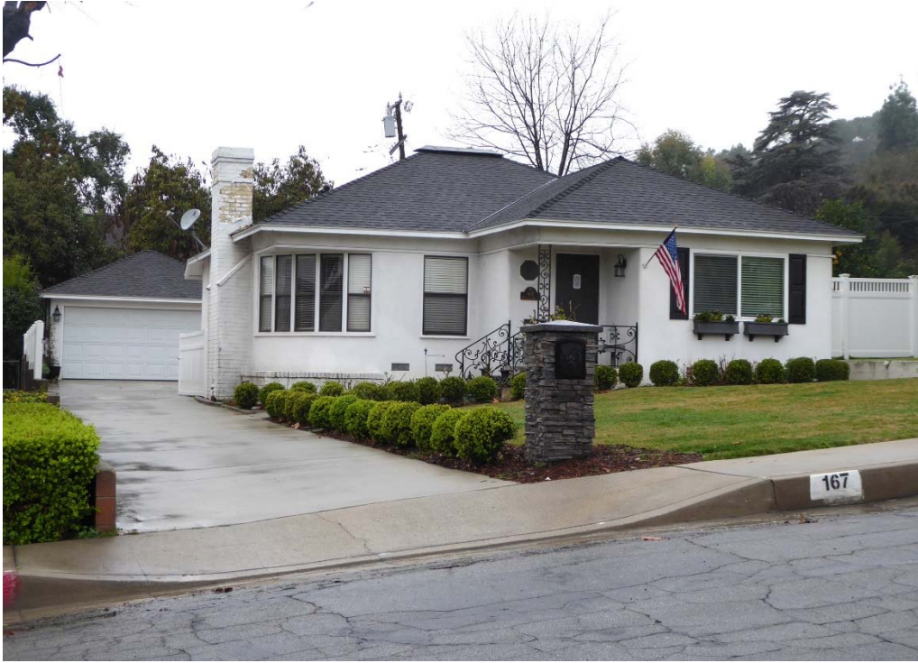
Figure 3. Overview of 167 N. Lincoln Place looking northwest.
