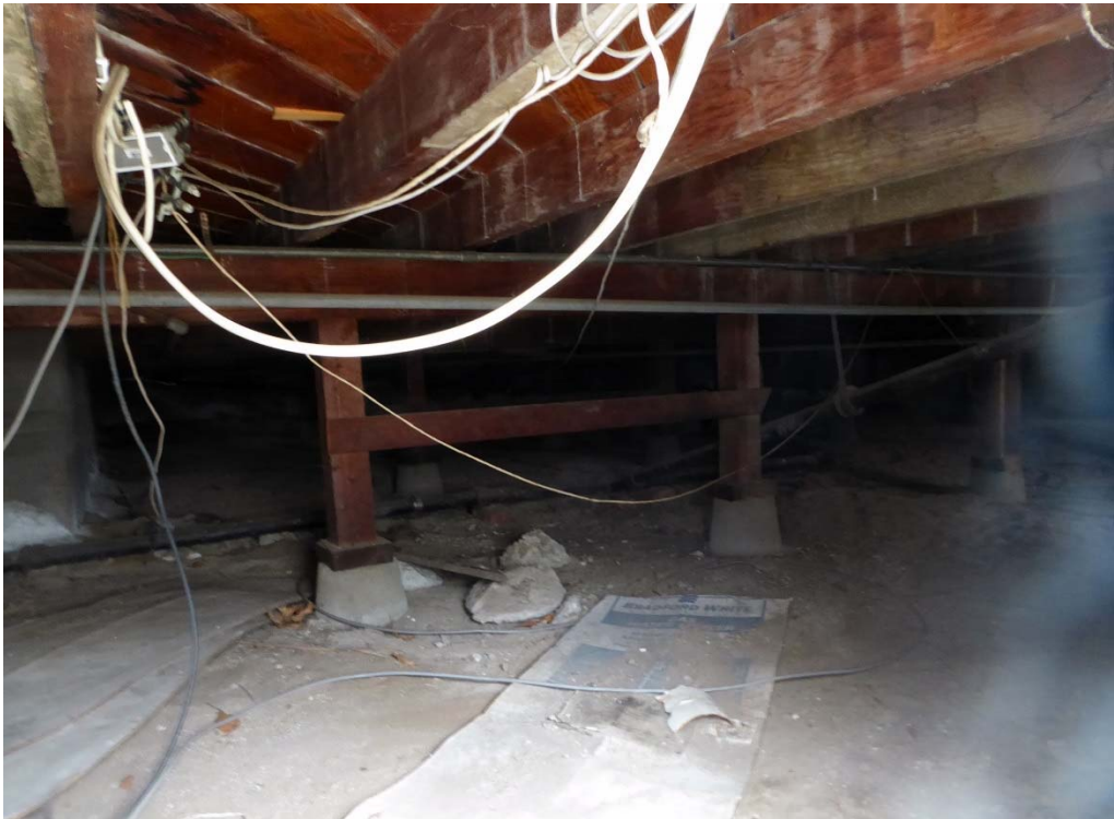
Figure 13. View of the crawlspace.
