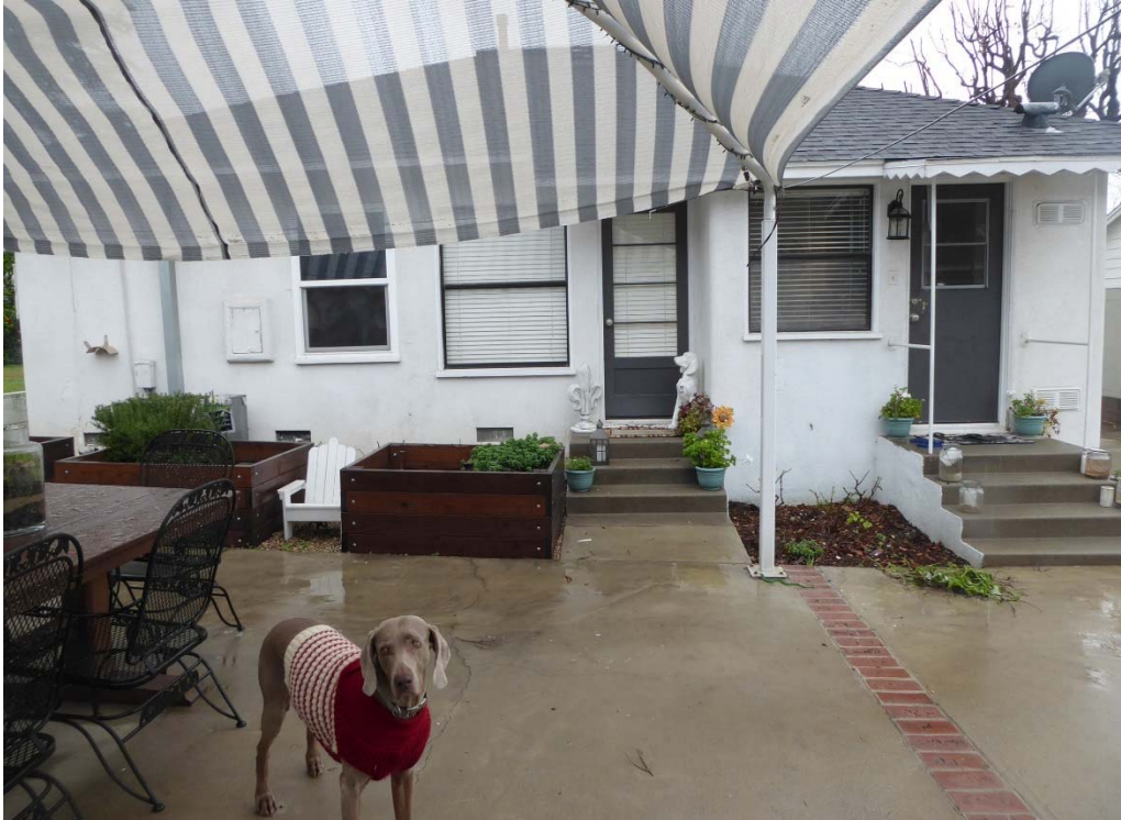
Figure 10. View of the west façade of the house looking east.
